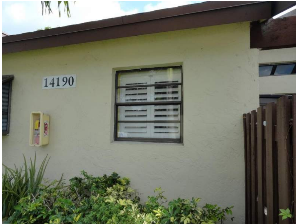
7. Opening Protection – Unrated Unprotected Windows
