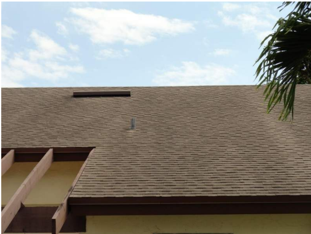
2. Roof Covering – Asphalt Shingles
