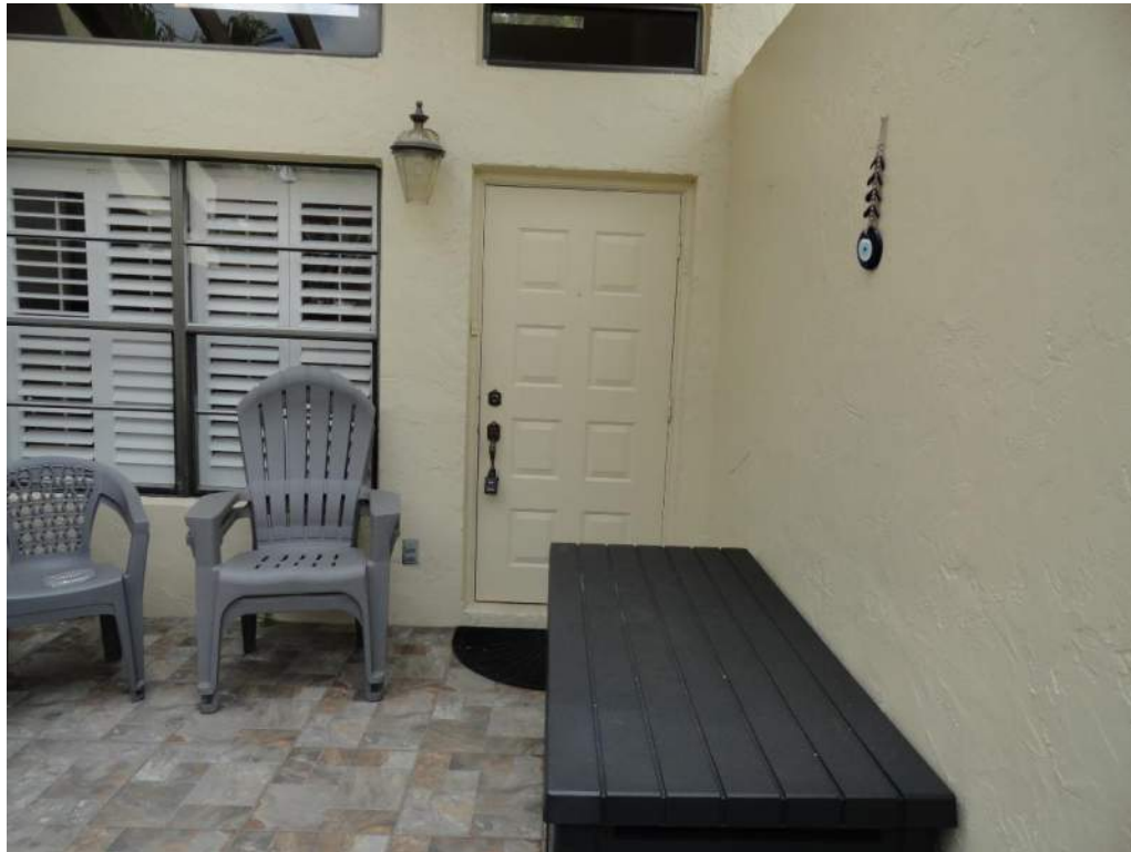
7. Opening Protection – Unprotected Unrated Unglazed Entry Door
