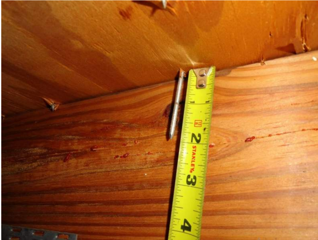
3. Roof Deck Attachment – 8d Nails
