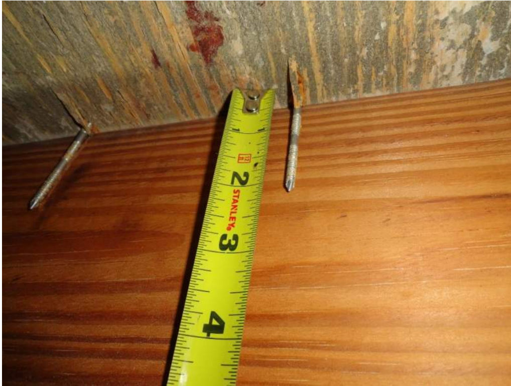
3. Roof Deck Attachment – 8d Nails
