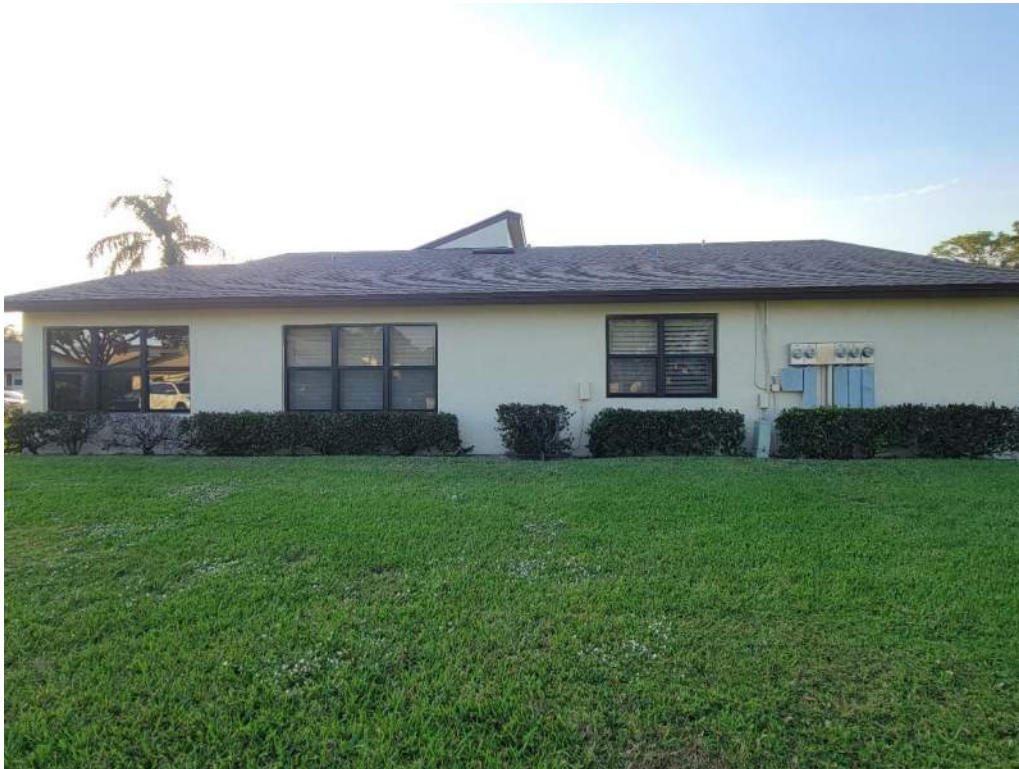
5. Roof Geometry – Right Elevation – Non-Hip
