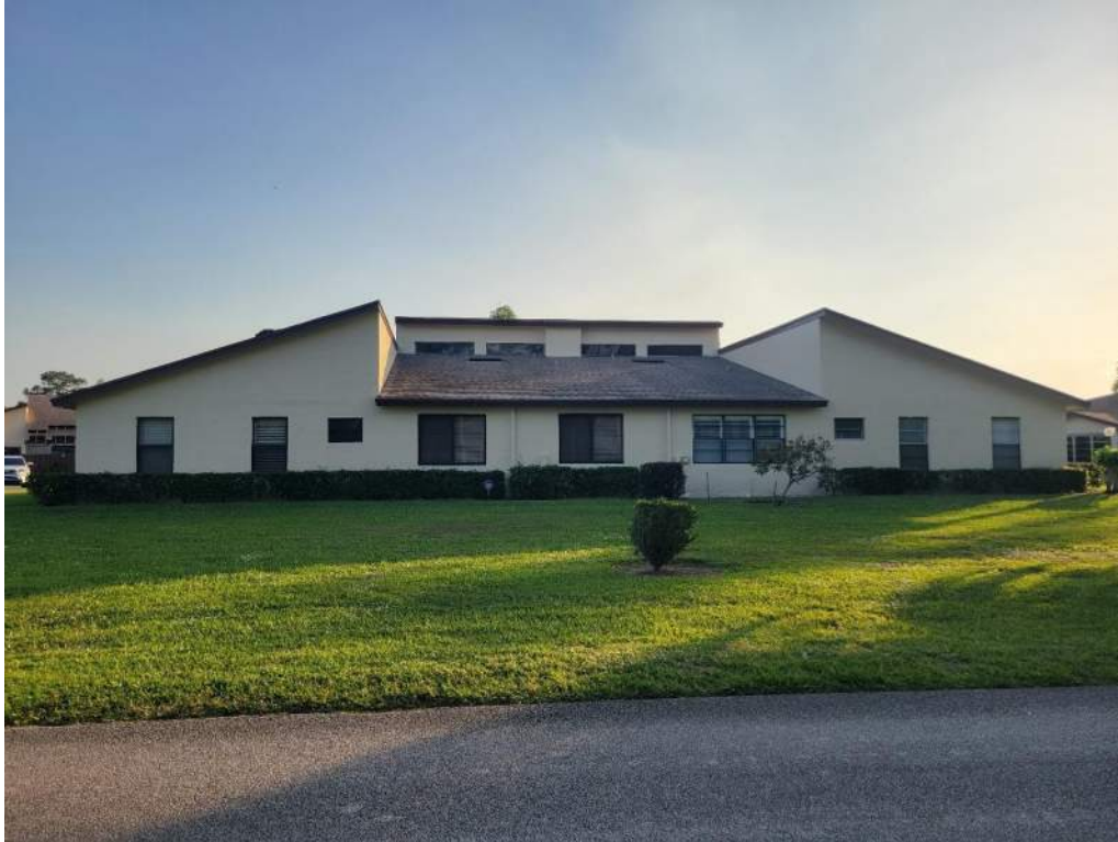
5. Roof Geometry – Rear Elevation – Non-Hip
