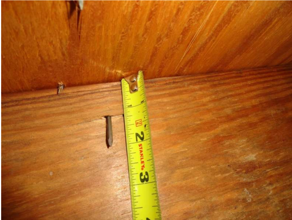
3. Roof Deck Attachment – 8d Nails
