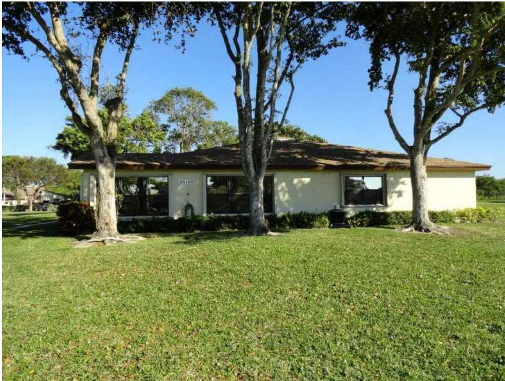
5. Roof Geometry – Right Elevation – Hip
