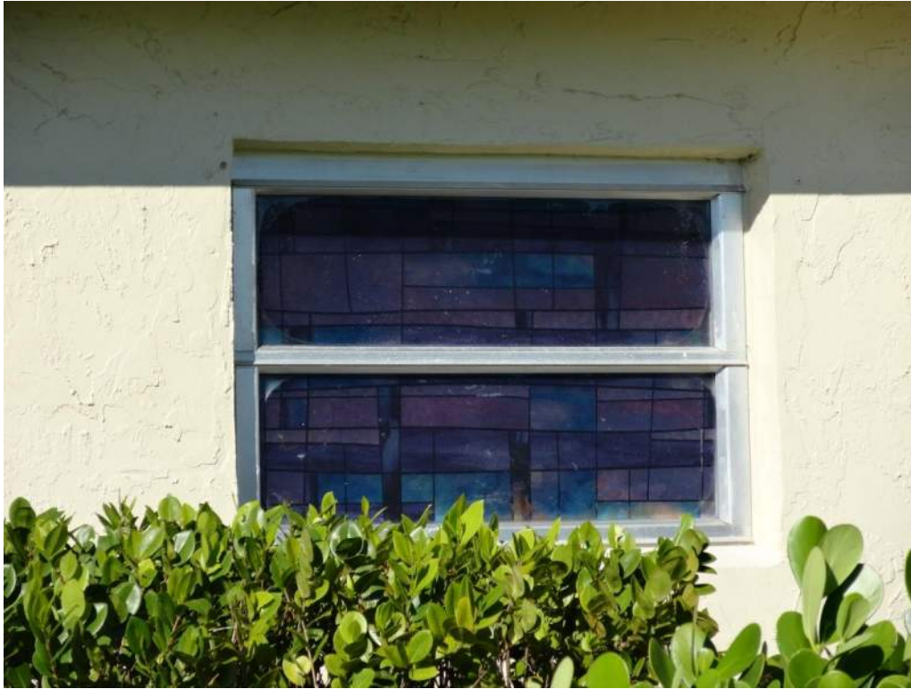
7. Opening Protection – Unrated Unprotected Windows
