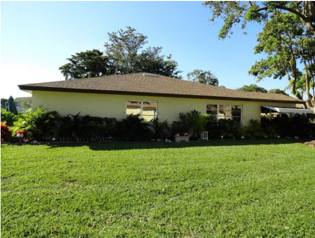
5. Roof Geometry – Left Elevation – Hip
