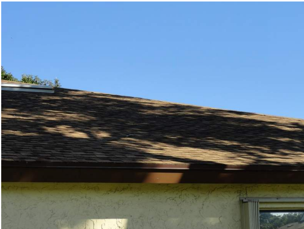
2. Roof Covering – Asphalt Shingles
