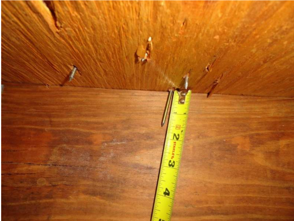
3. Roof Deck Attachment – 8d Nails
