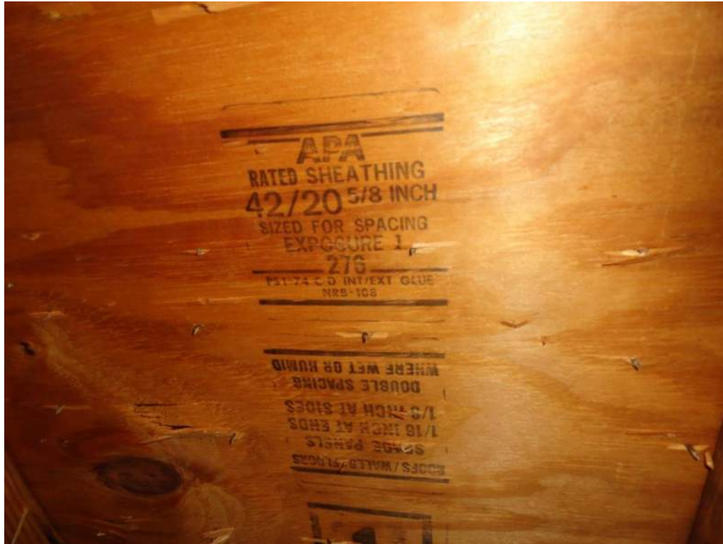
3. Roof Deck Attachment – 5/8" Plywood
