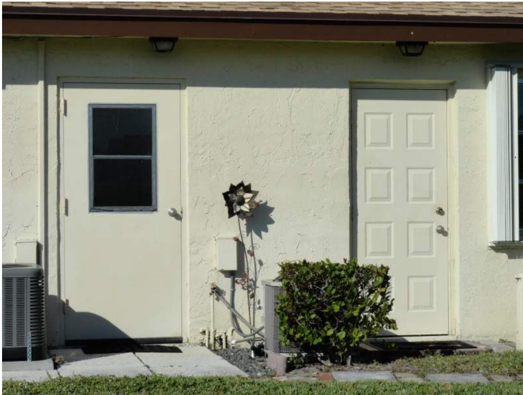
7. Opening Protection – Unprotected Unrated Unglazed Entry Door
