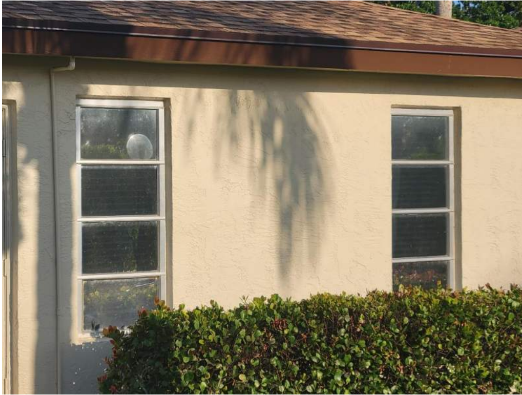
7. Opening Protection – Unrated Unprotected Windows
