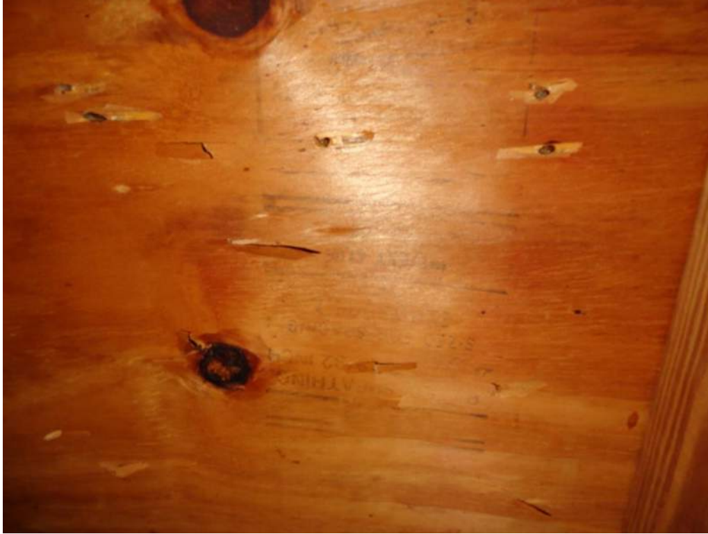
3. Roof Deck Attachment – 19/32" Plywood
