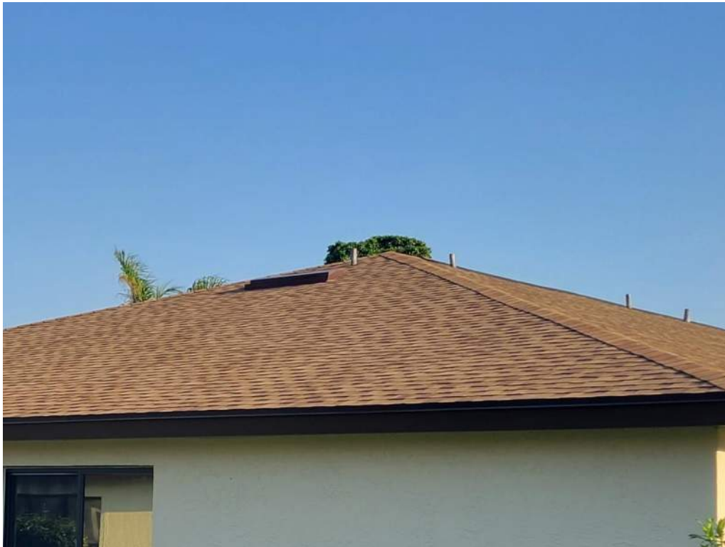
2. Roof Covering – Asphalt Shingles
