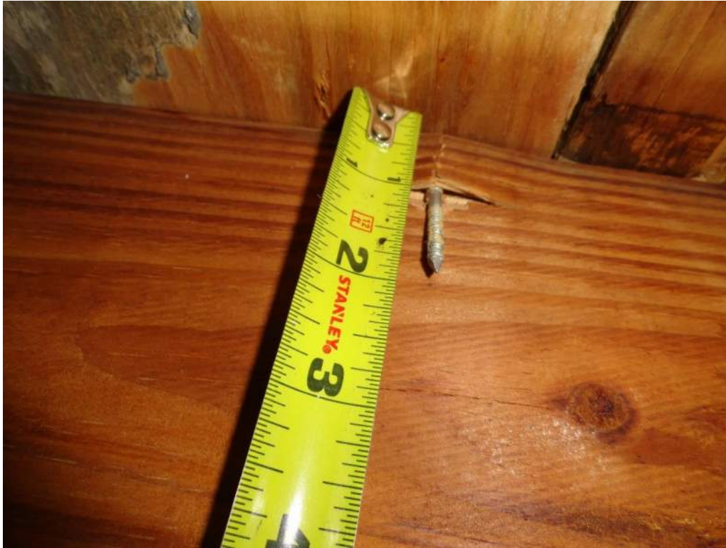
3. Roof Deck Attachment – 8d Nails
