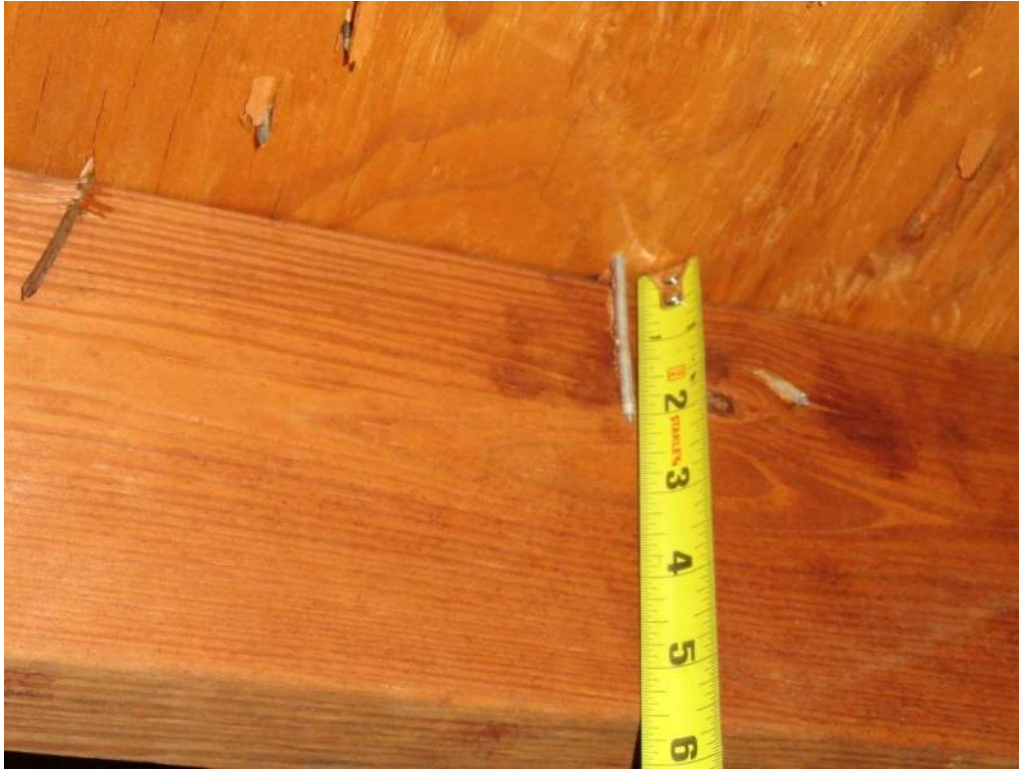
3. Roof Deck Attachment – 8d Nails
