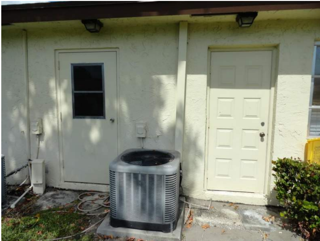
7. Opening Protection – Unprotected Unrated Unglazed Entry Door
