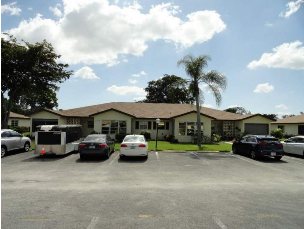
5. Roof Geometry – Front Elevation – Non-Hip
