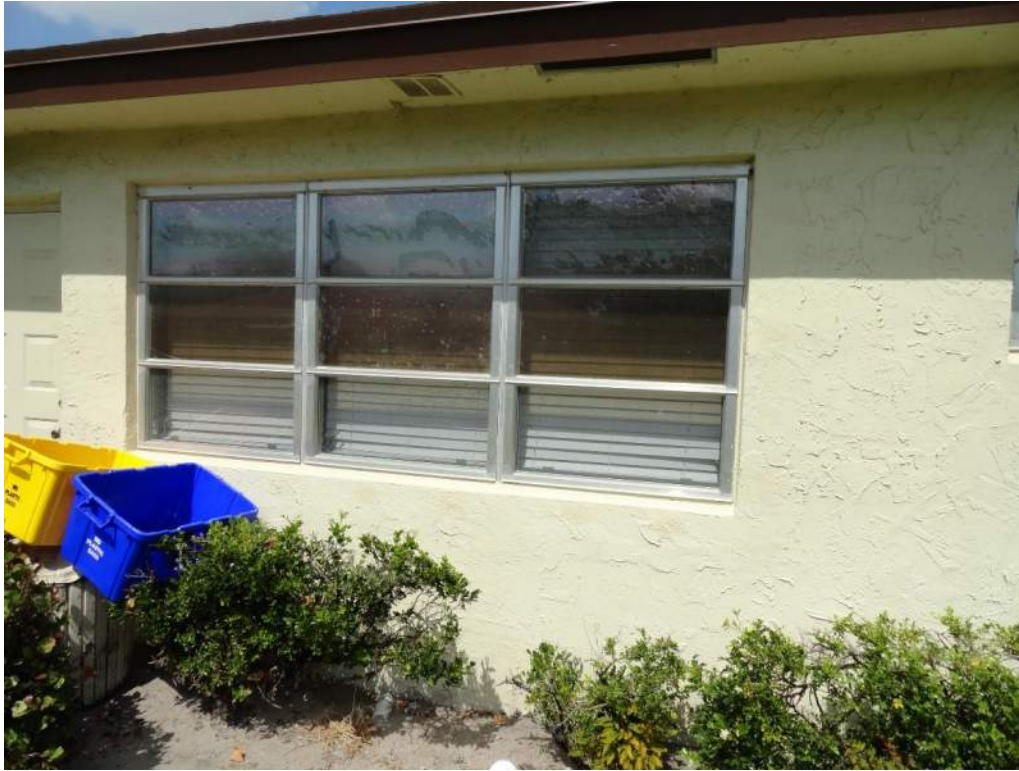
7. Opening Protection – Unrated Unprotected Windows
