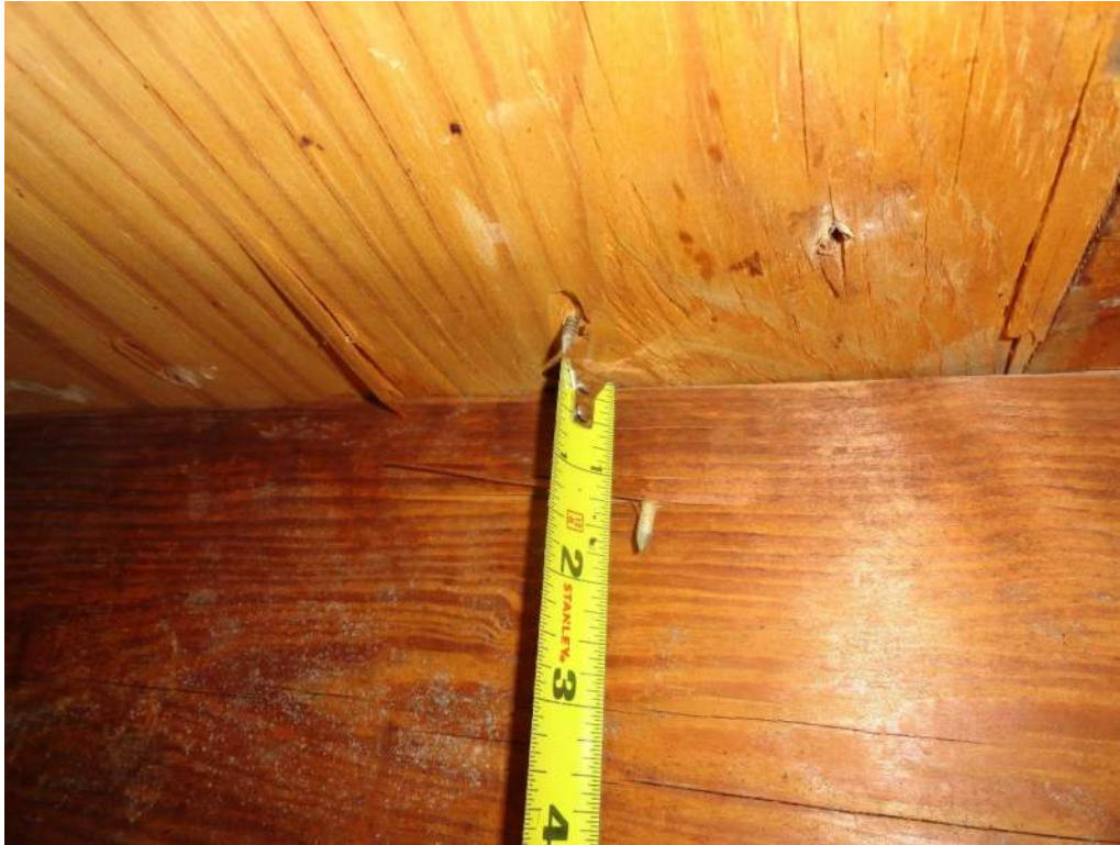
3. Roof Deck Attachment – 8d Nails
