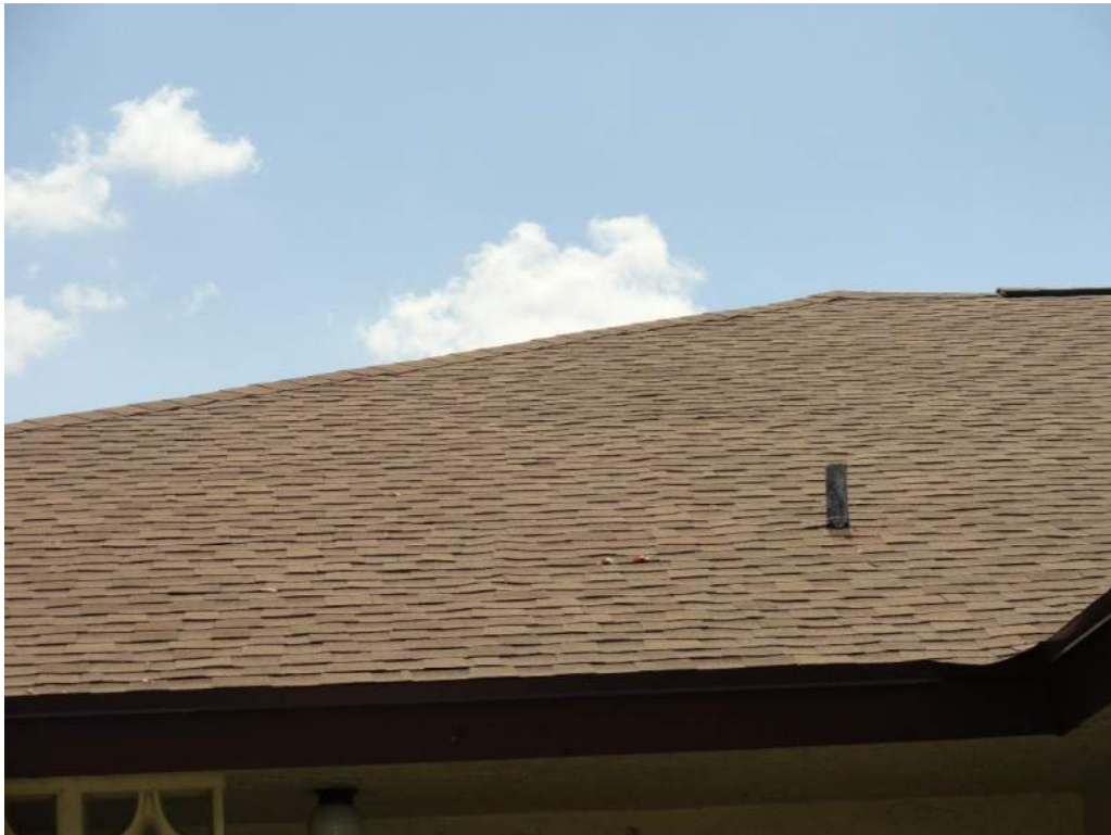
2. Roof Covering – Asphalt Shingles
