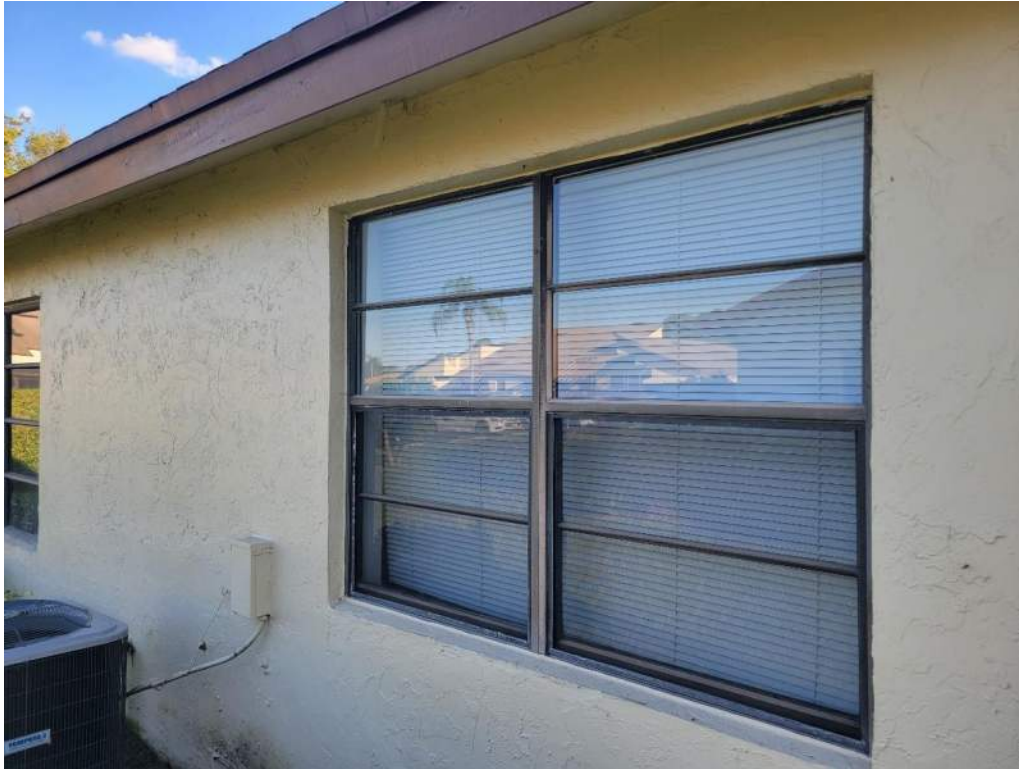
7. Opening Protection – Unprotected Unrated Windows
