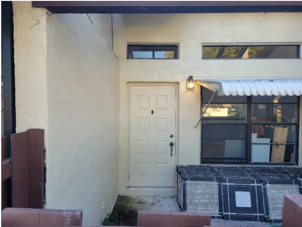
7. Opening Protection – Unprotected Unrated Unglazed Entry Door
