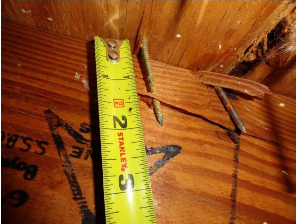
3. Roof Deck Attachment – 8d Nails
