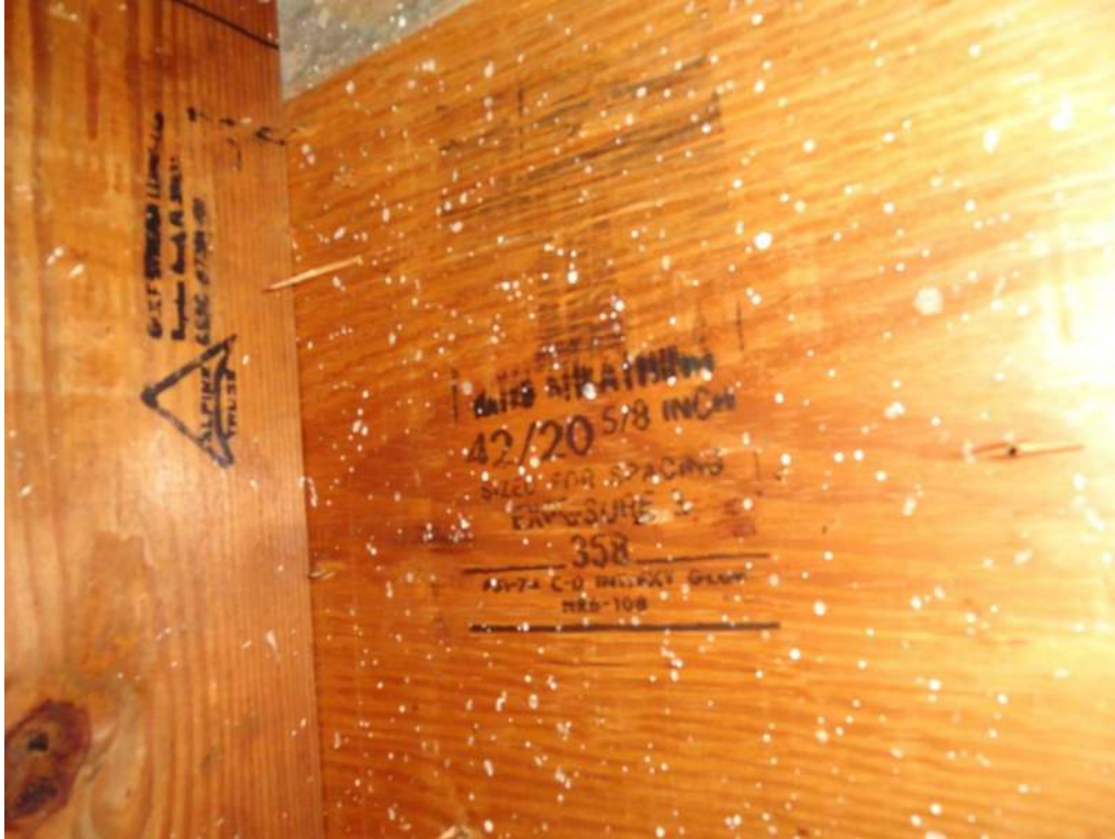
3. Roof Deck Attachment – 5/8" Plywood
