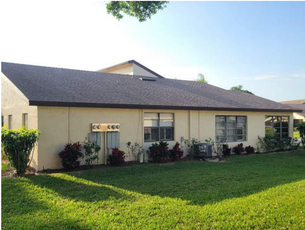
5. Roof Geometry – Left Elevation – Non-Hip
