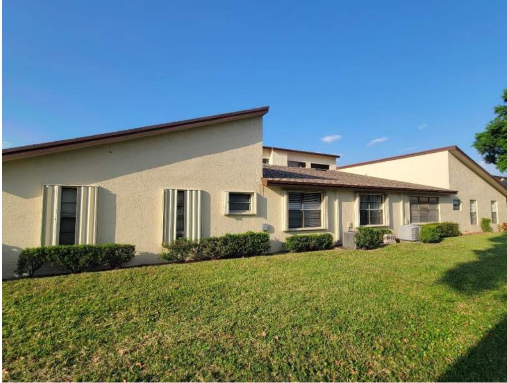
5. Roof Geometry – Rear Elevation – Non-Hip
