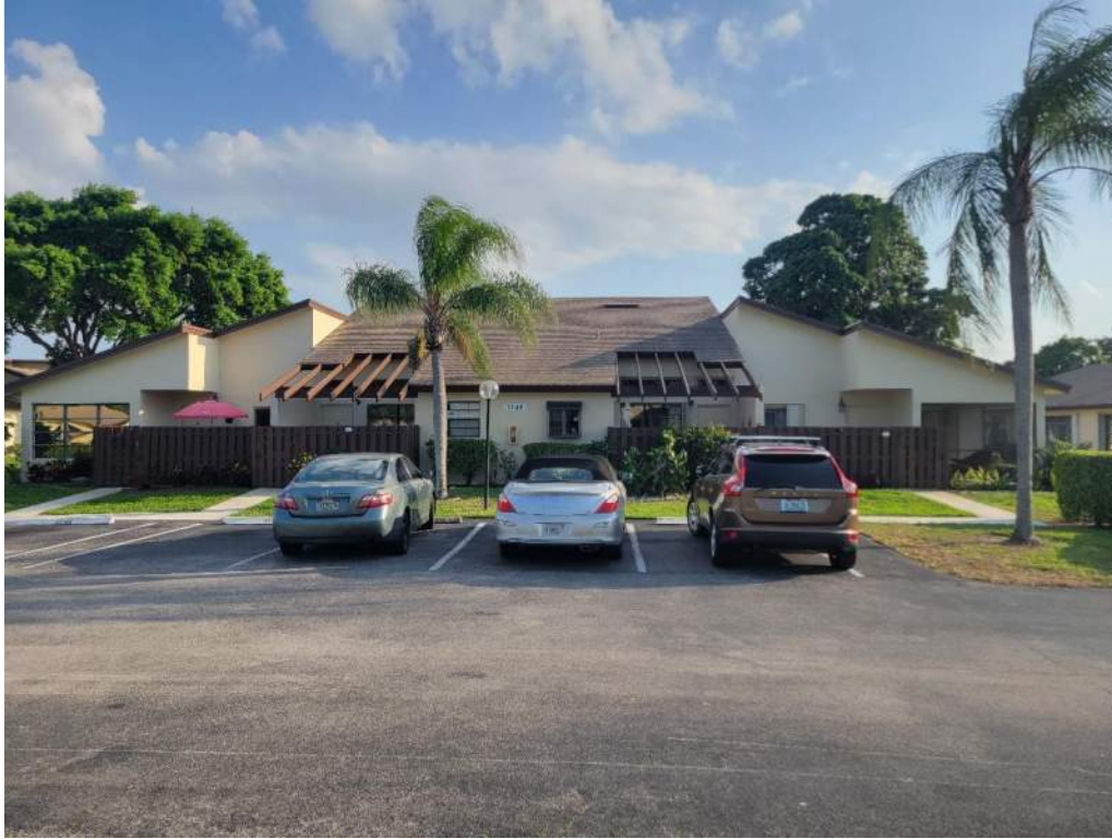
5. Roof Geometry – Front Elevation – Non-Hip
