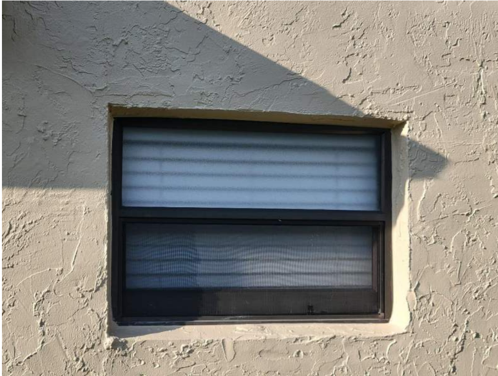
7. Opening Protection – Unrated Unprotected Windows
