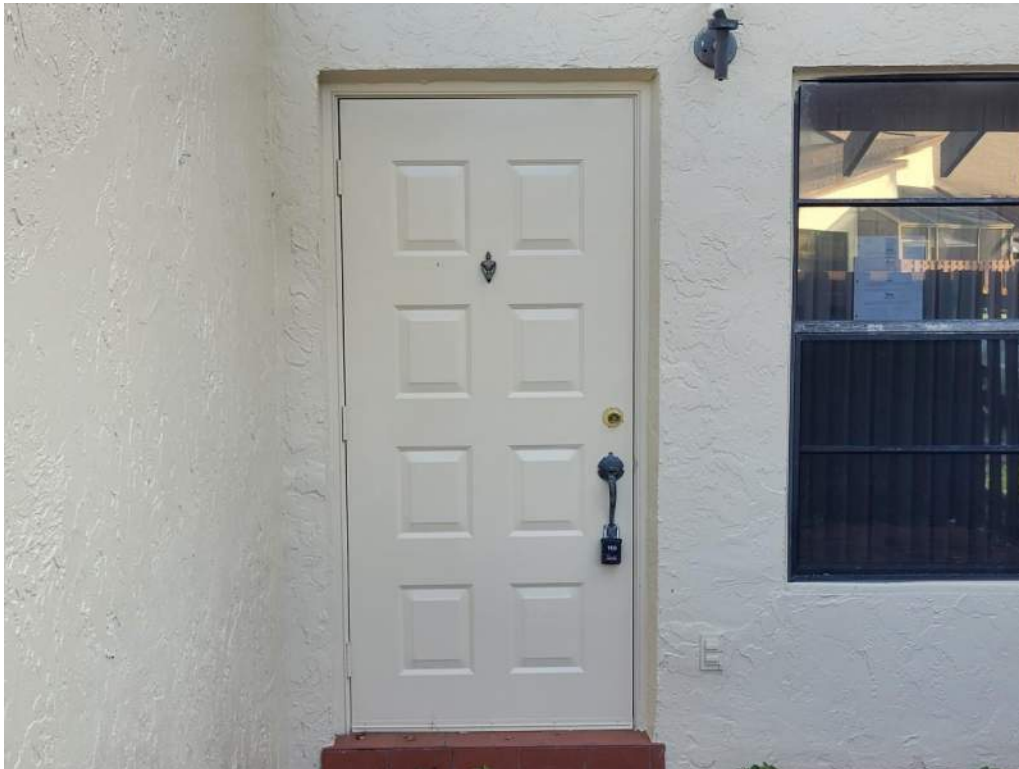
7. Opening Protection – Unprotected Unrated Unglazed Entry Door
