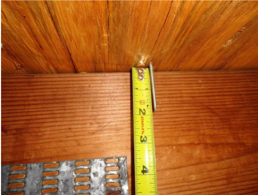
3. Roof Deck Attachment – 8d Nails
