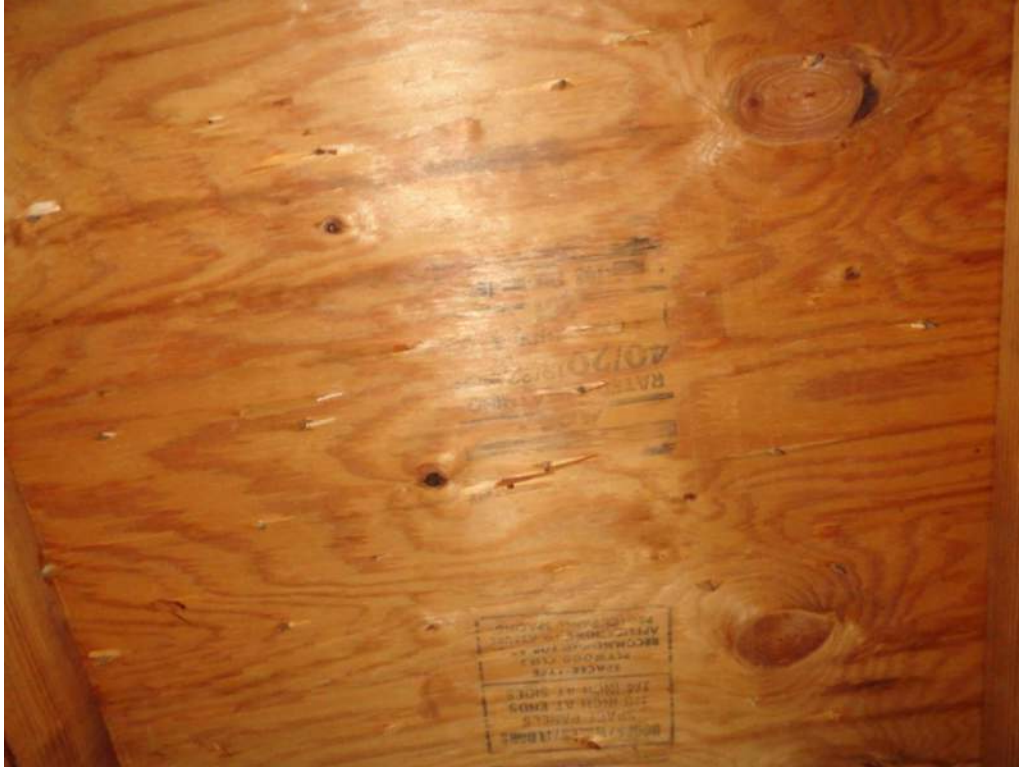
3. Roof Deck Attachment – 19/32" Plywood
