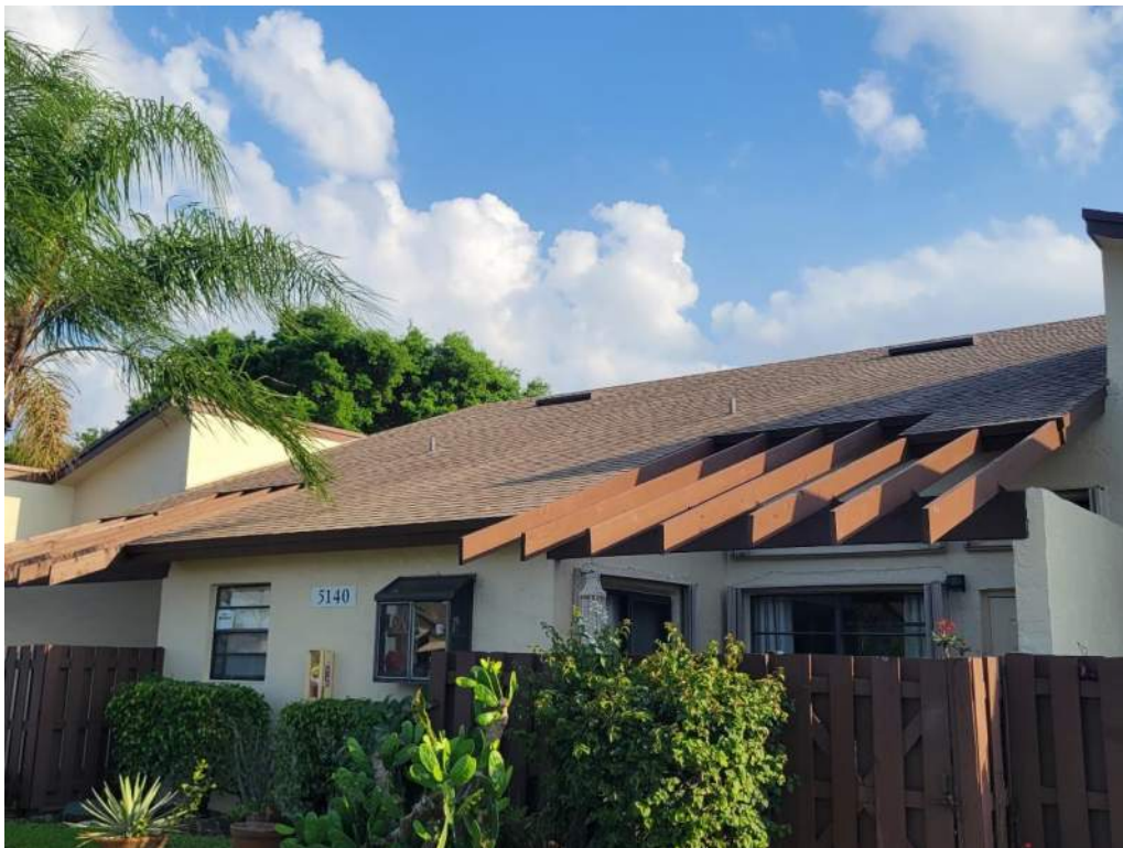
2. Roof Covering – Asphalt Shingles
