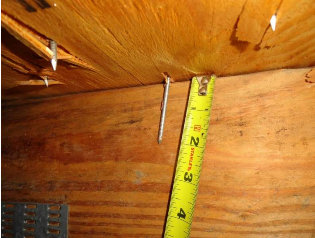
3. Roof Deck Attachment – 8d Nails
