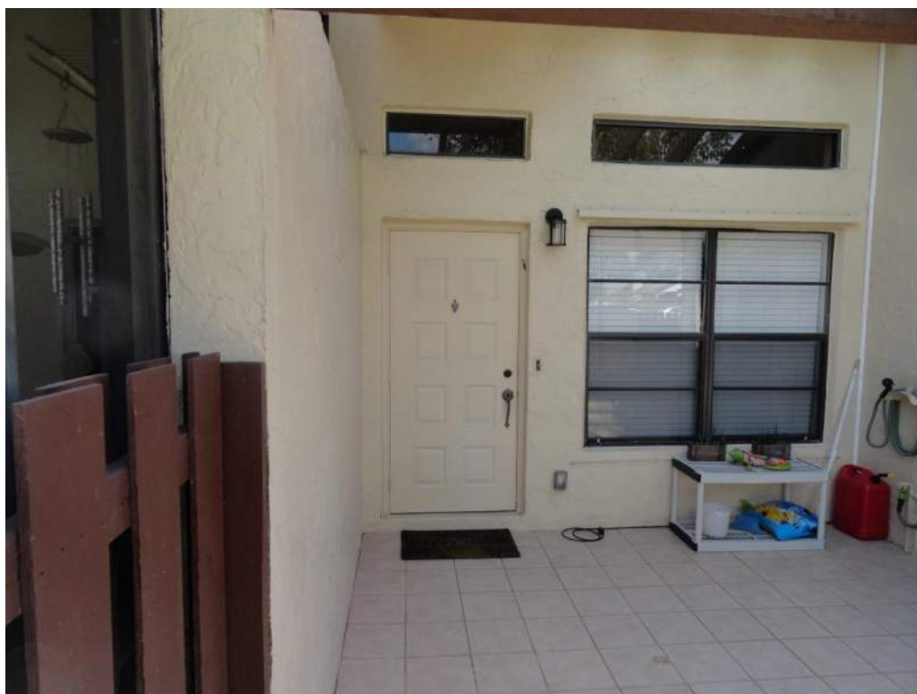
7. Opening Protection – Unprotected Unrated Unglazed Entry Door
