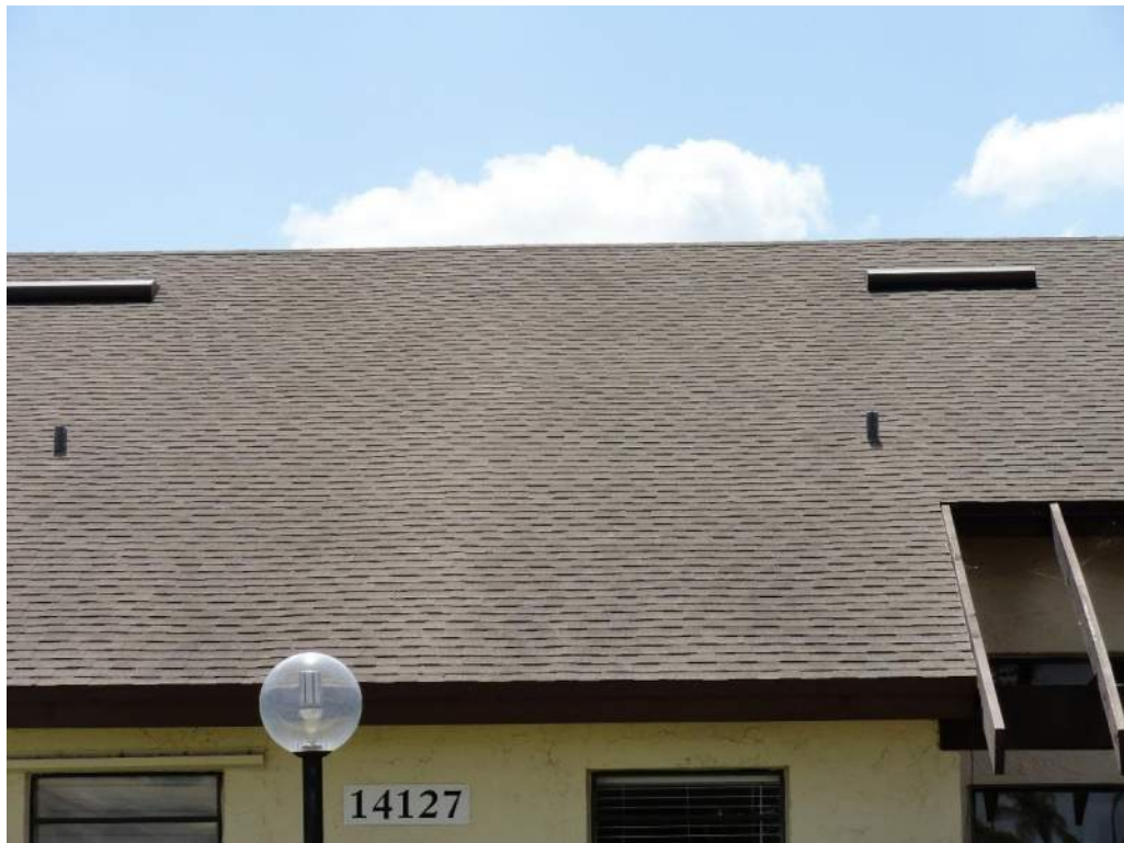
2. Roof Covering – Asphalt Shingles
