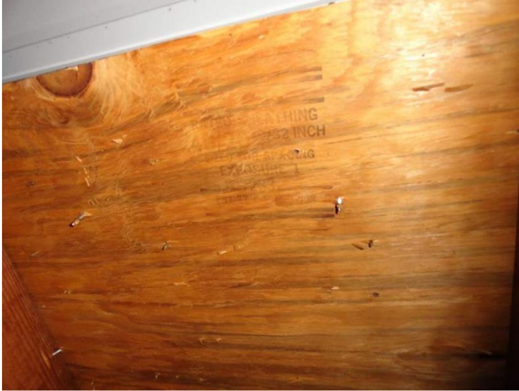
3. Roof Deck Attachment – 19/32" Plywood
