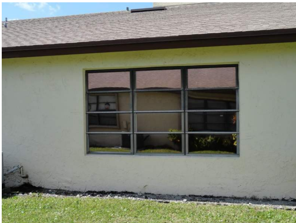
7. Opening Protection – Unprotected Unrated Windows
