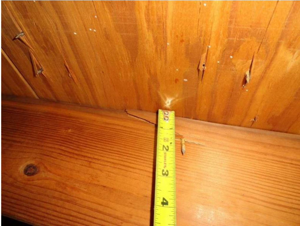
3. Roof Deck Attachment – 8d Nails
