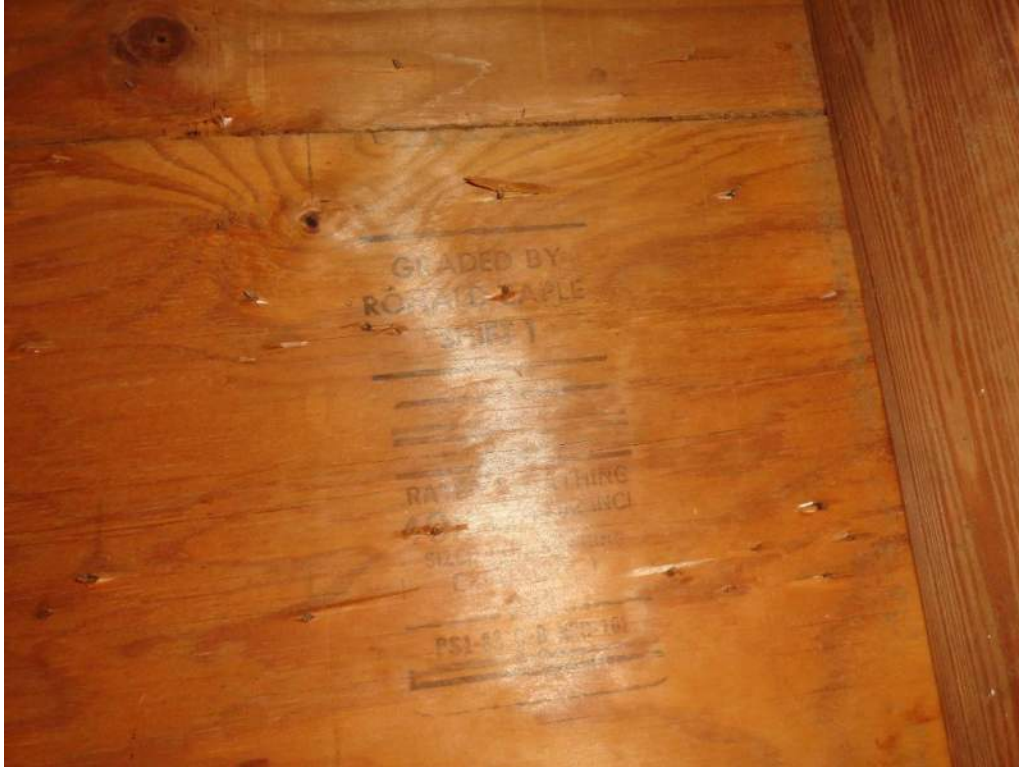
3. Roof Deck Attachment – 19/32" Plywood
