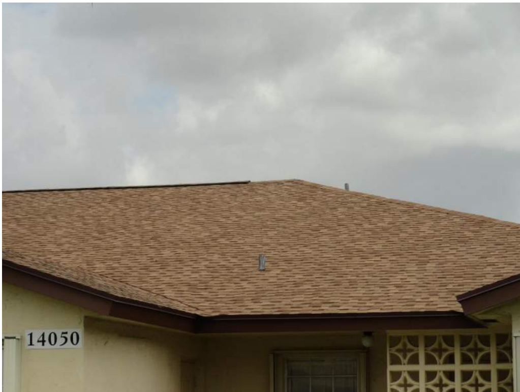
2. Roof Covering – Asphalt Shingles
