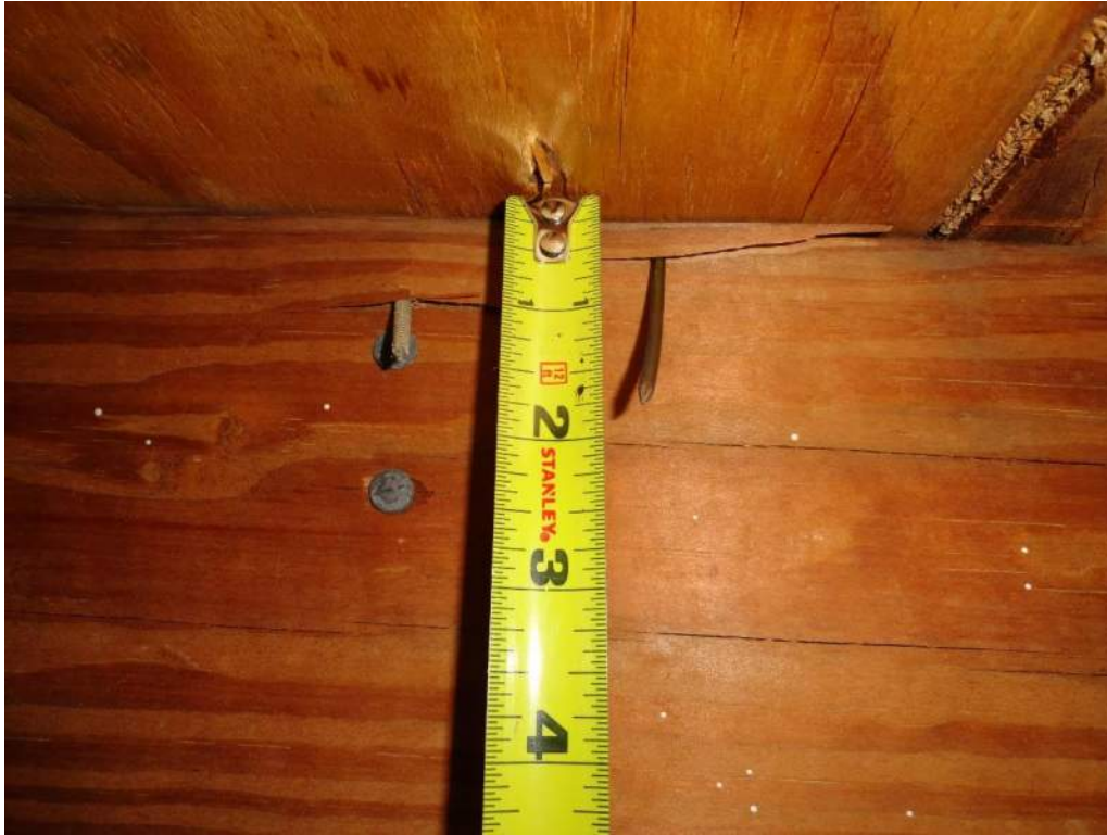
3. Roof Deck Attachment – 8d Nails
