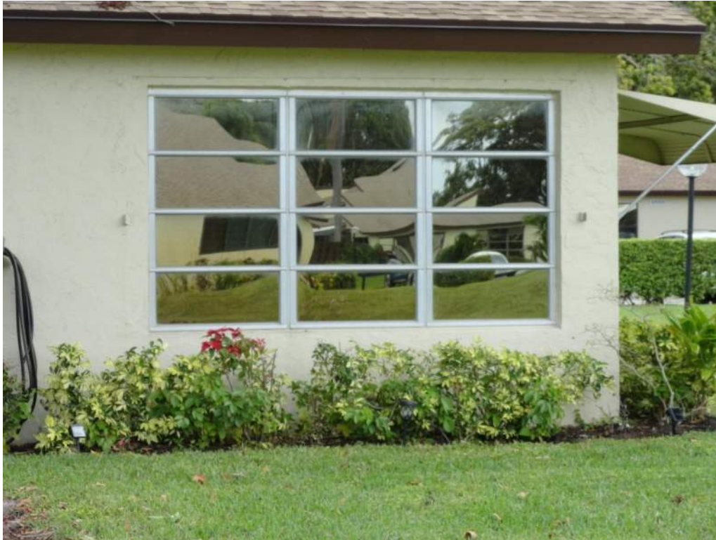
7. Opening Protection – Unrated Unprotected Windows
