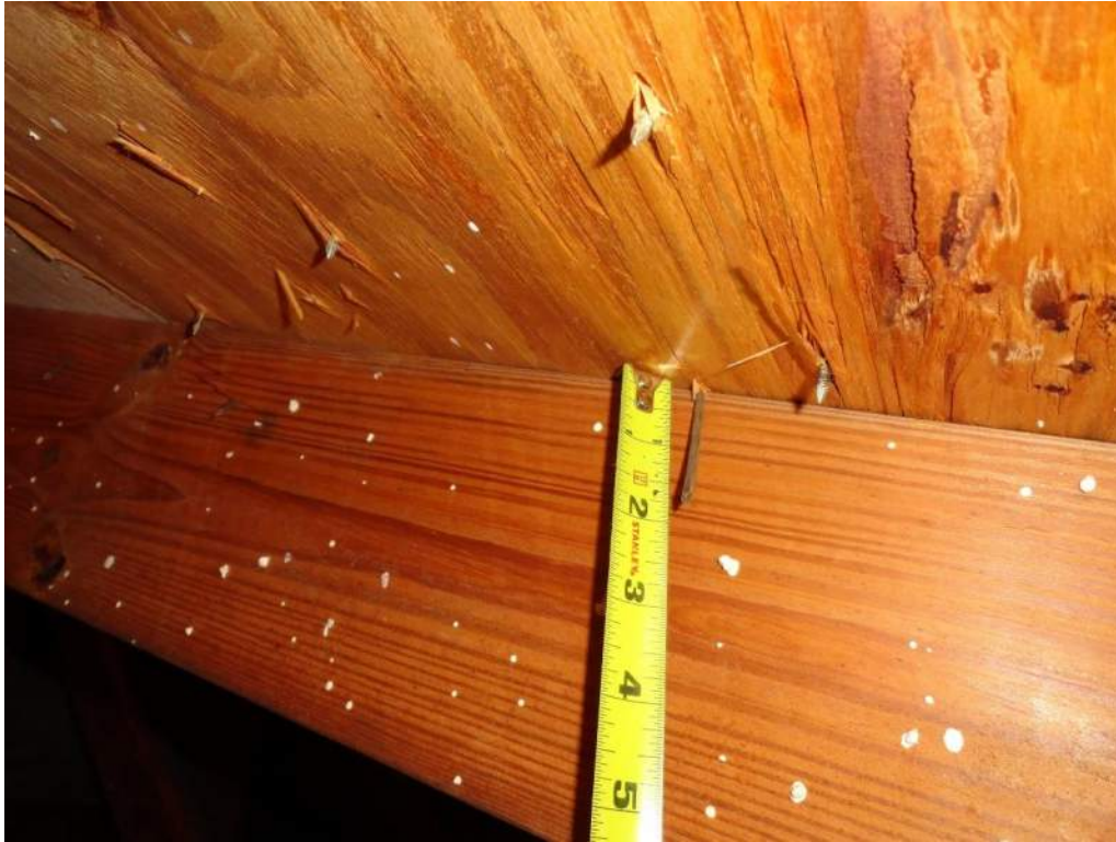
3. Roof Deck Attachment – 8d Nails
