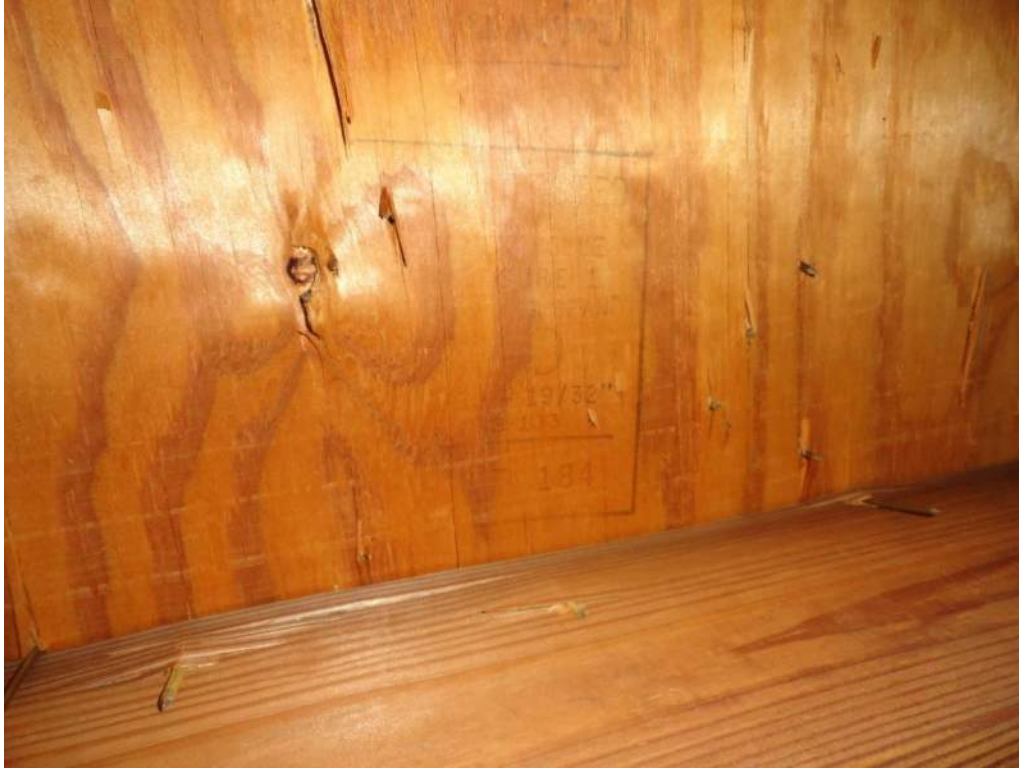
3. Roof Deck Attachment – 19/32" Plywood
