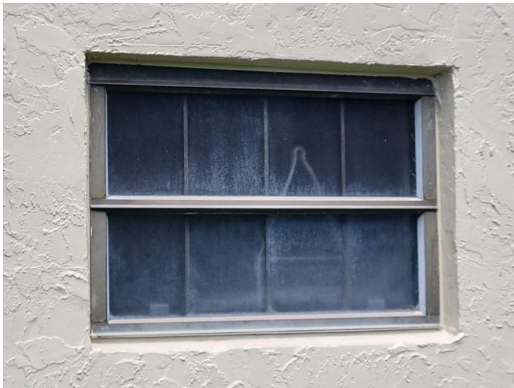
7. Opening Protection – Unrated Unprotected Windows
