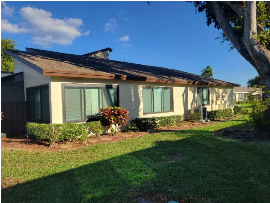
5. Roof Geometry – Right Elevation – Non-Hip
