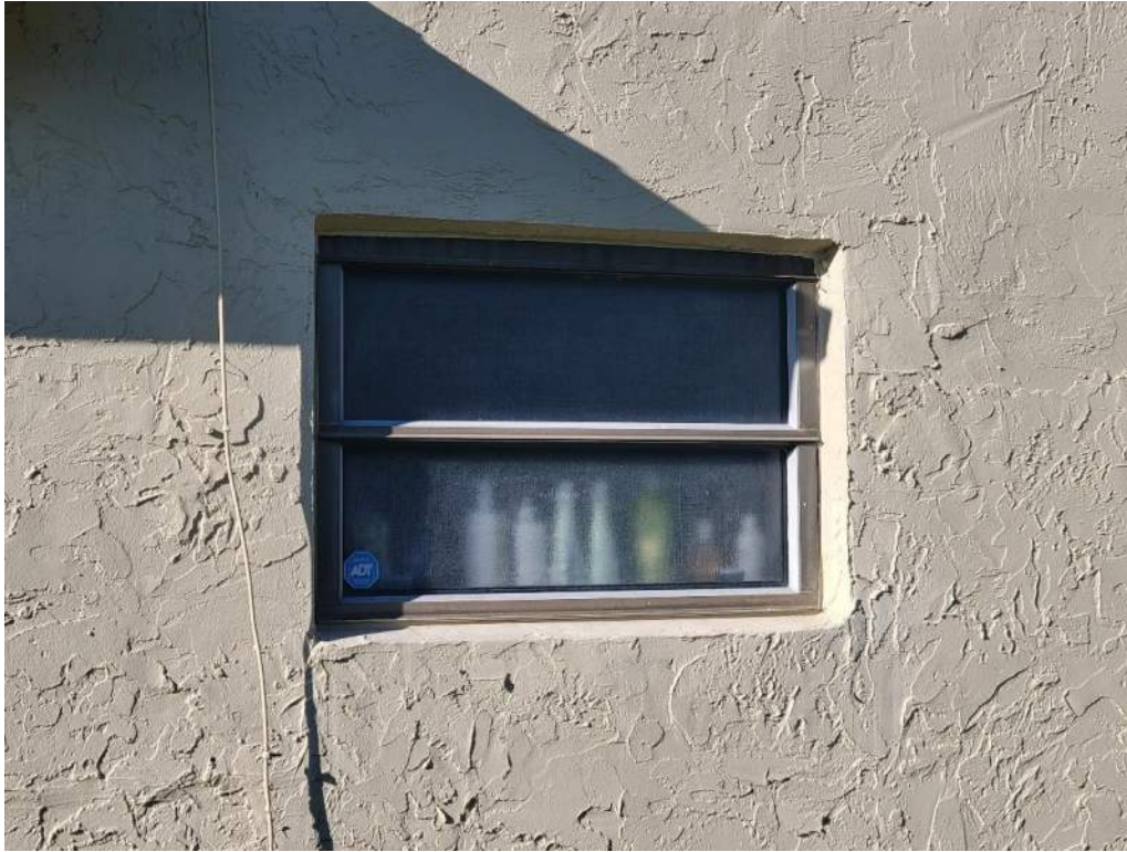
7. Opening Protection – Unrated Unprotected Windows
