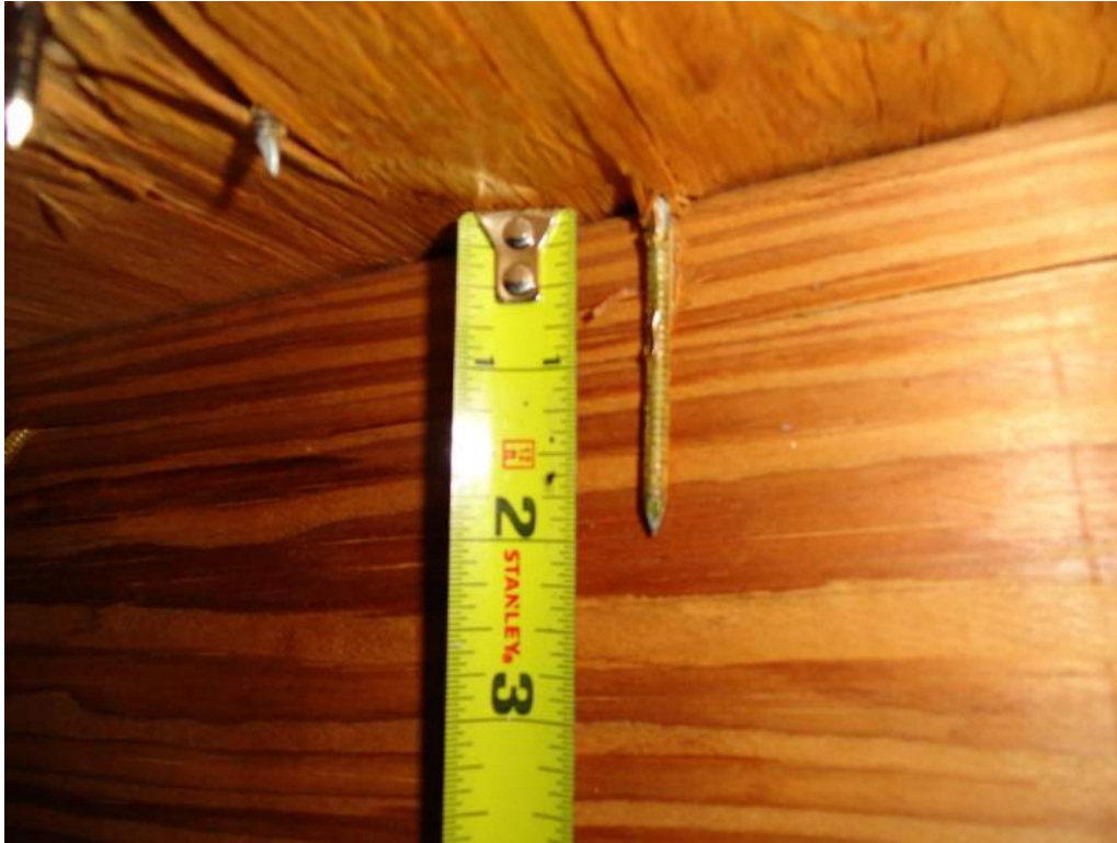
3. Roof Deck Attachment – 8d Nails
