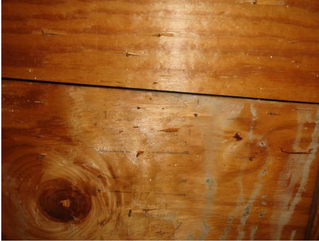
3. Roof Deck Attachment – 19/32" Plywood
