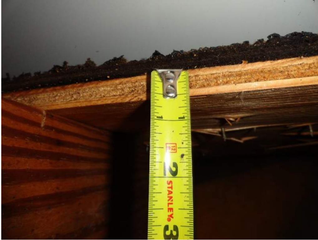
3. Roof Deck Attachment – 19/32" Plywood
