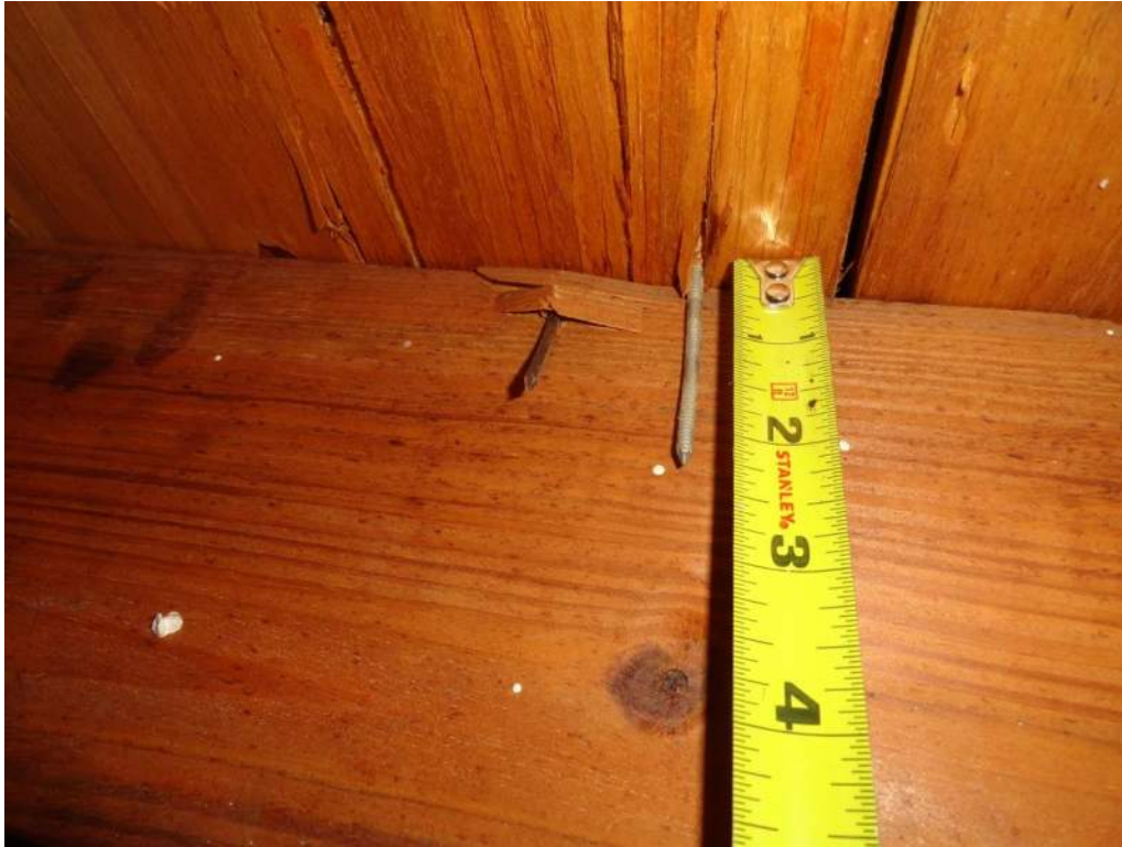
3. Roof Deck Attachment – 8d Nails
