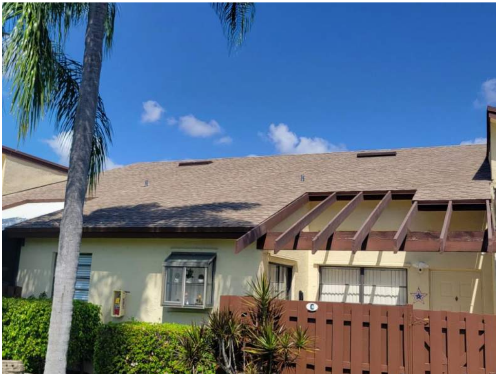
2. Roof Covering – Asphalt Shingles
