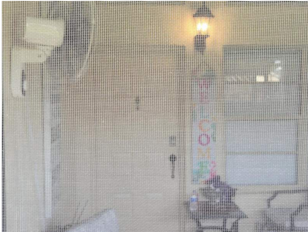
7. Opening Protection – Unprotected Unrated Unglazed Entry Door
