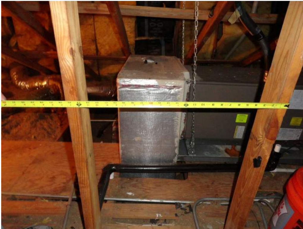
3. Roof Deck Attachment – Trusses at 24" O. C. Max.
