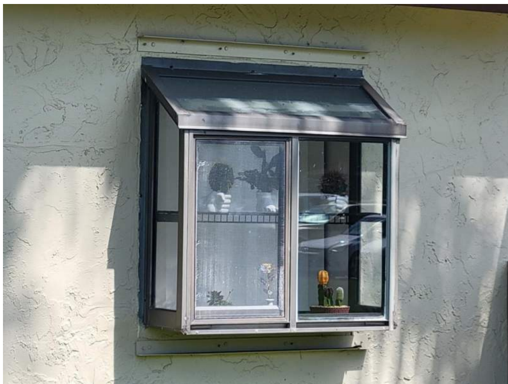
7. Opening Protection – Unrated Unprotected Windows
