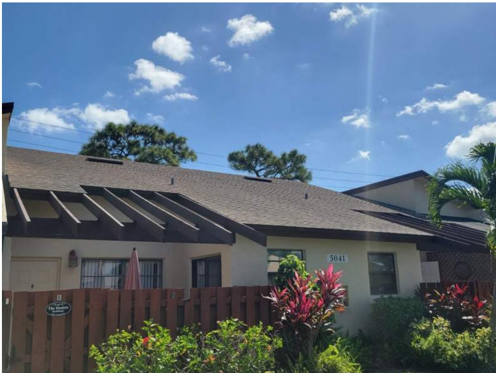
2. Roof Covering – Asphalt Shingles
