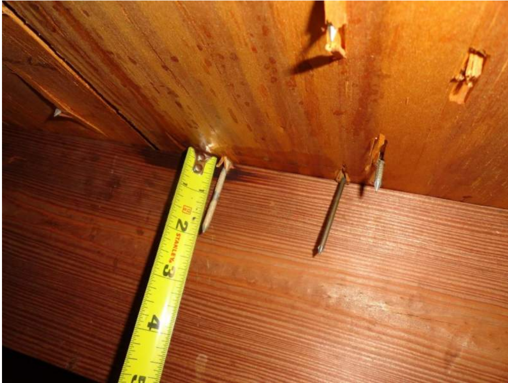
3. Roof Deck Attachment – 8d Nails
