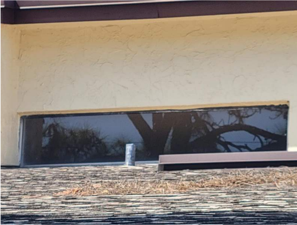
7. Opening Protection – Unrated Unprotected Windows
