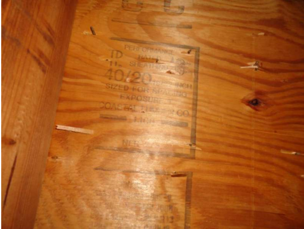
3. Roof Deck Attachment – 19/32" Plywood
