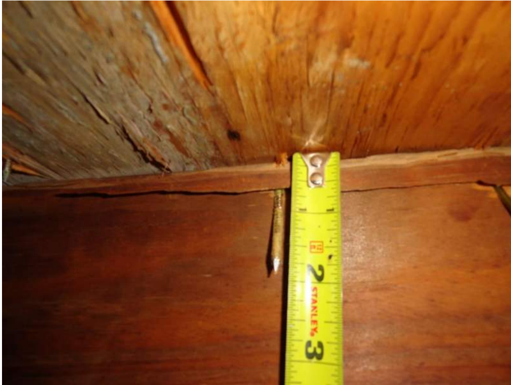
3. Roof Deck Attachment – 8d Nails
