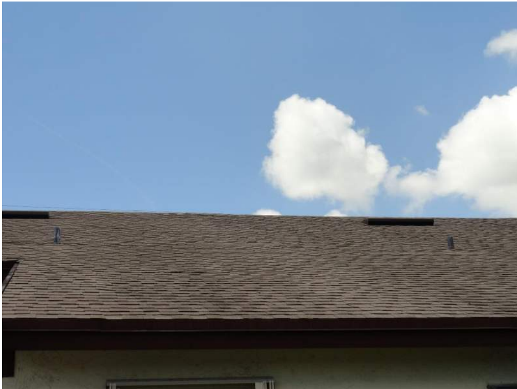
2. Roof Covering – Asphalt Shingles
