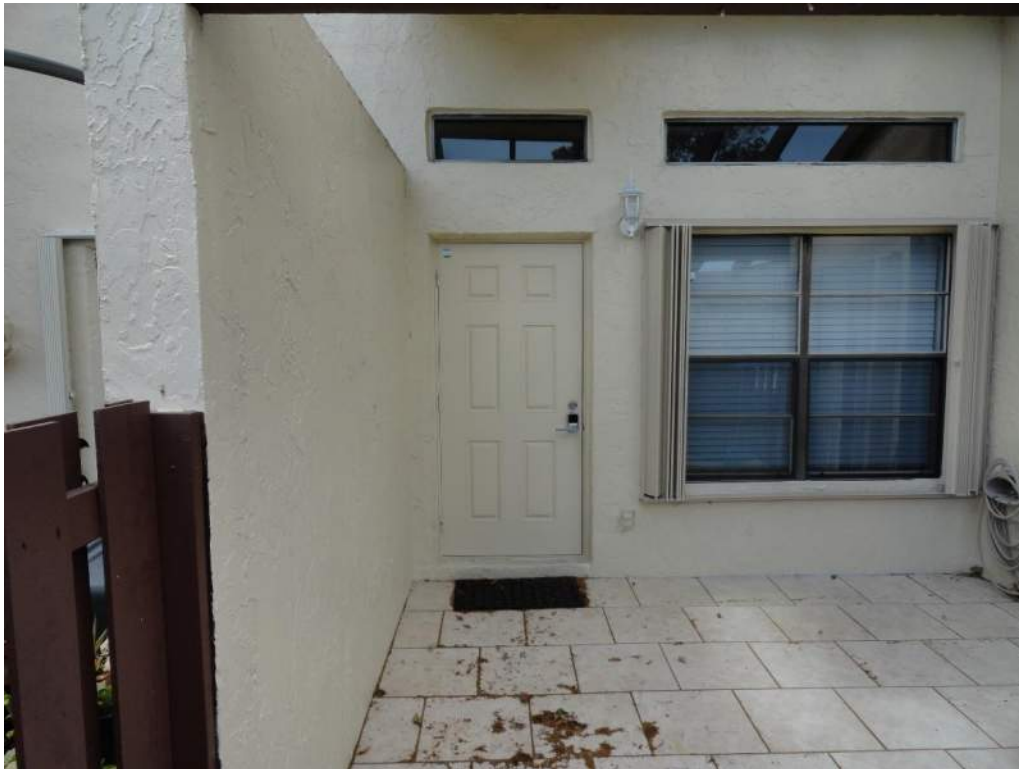
7. Opening Protection – Unprotected Unrated Unglazed Entry Door
