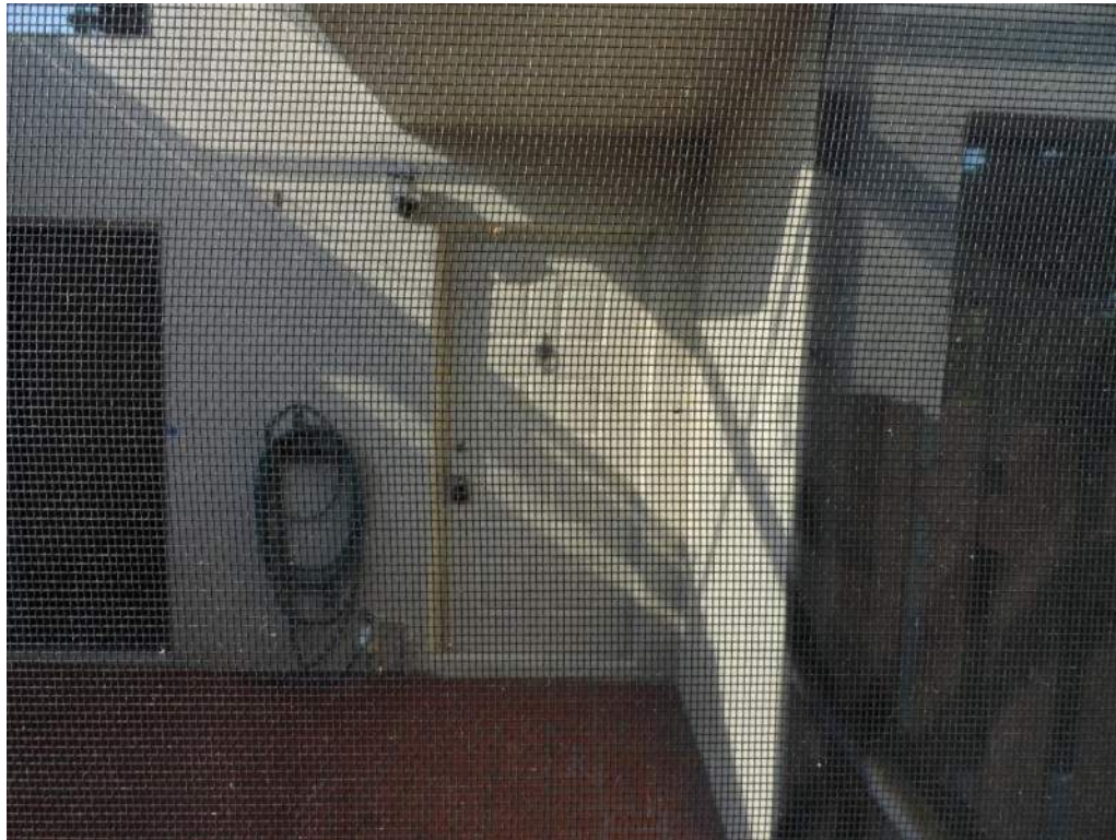
7. Opening Protection – Unprotected Unrated Unglazed Entry Door
