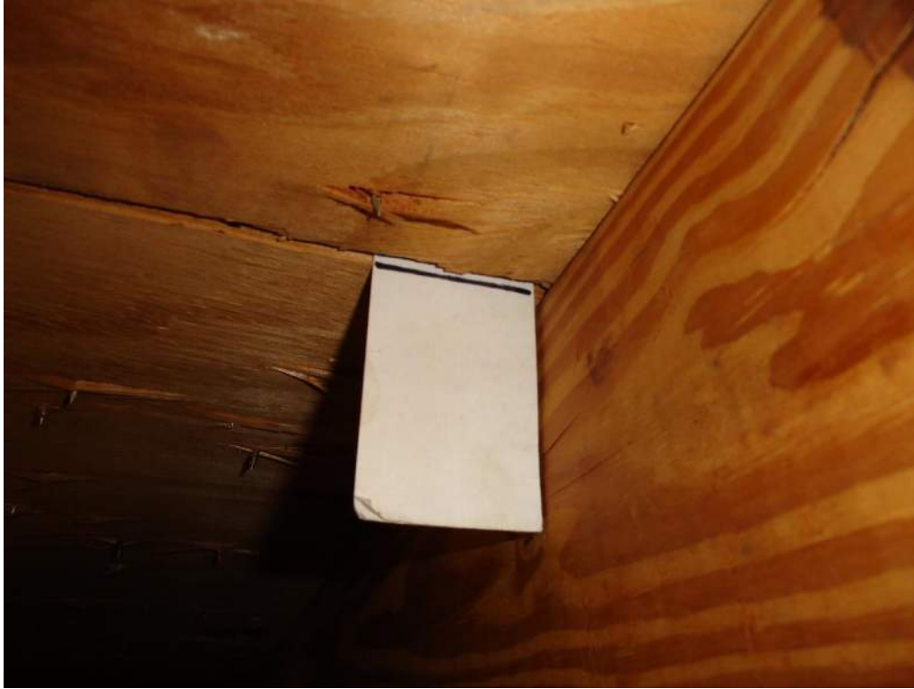
3. Roof Deck Attachment – 5/8" Plywood
