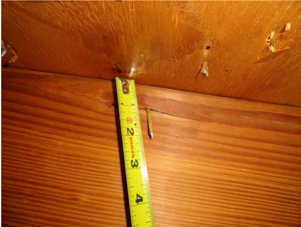
3. Roof Deck Attachment – 8d Nails
