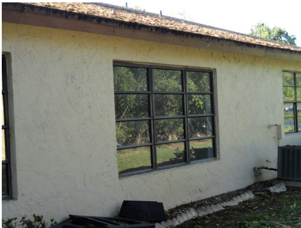
7. Opening Protection – Unprotected Unrated Windows
