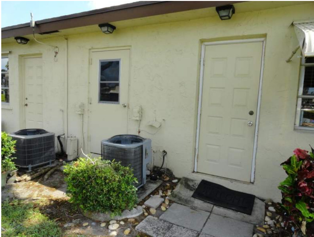
7. Opening Protection – Unprotected Unrated Unglazed Entry Door
