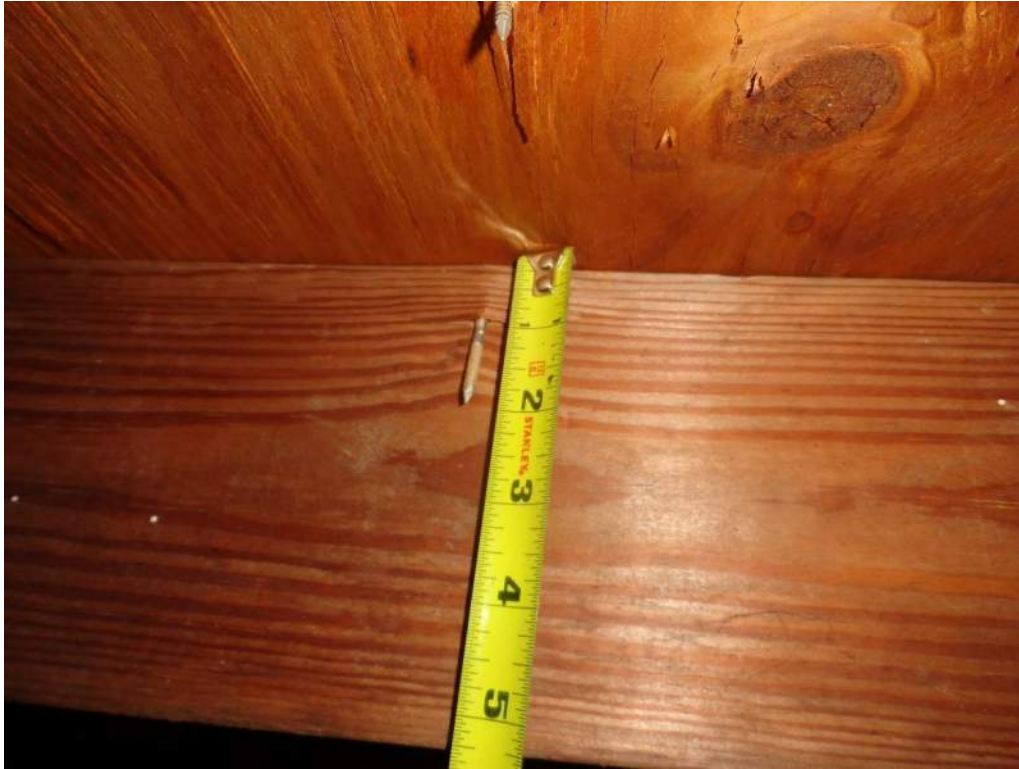
3. Roof Deck Attachment – 8d Nails
