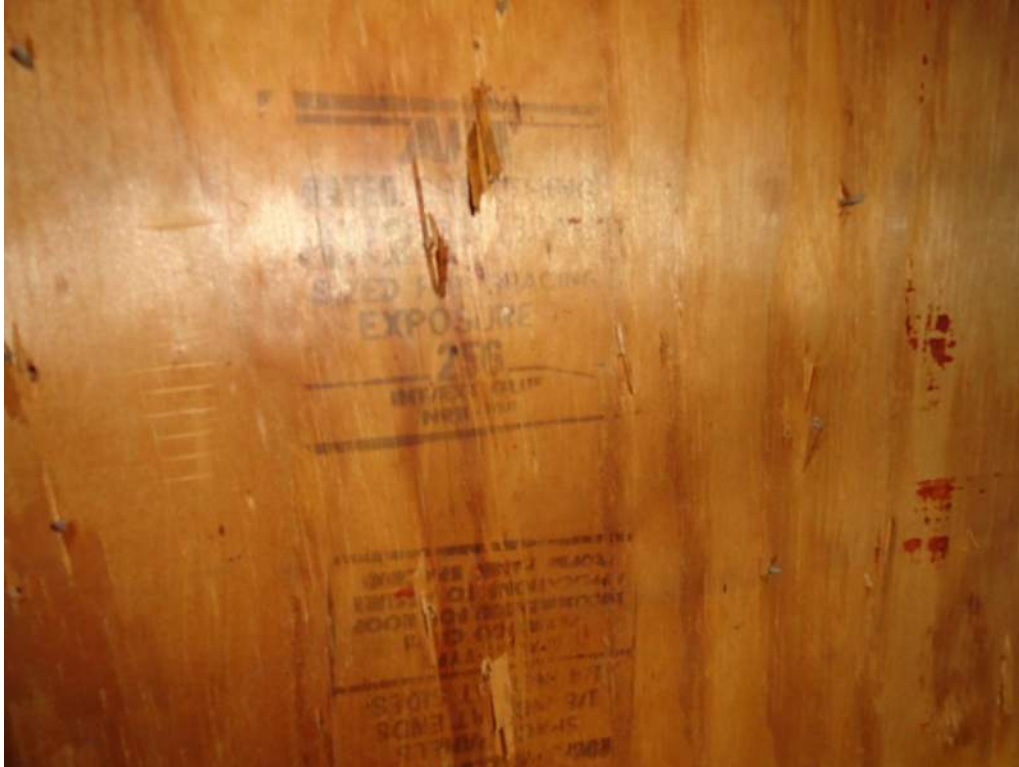
3. Roof Deck Attachment – 19/32" Plywood
