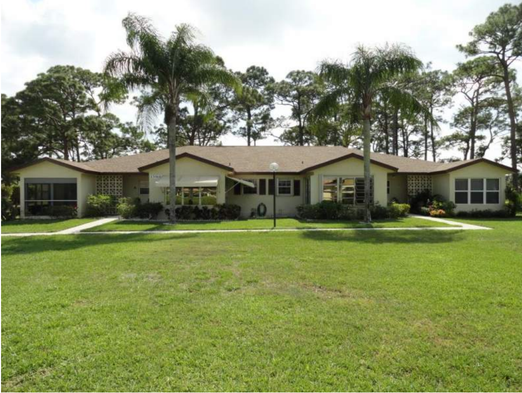
5. Roof Geometry – Front Elevation – Non-Hip
