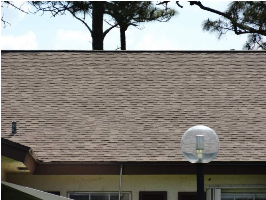
2. Roof Covering – Asphalt Shingles
