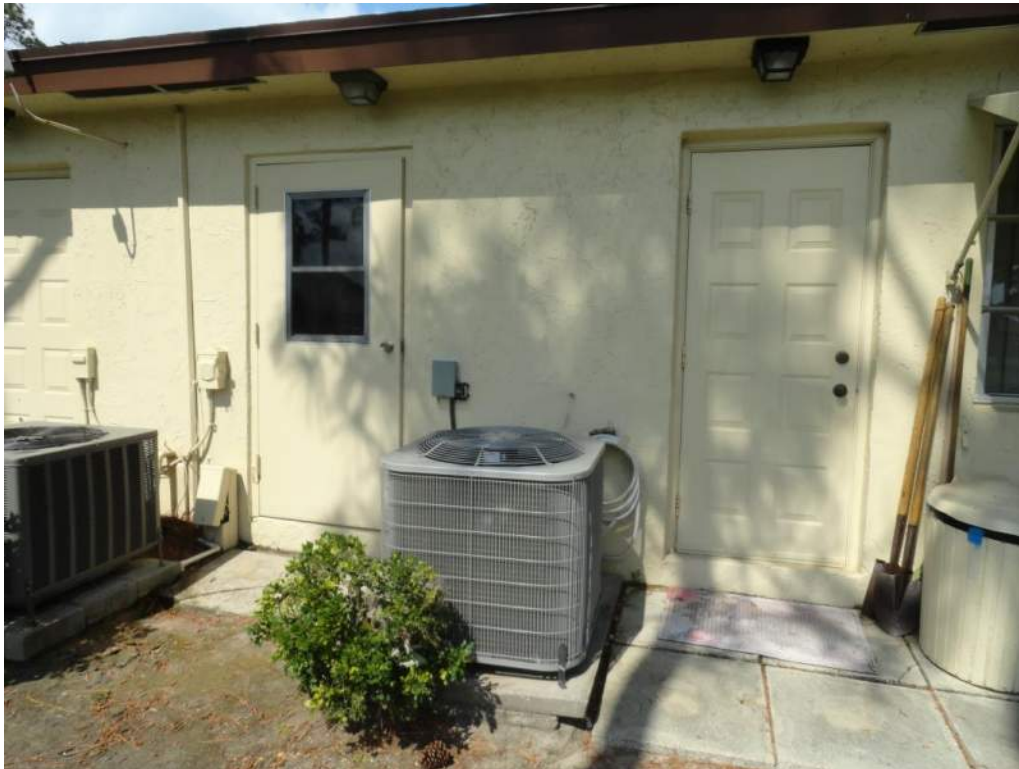
7. Opening Protection – Unprotected Unrated Unglazed Entry Door
