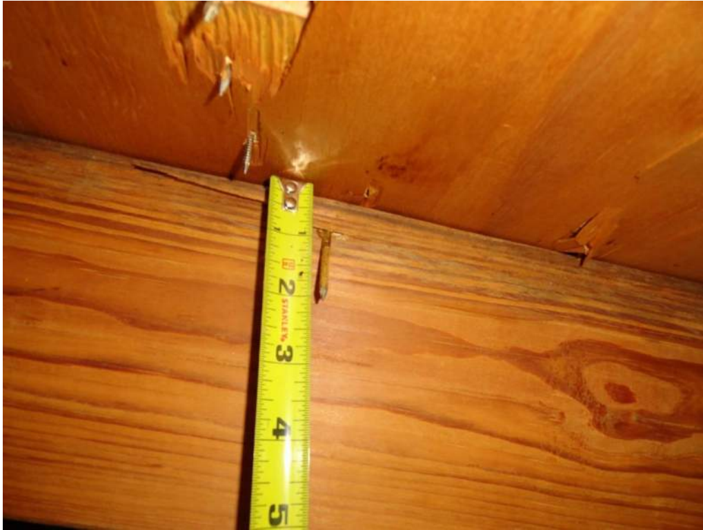
3. Roof Deck Attachment – 8d Nails
