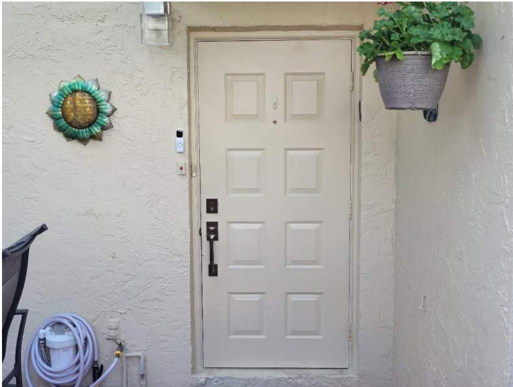
7. Opening Protection – Unprotected Unrated Unglazed Entry Door
