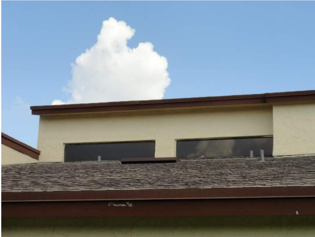
7. Opening Protection – Unrated Unprotected Windows
