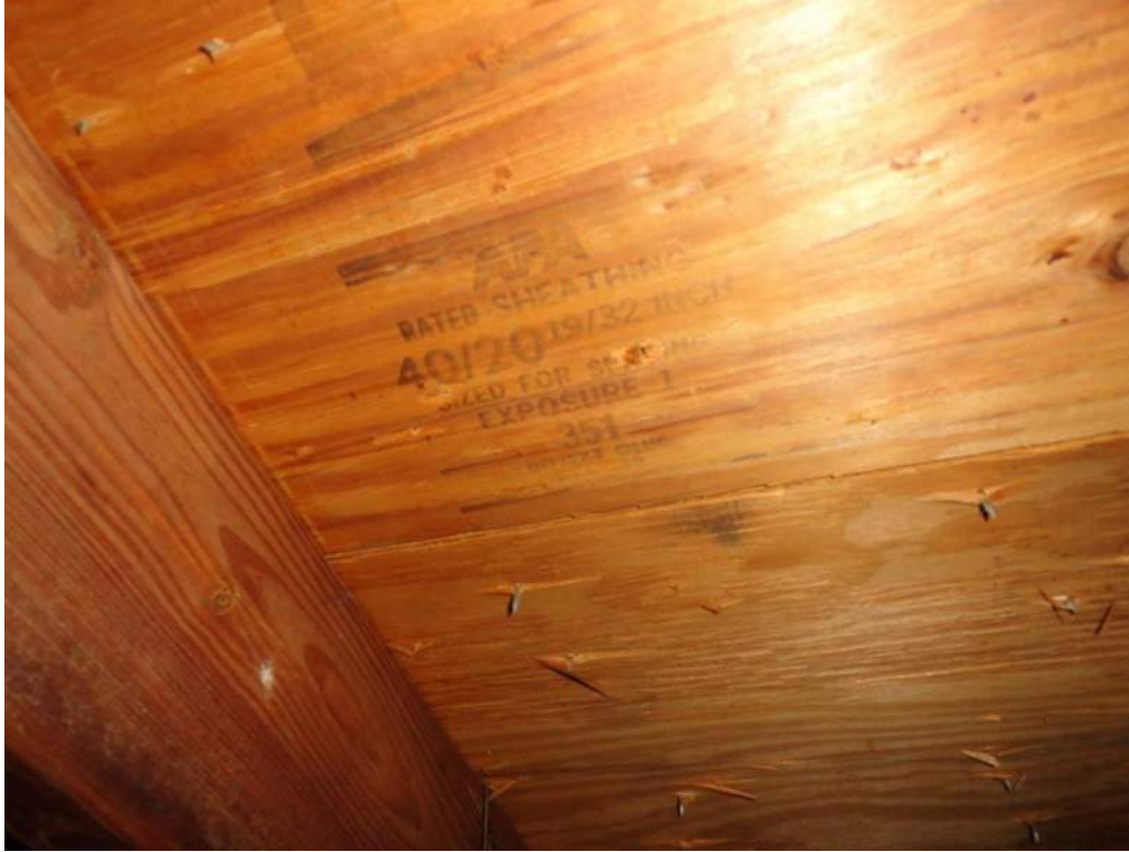
3. Roof Deck Attachment – 19/32" Plywood
