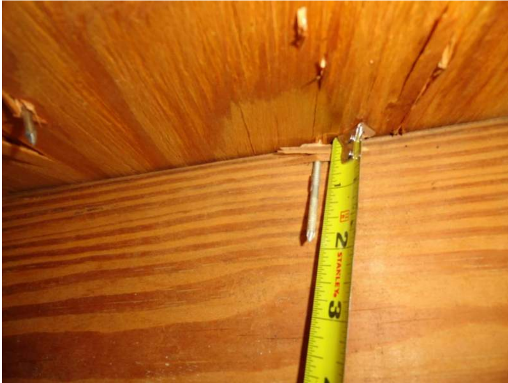
3. Roof Deck Attachment – 8d Nails
