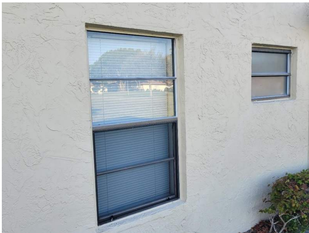
7. Opening Protection – Unrated Unprotected Windows
