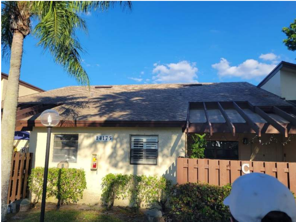
2. Roof Covering – Asphalt Shingles
