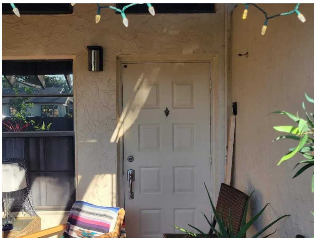
7. Opening Protection – Unprotected Unrated Unglazed Entry Door
