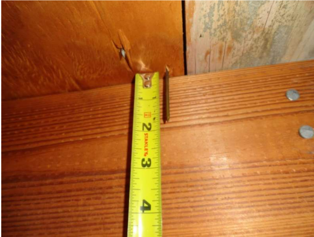
3. Roof Deck Attachment – 8d Nails
