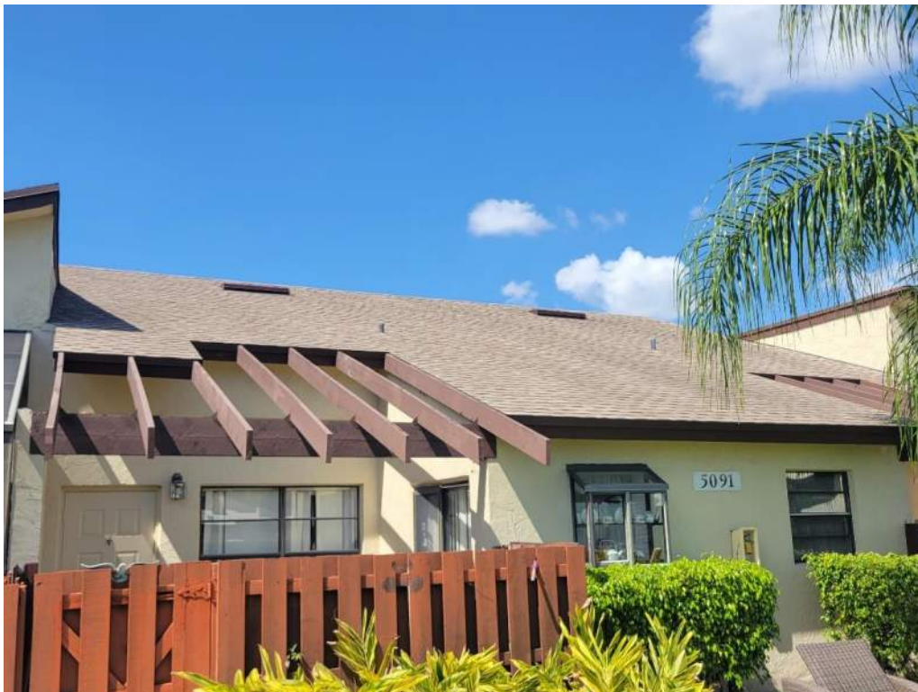
2. Roof Covering – Asphalt Shingles
