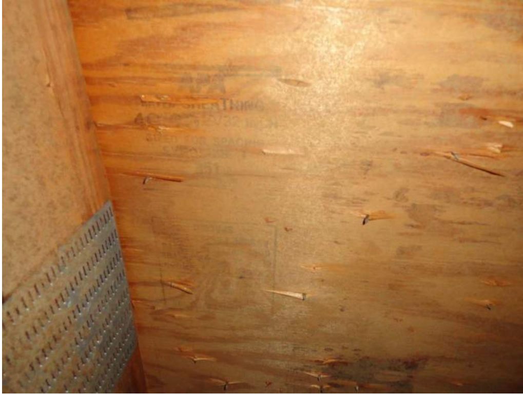
3. Roof Deck Attachment – 19/32" Plywood
