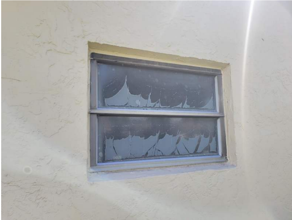
7. Opening Protection – Unrated Unprotected Windows
