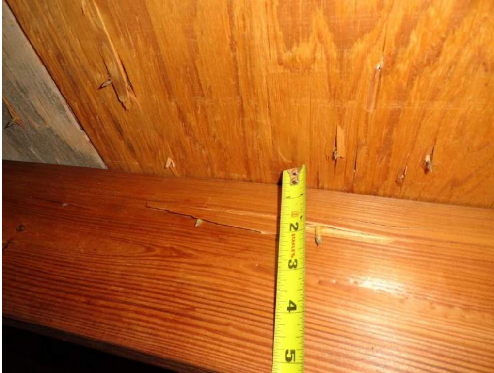
3. Roof Deck Attachment – 8d Nails
