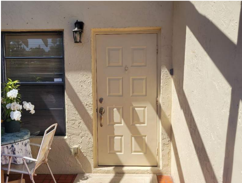
7. Opening Protection – Unprotected Unrated Unglazed Entry Door
