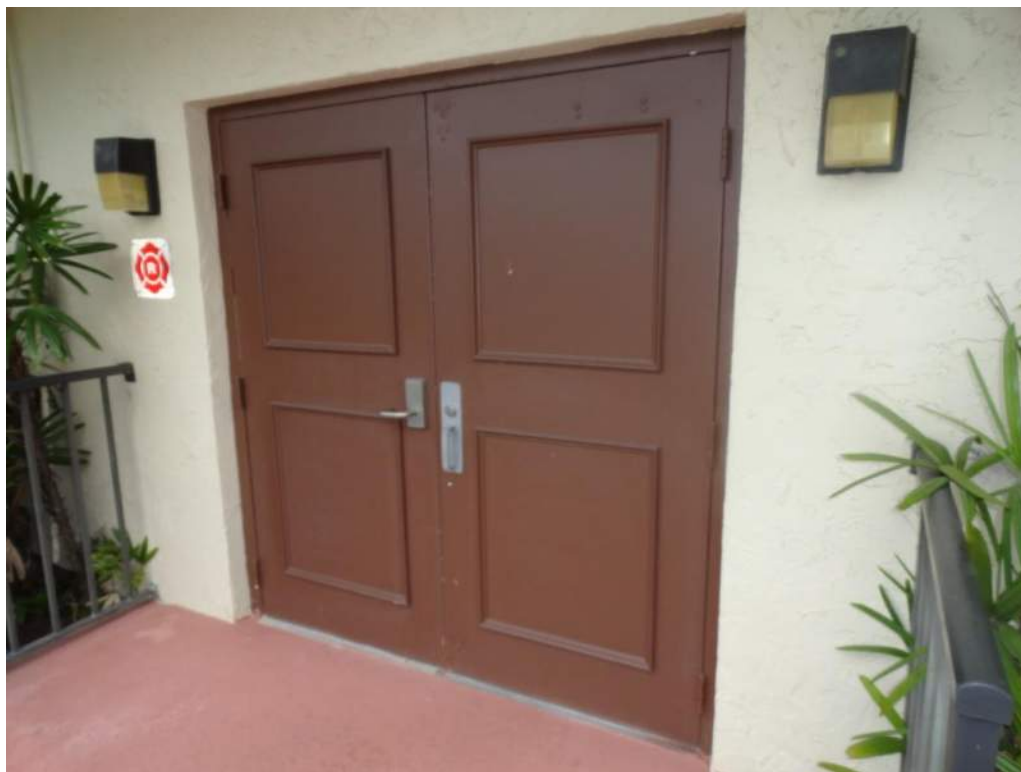
7. Opening Protection – Unprotected Unrated Unglazed Entry Door
