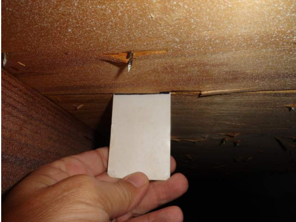
3. Roof Deck Attachment – 5/8" Plywood
