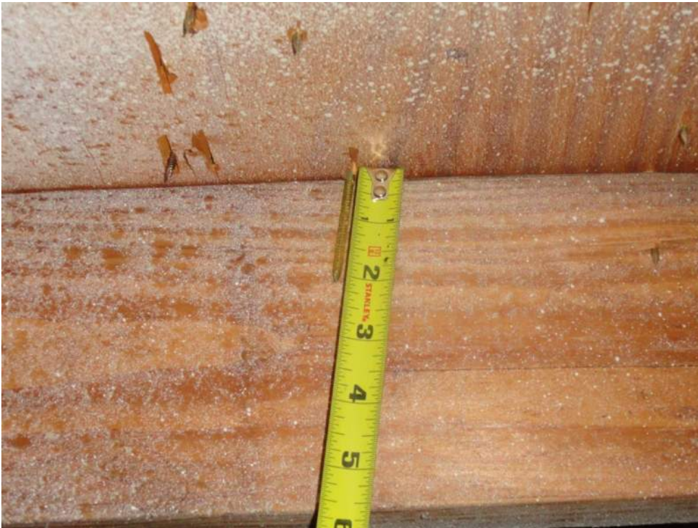
3. Roof Deck Attachment – 8d Nails
