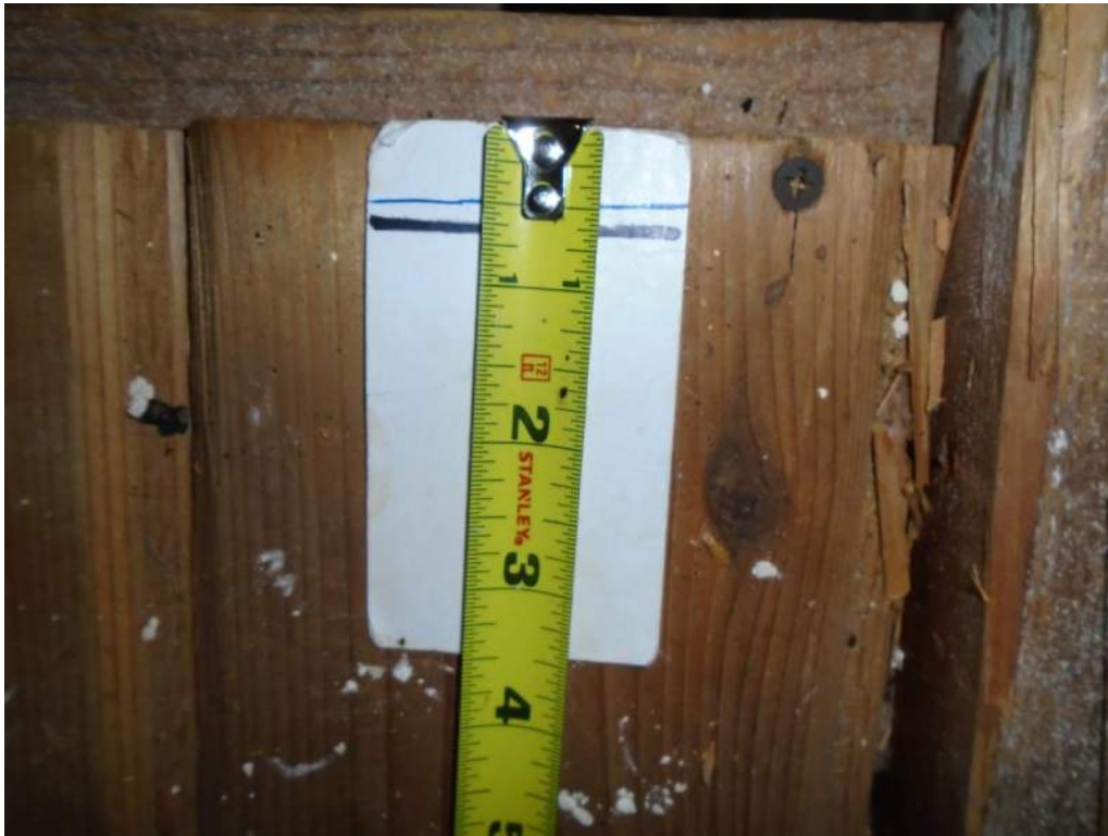
3. Roof Deck Attachment – 5/8" Plywood
