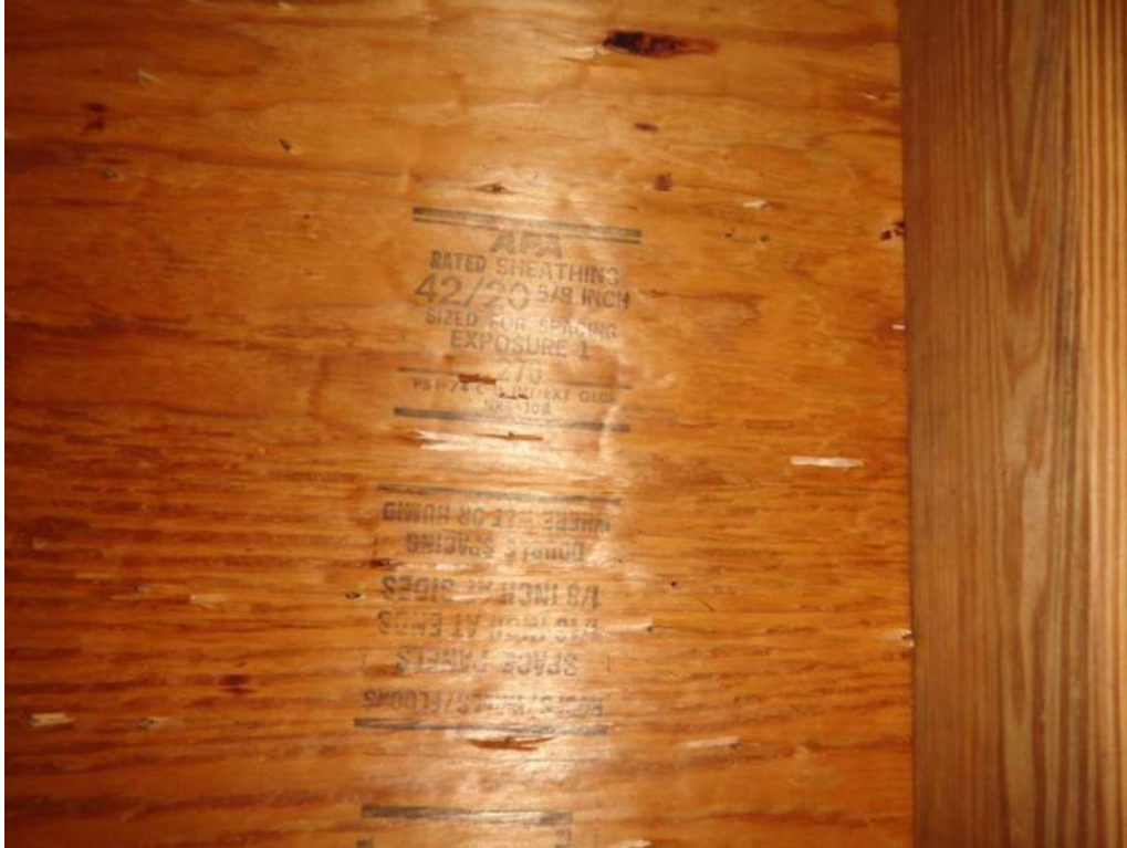
3. Roof Deck Attachment – 19/32" Plywood
