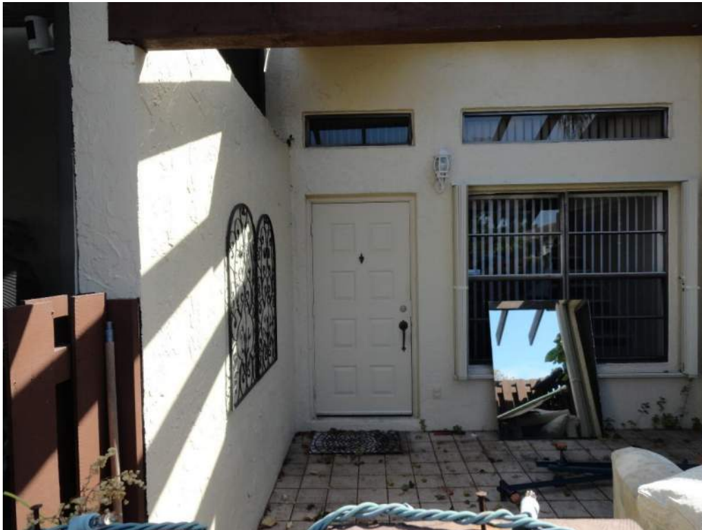
7. Opening Protection – Unprotected Unrated Unglazed Entry Door
