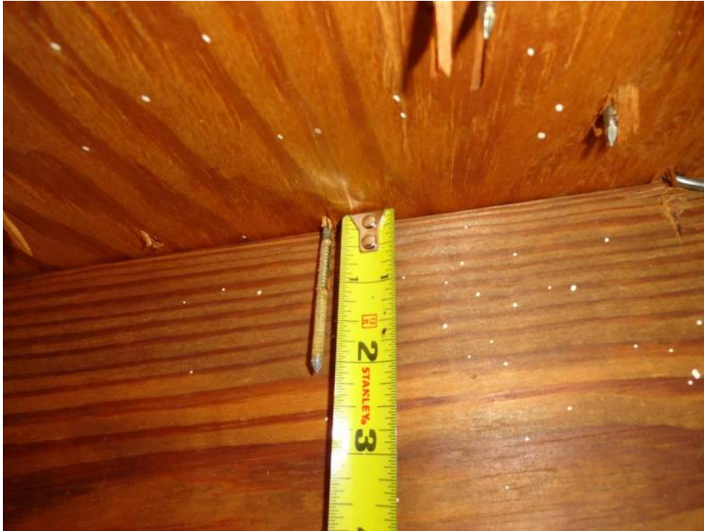
3. Roof Deck Attachment – 8d Nails
