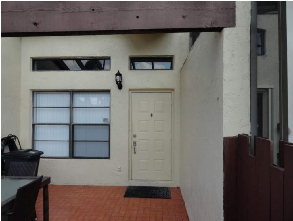
7. Opening Protection – Unprotected Unrated Unglazed Entry Door
