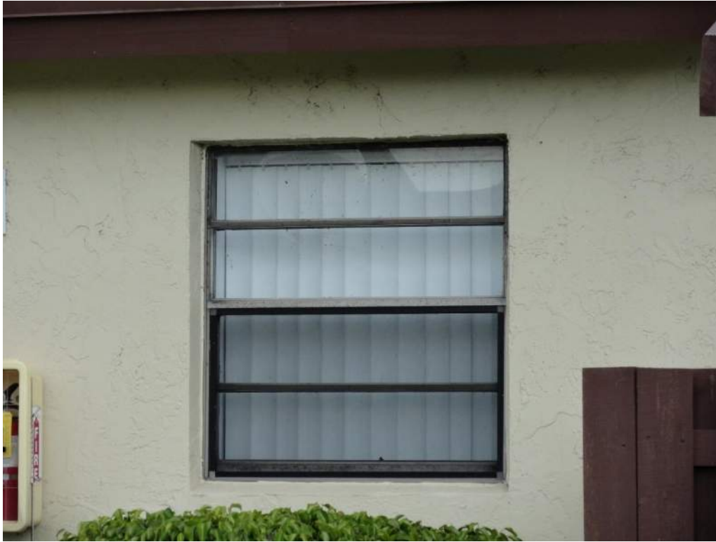
7. Opening Protection – Unrated Unprotected Windows
