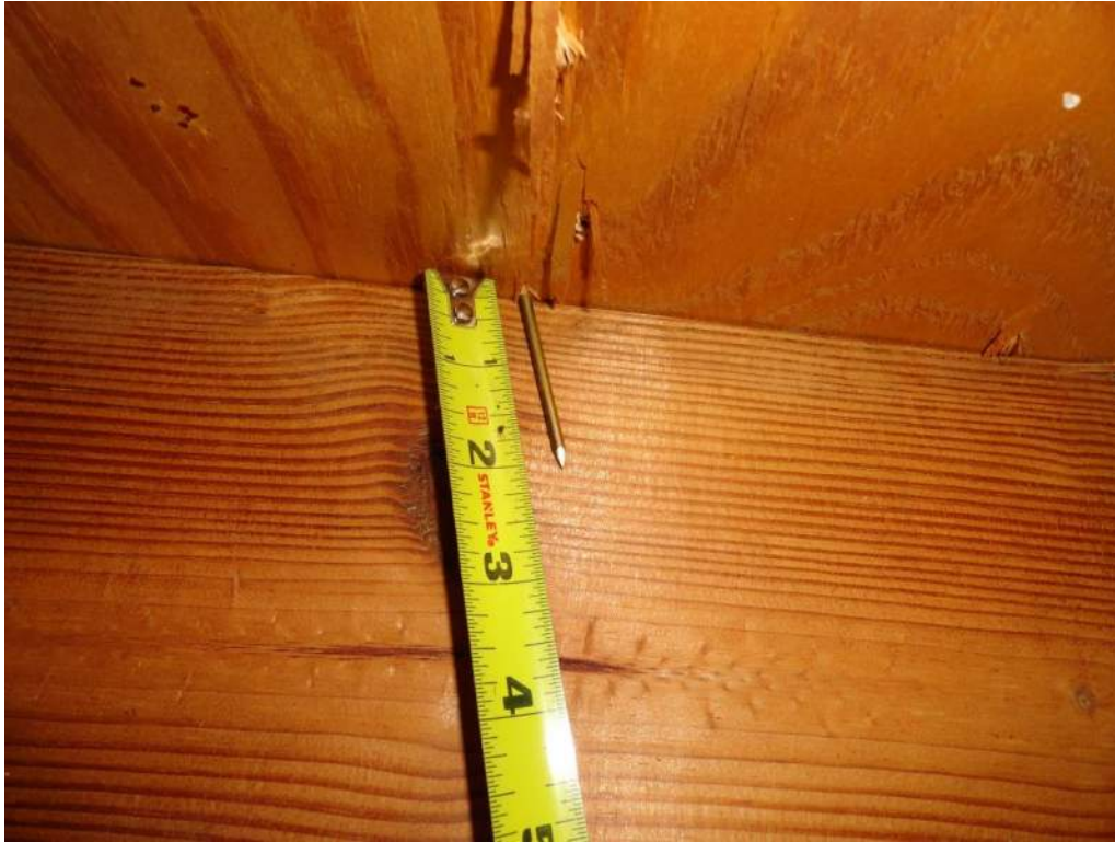
3. Roof Deck Attachment – 8d Nails
