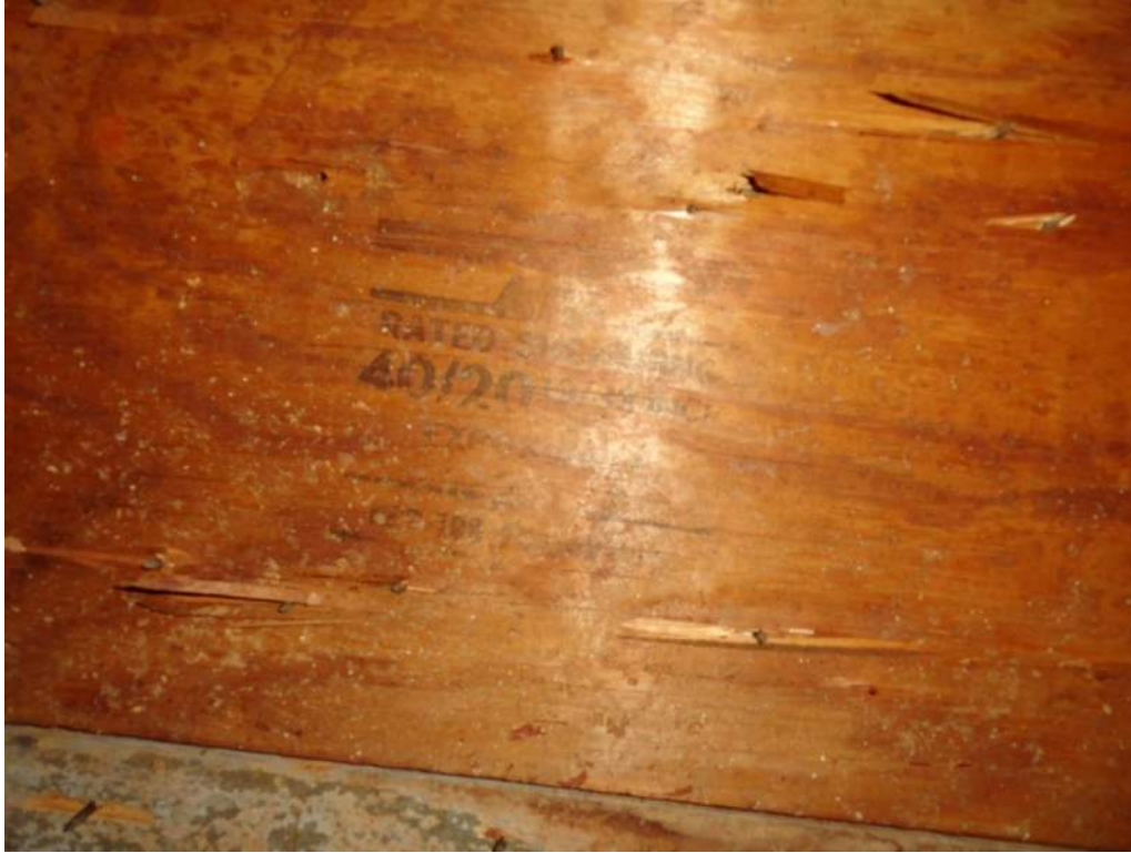
3. Roof Deck Attachment – 19/32" Plywood
