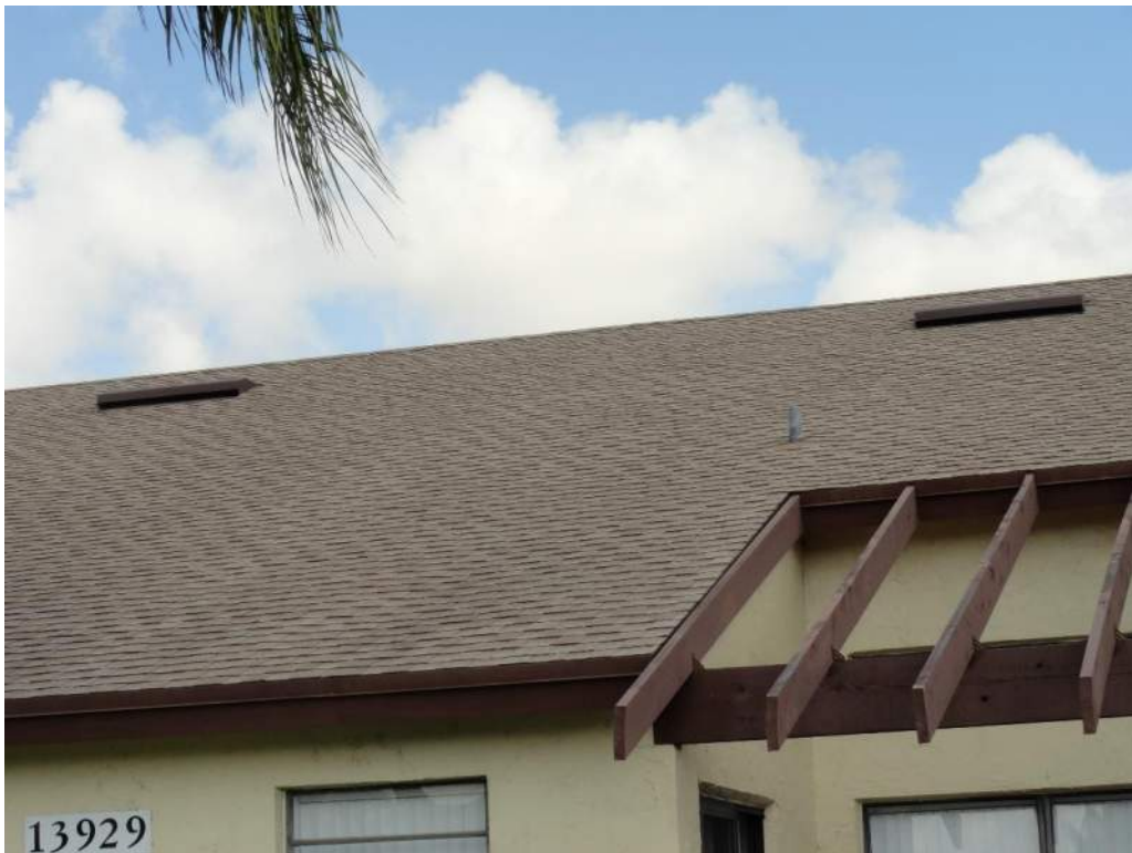
2. Roof Covering – Asphalt Shingles
