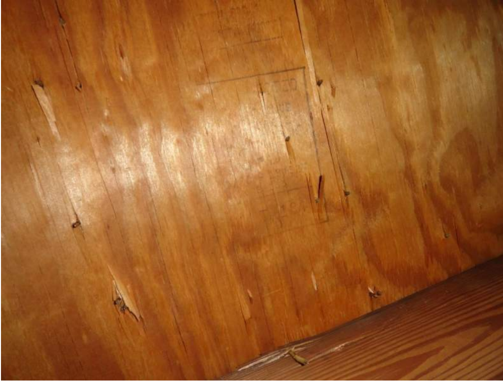
3. Roof Deck Attachment – 19/32" Plywood
