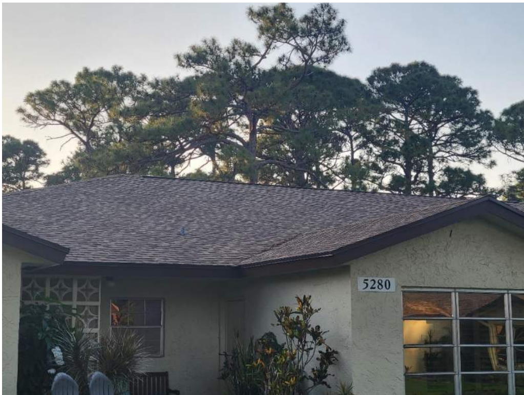
2. Roof Covering – Asphalt Shingles
