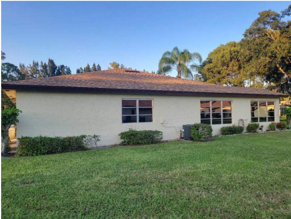
5. Roof Geometry – Left Elevation – Hip
