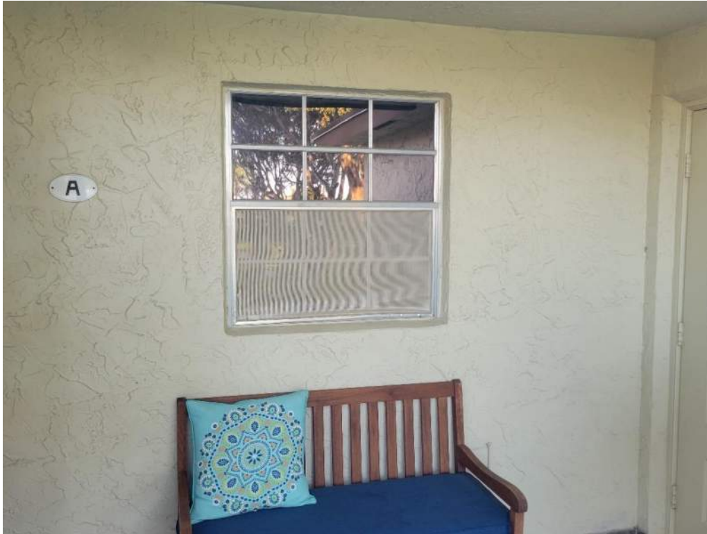
7. Opening Protection – Unrated Unprotected Windows
