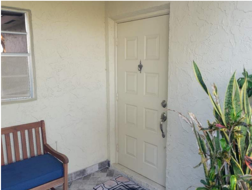
7. Opening Protection – Unprotected Unrated Unglazed Entry Door
