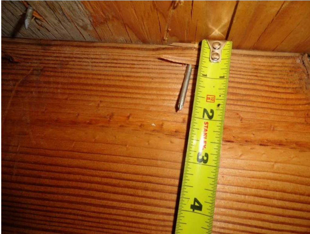
3. Roof Deck Attachment – 8d Nails
