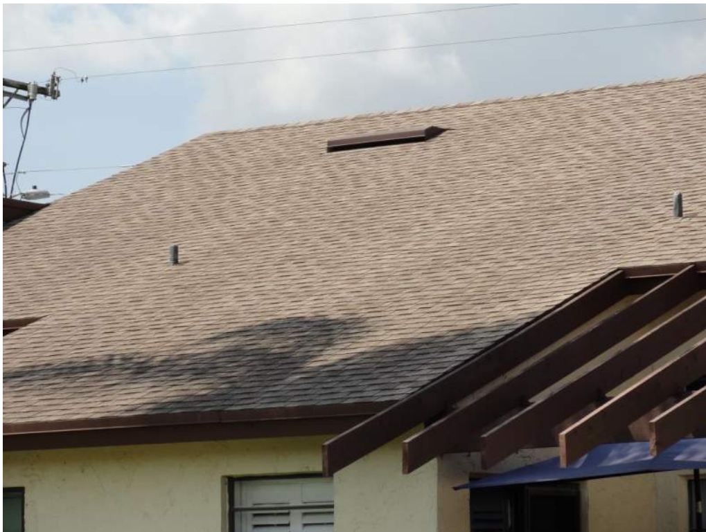
2. Roof Covering – Asphalt Shingles
