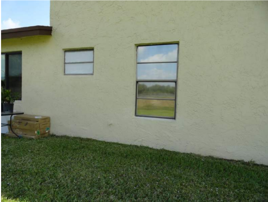
7. Opening Protection – Unrated Unprotected Windows
