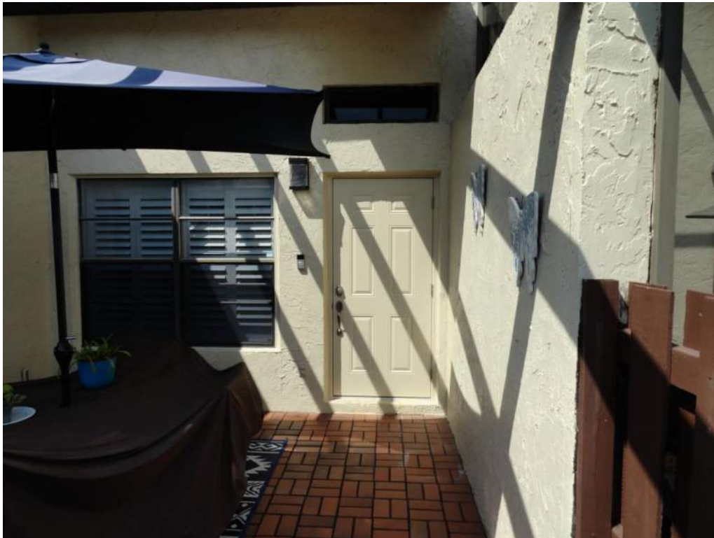
7. Opening Protection – Unprotected Unrated Unglazed Entry Door
