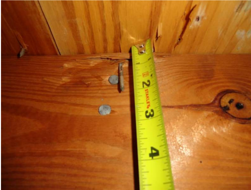
3. Roof Deck Attachment – 8d Nails
