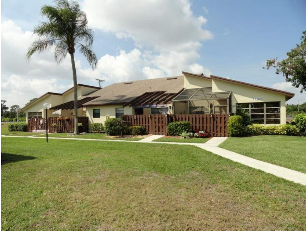
5. Roof Geometry – Front Elevation – Non-Hip
