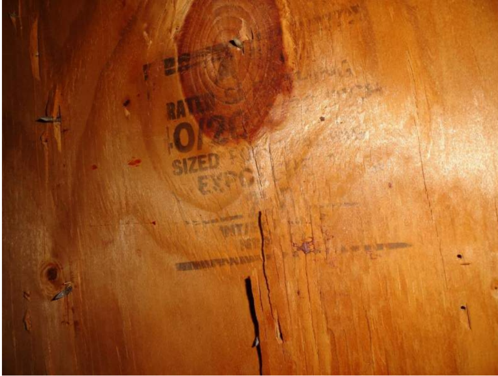
3. Roof Deck Attachment – 19/32" Plywood
