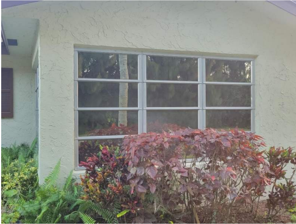
7. Opening Protection – Unrated Unprotected Windows
