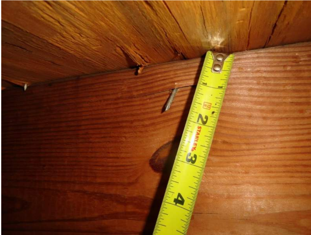
3. Roof Deck Attachment – 8d Nails
