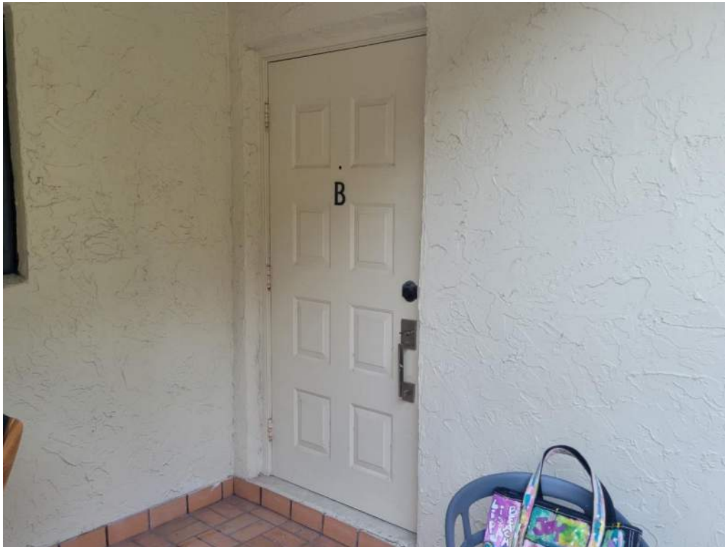
7. Opening Protection – Unprotected Unrated Unglazed Entry Door
