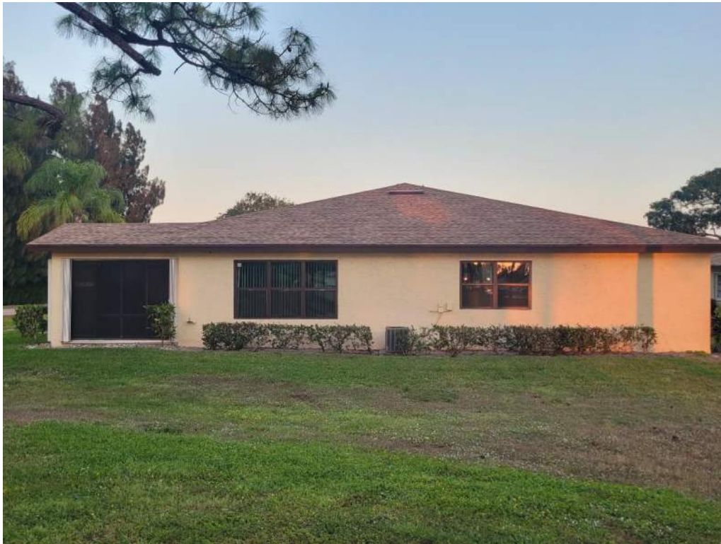
5. Roof Geometry – Right Elevation – Hip
