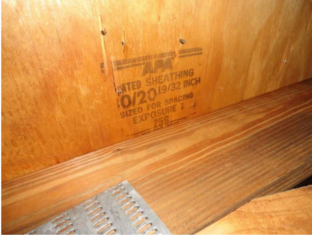
3. Roof Deck Attachment – 19/32" Plywood
