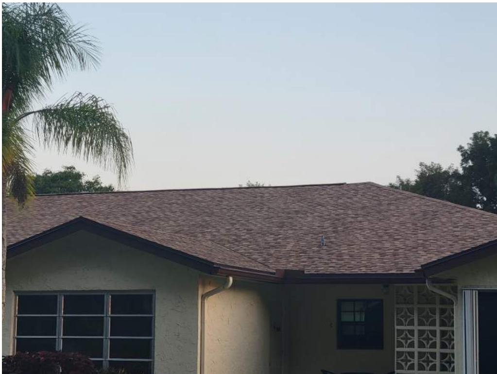
2. Roof Covering – Asphalt Shingles
