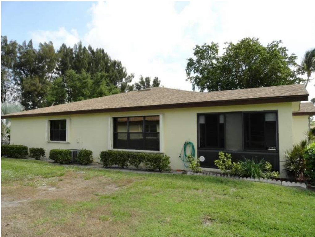
5. Roof Geometry – Left Elevation – Hip
