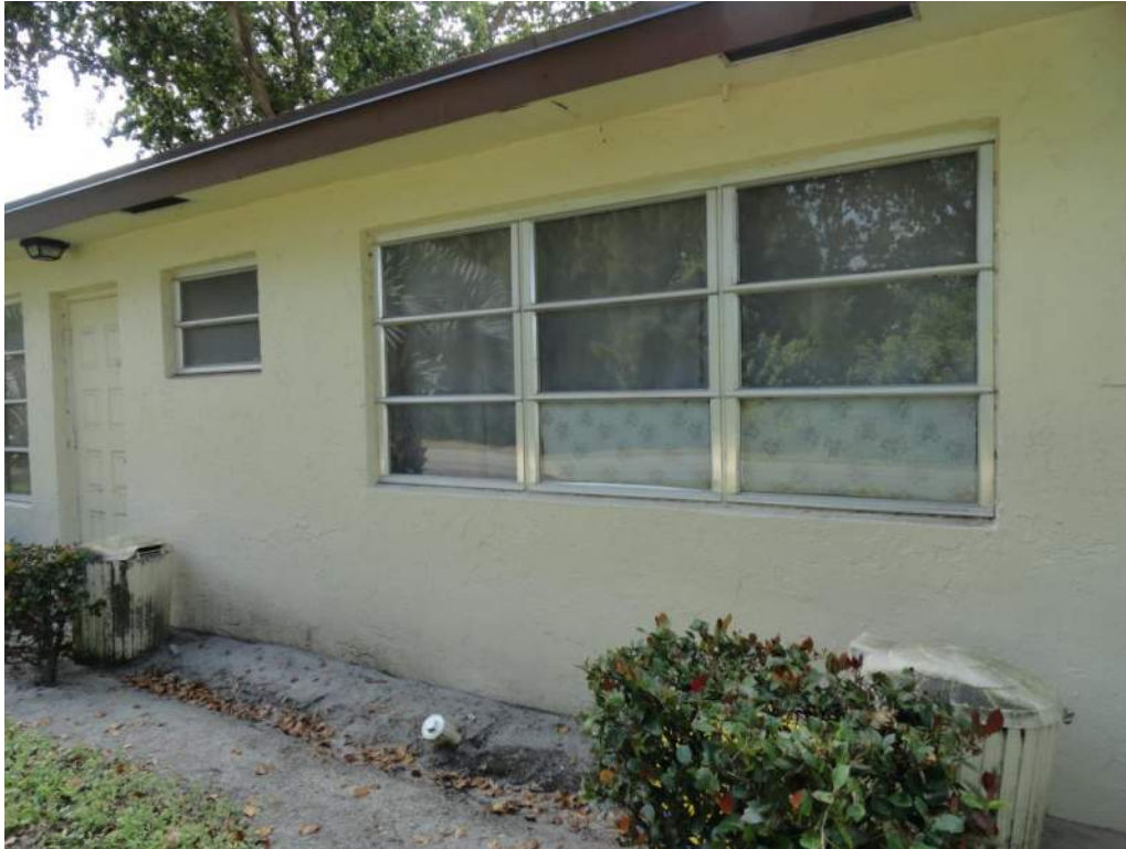
7. Opening Protection – Unrated Unprotected Windows
