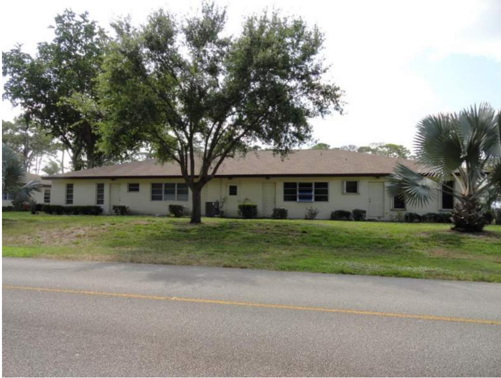
5. Roof Geometry – Rear Elevation – Hip
