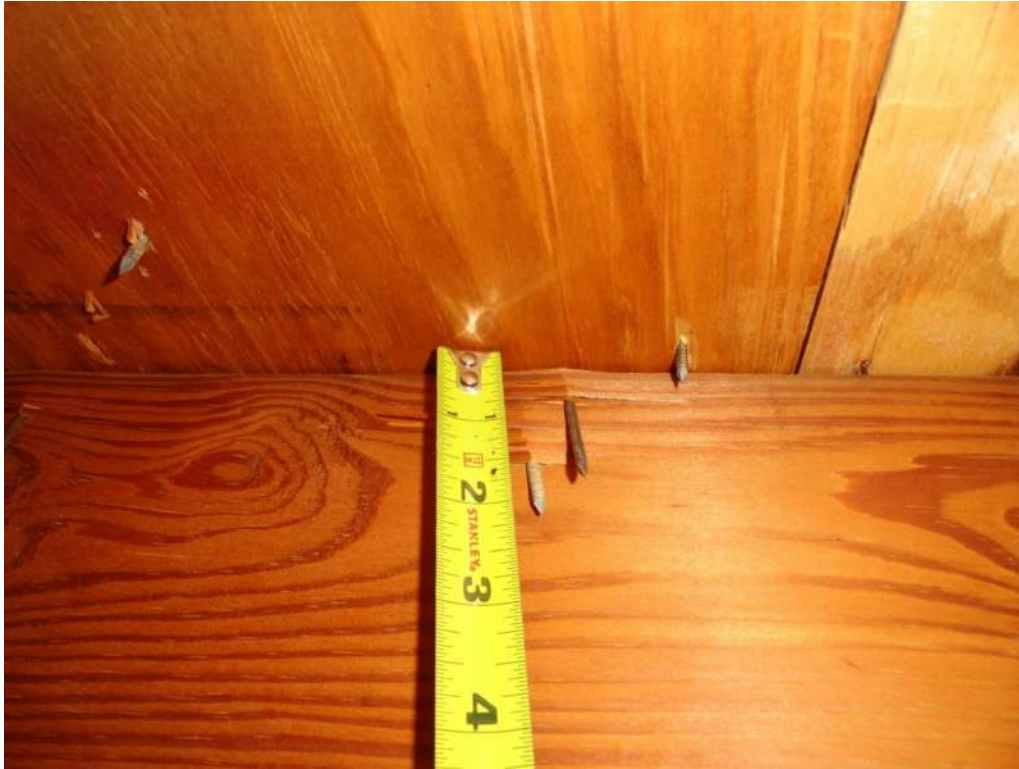
3. Roof Deck Attachment – 8d Nails
