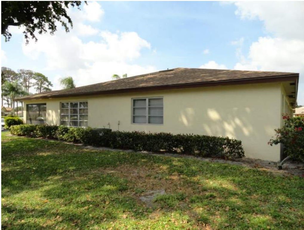
5. Roof Geometry – Right Elevation – Hip
