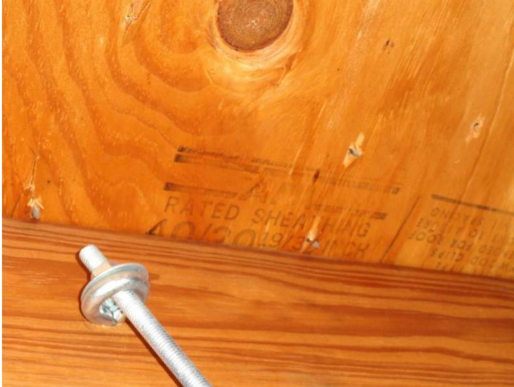
3. Roof Deck Attachment – 19/32" Plywood
