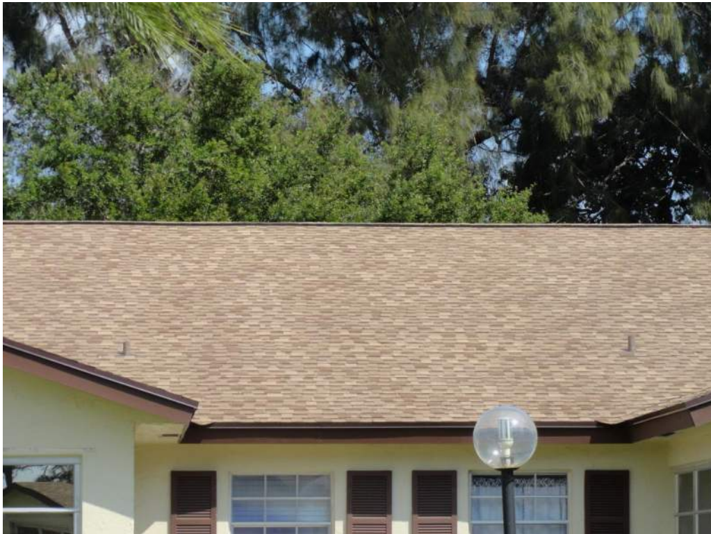
2. Roof Covering – Asphalt Shingles
