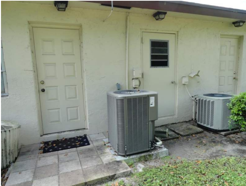
7. Opening Protection – Unprotected Unrated Unglazed Entry Door
