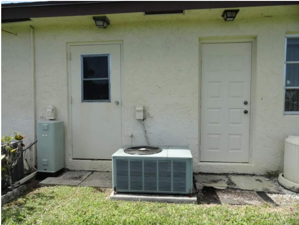
7. Opening Protection – Unprotected Unrated Unglazed Entry Door
