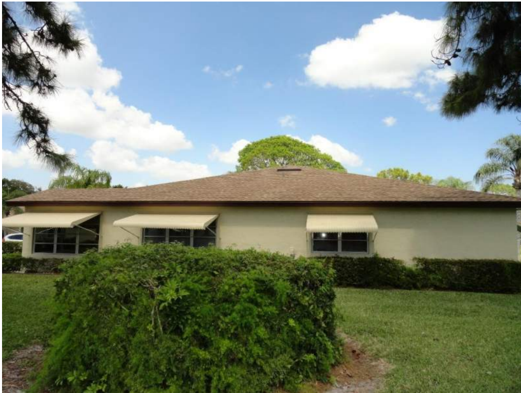
5. Roof Geometry – Right Elevation – Hip
