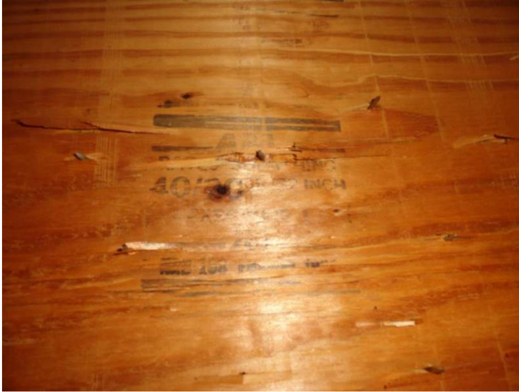
3. Roof Deck Attachment – 19/32" Plywood
