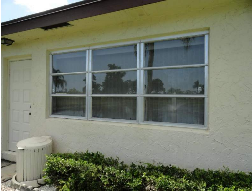
7. Opening Protection – Unrated Unprotected Windows
