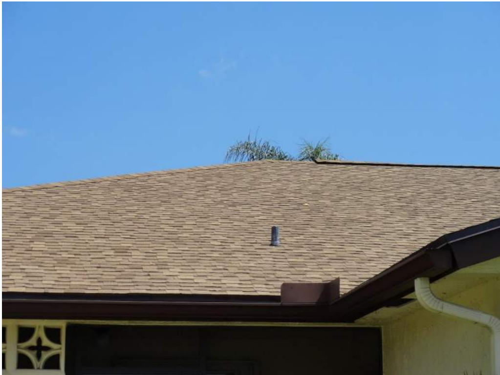
2. Roof Covering – Asphalt Shingles
