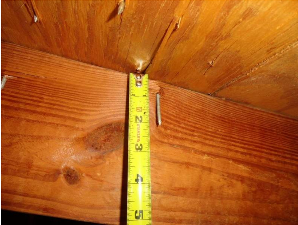
3. Roof Deck Attachment – 8d Nails
