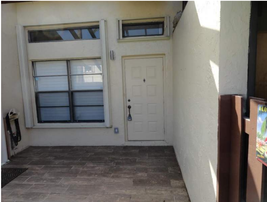
7. Opening Protection – Unprotected Unrated Unglazed Entry Door
