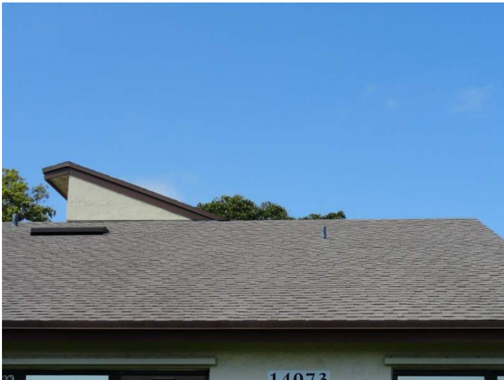
2. Roof Covering – Asphalt Shingles
