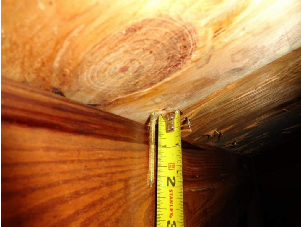
3. Roof Deck Attachment – 8d Nails
