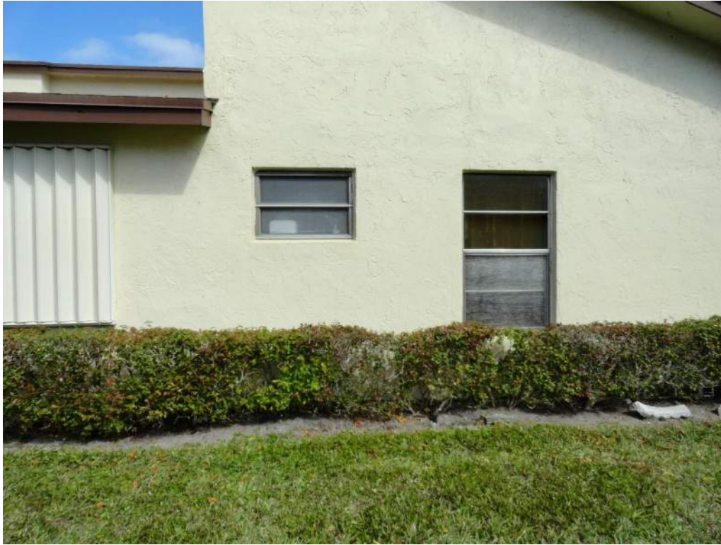
7. Opening Protection – Unrated Unprotected Windows
