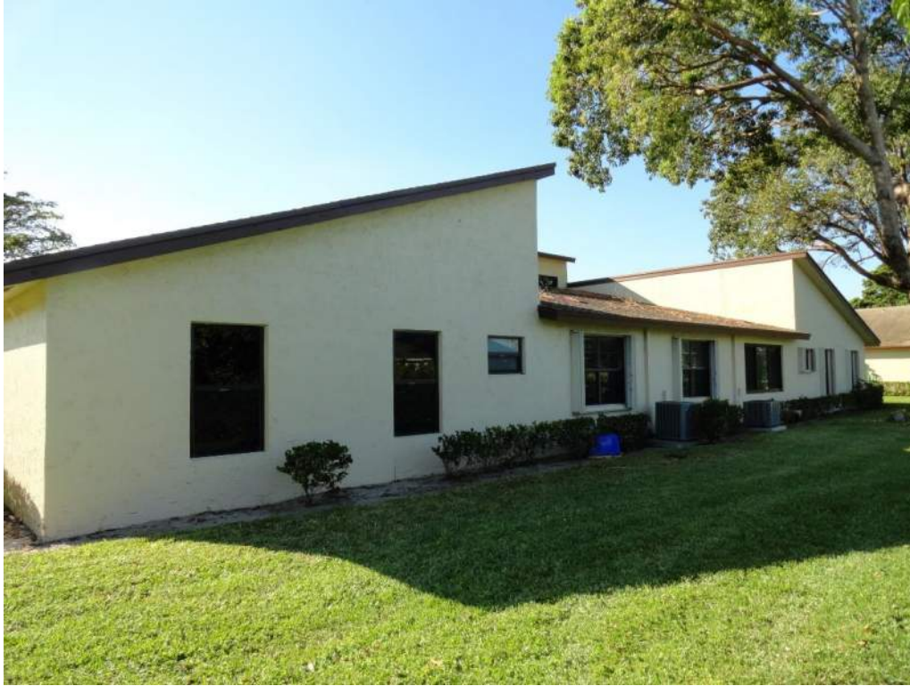
5. Roof Geometry – Rear Elevation – Non-Hip
