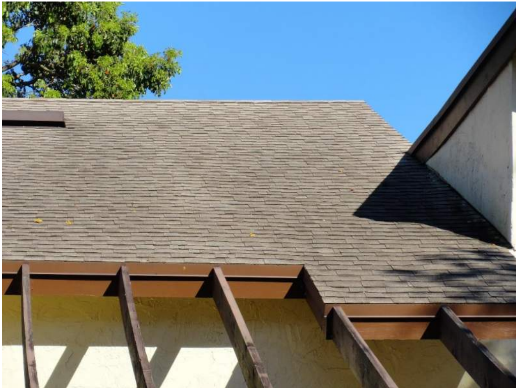
2. Roof Covering – Asphalt Shingles
