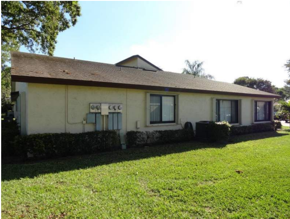
5. Roof Geometry – Left Elevation – Non-Hip
