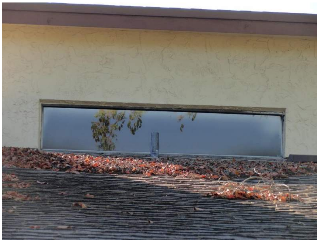
7. Opening Protection – Unrated Unprotected Windows
