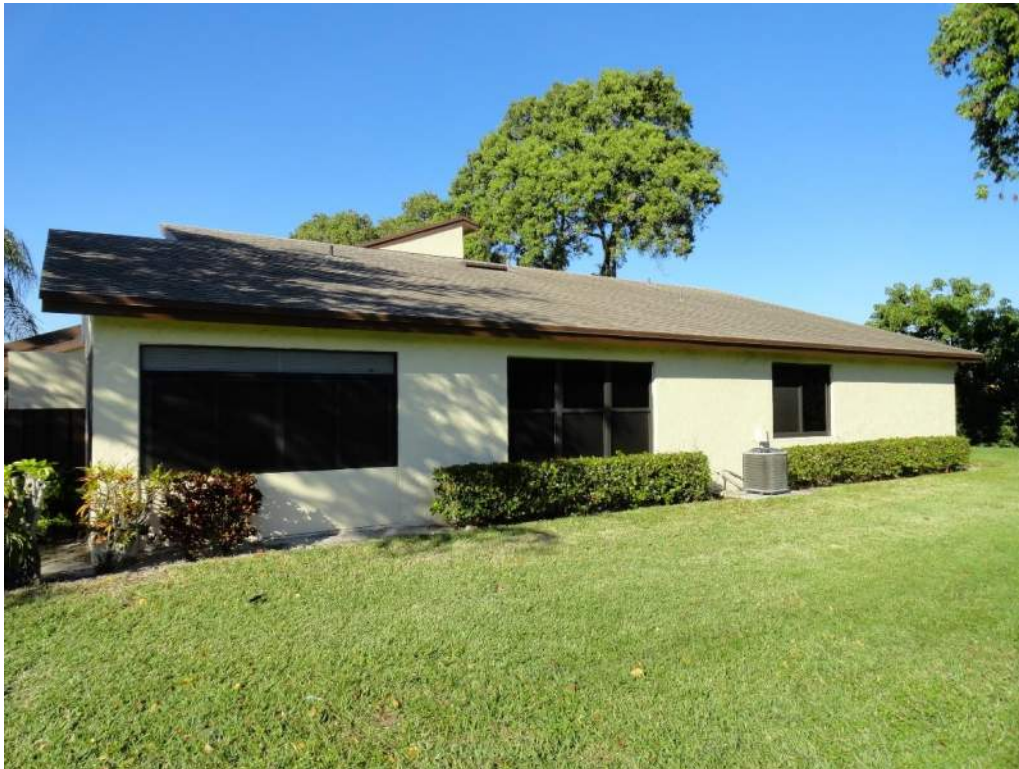
5. Roof Geometry – Right Elevation – Non-Hip
