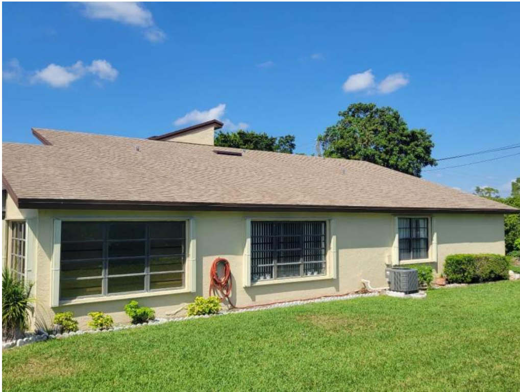
5. Roof Geometry – Right Elevation – Hip
