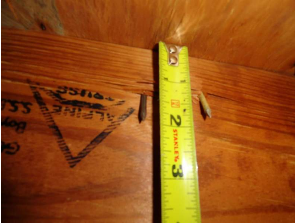
3. Roof Deck Attachment – 8d Nails
