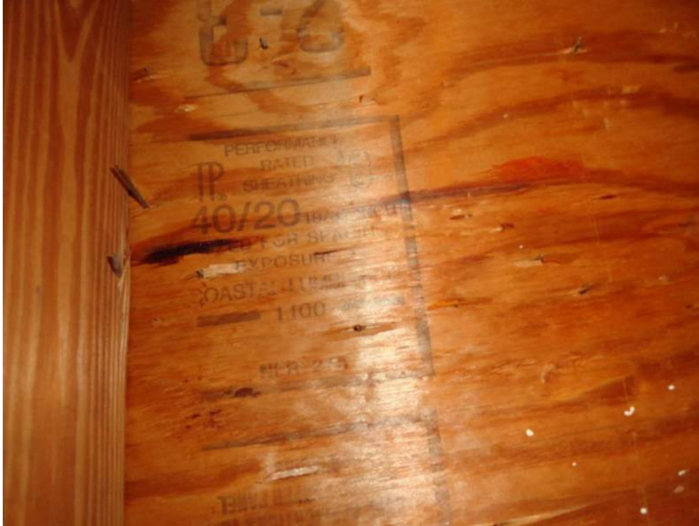
3. Roof Deck Attachment – 19/32" Plywood
