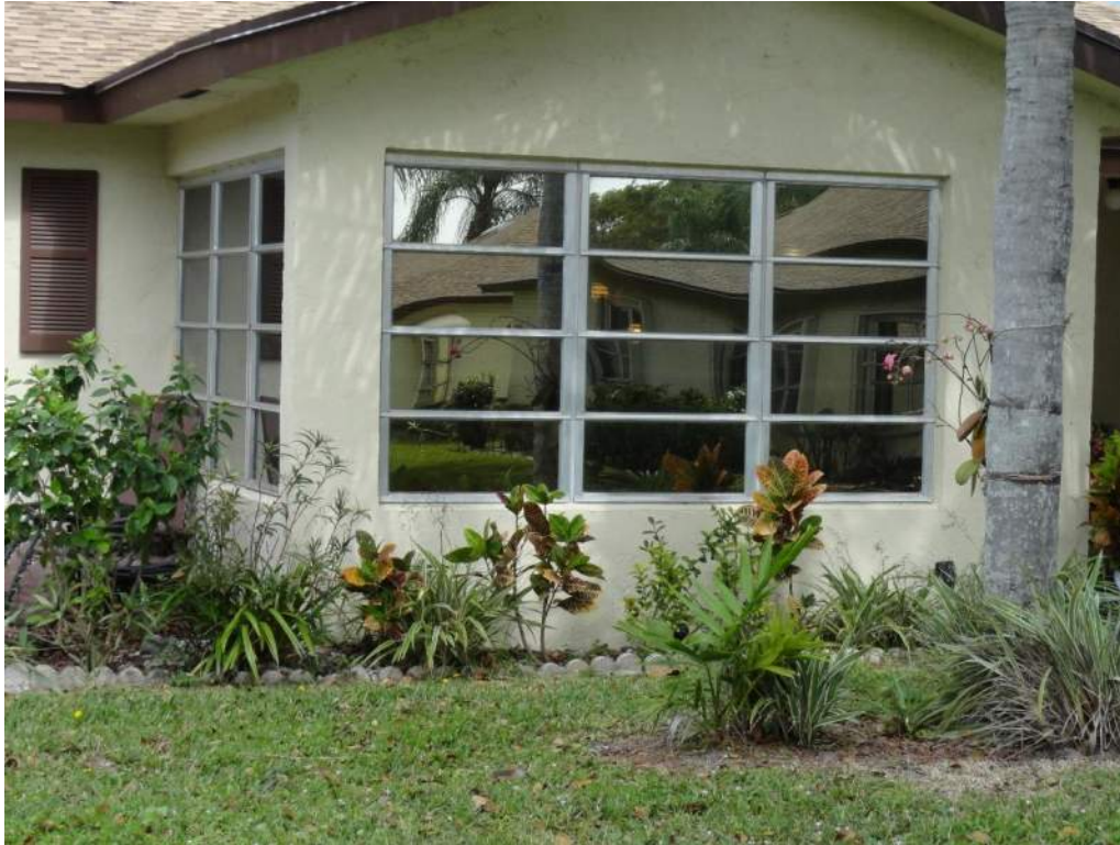
7. Opening Protection – Unrated Unprotected Windows
