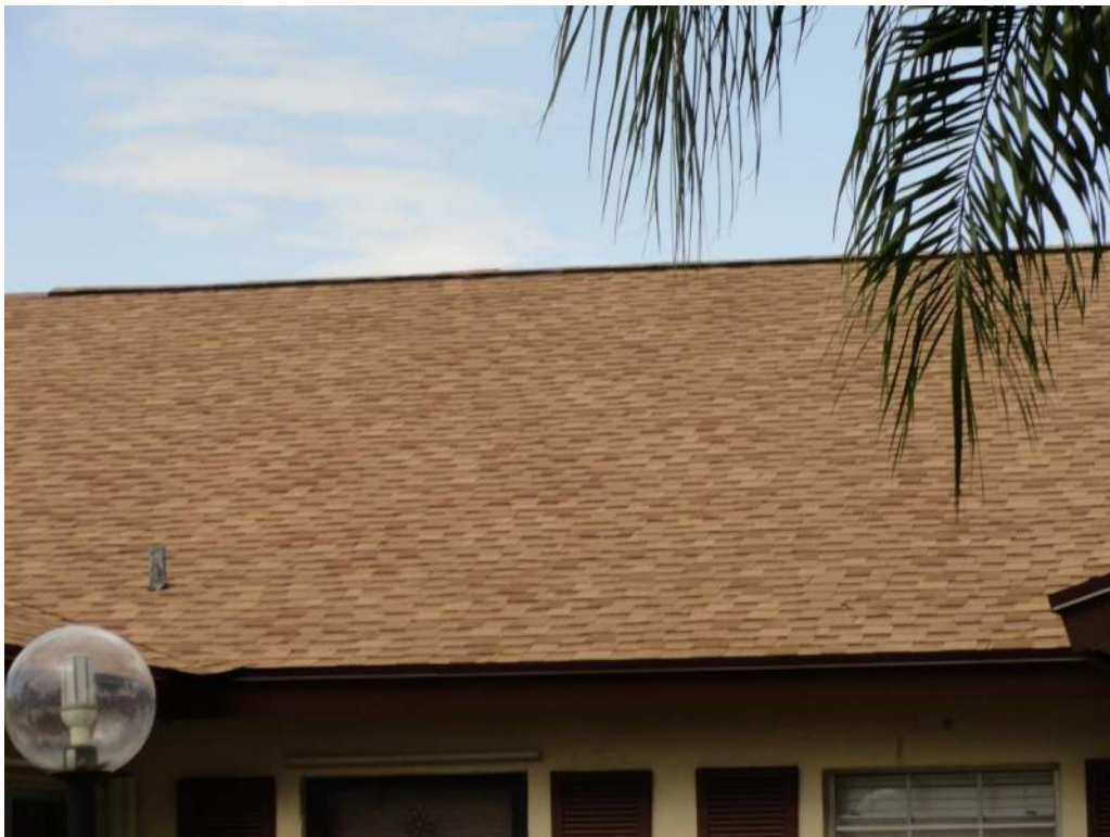
2. Roof Covering – Asphalt Shingles
