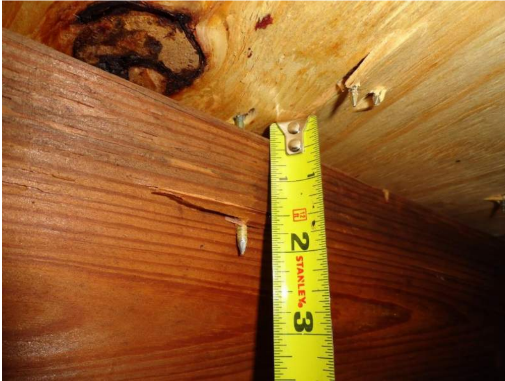
3. Roof Deck Attachment – 8d Nails
