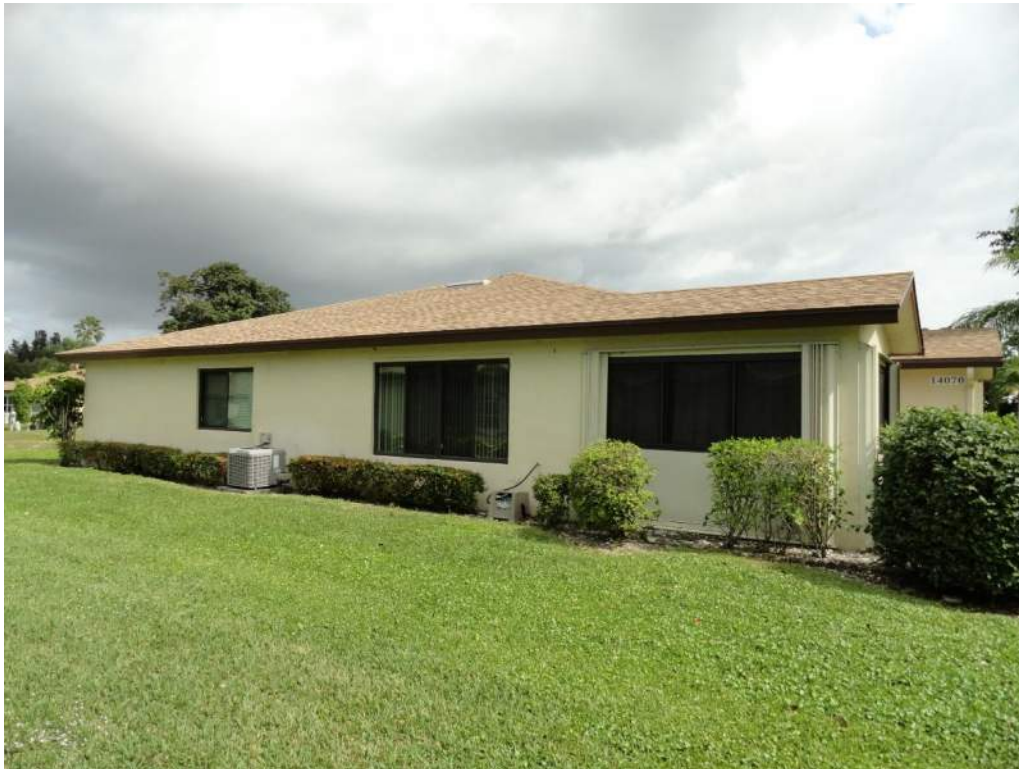
5. Roof Geometry – Left Elevation – Hip
