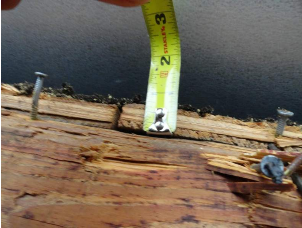
3. Roof Deck Attachment – 19/32" Plywood
