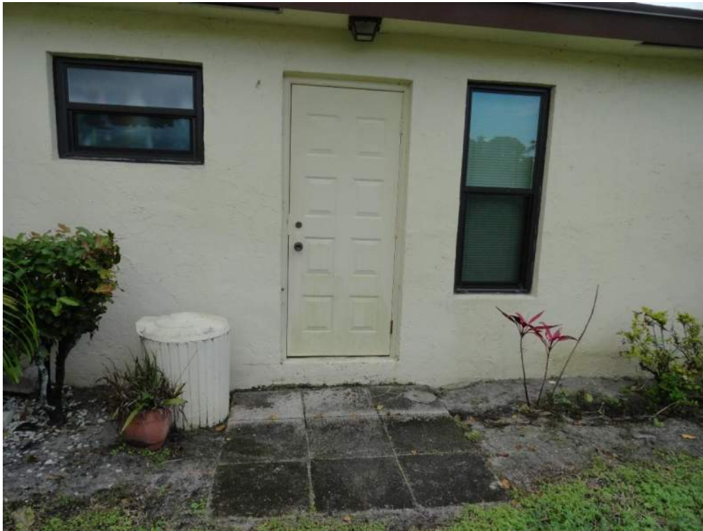
7. Opening Protection – Unprotected Unrated Unglazed Entry Door
