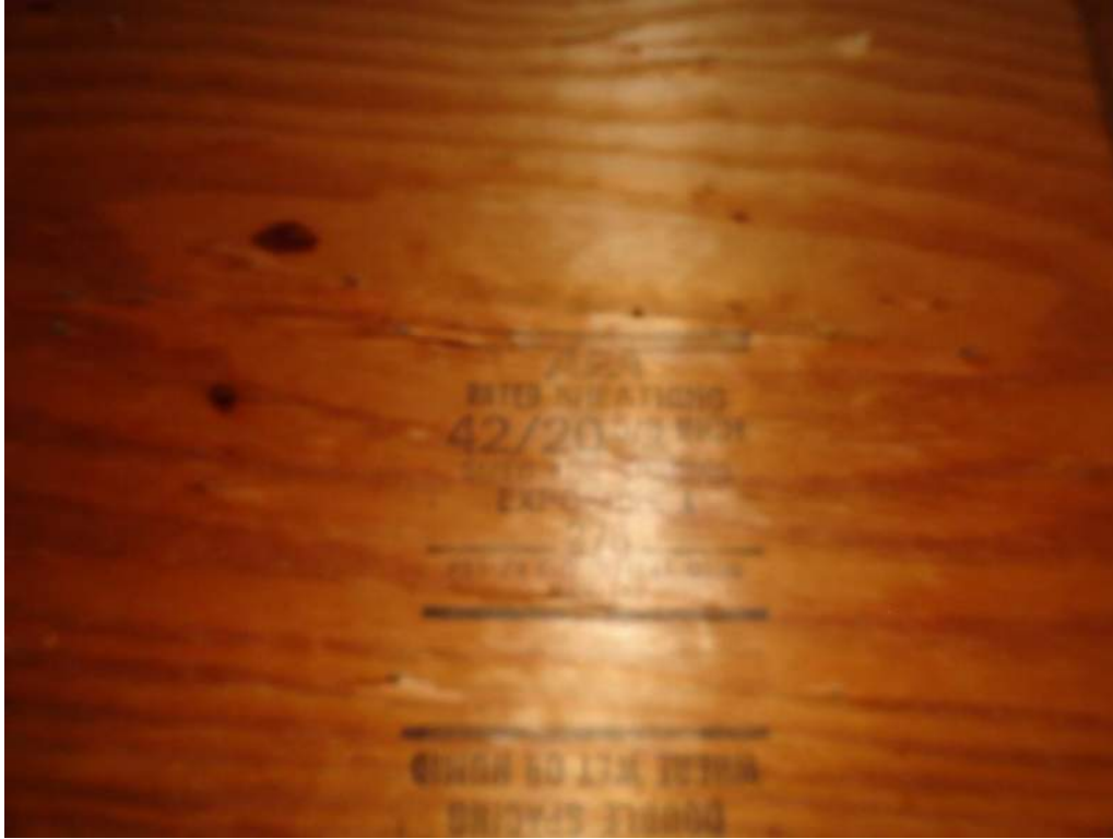
3. Roof Deck Attachment – 19/32" Plywood
