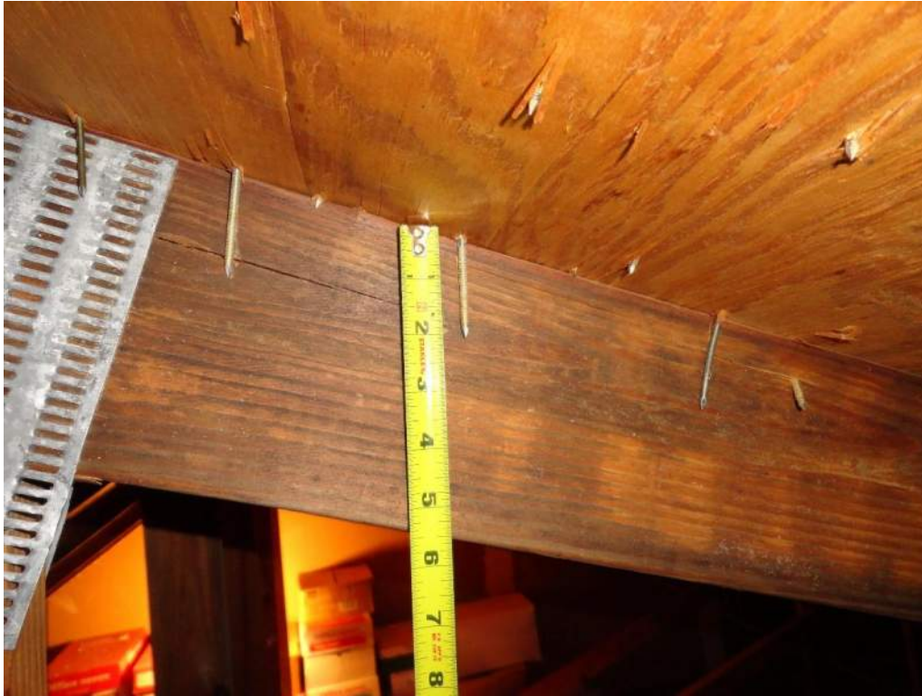
3. Roof Deck Attachment – 8d Nails
