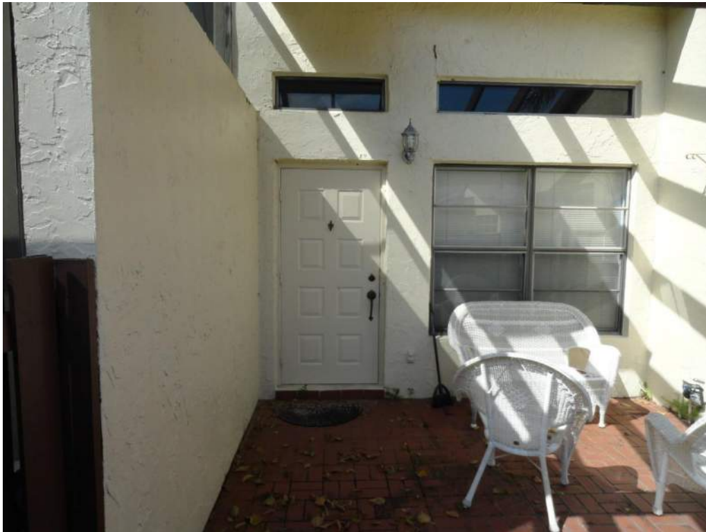
7. Opening Protection – Unprotected Unrated Unglazed Entry Door
