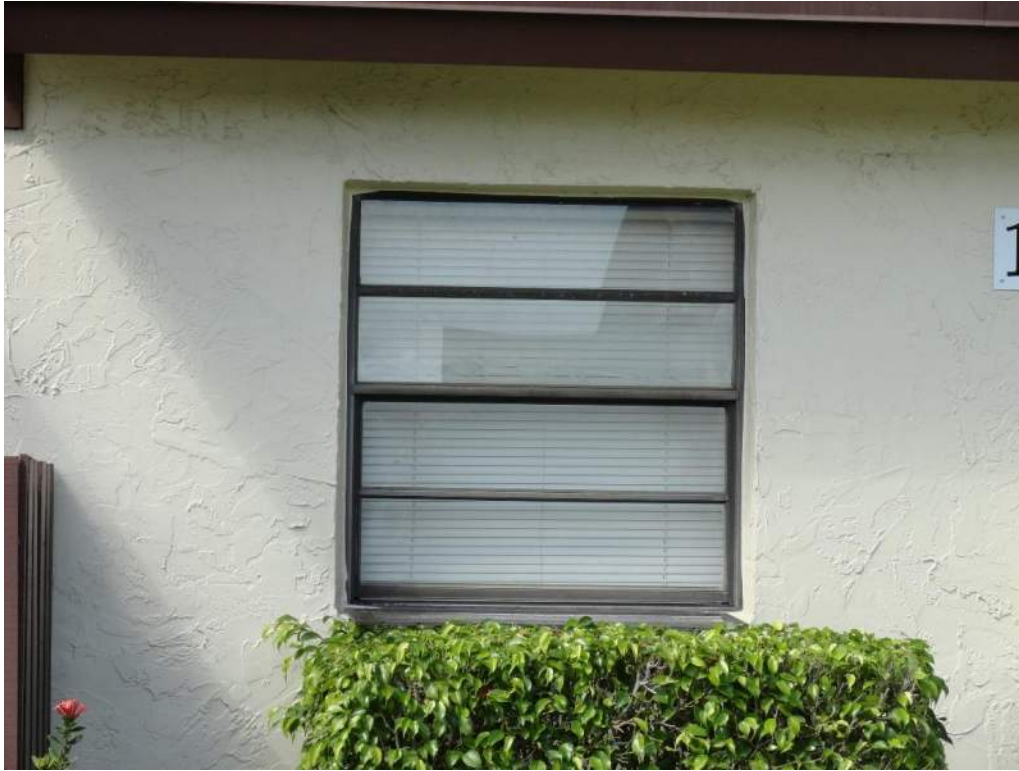
7. Opening Protection – Unrated Unprotected Windows
