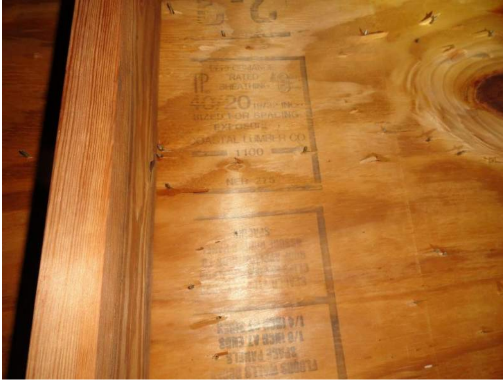
3. Roof Deck Attachment – 19/32" Plywood
