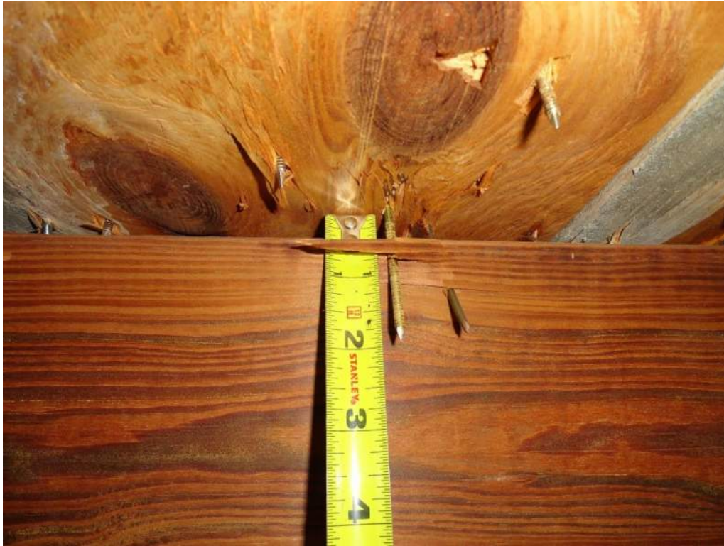
3. Roof Deck Attachment – 8d Nails
