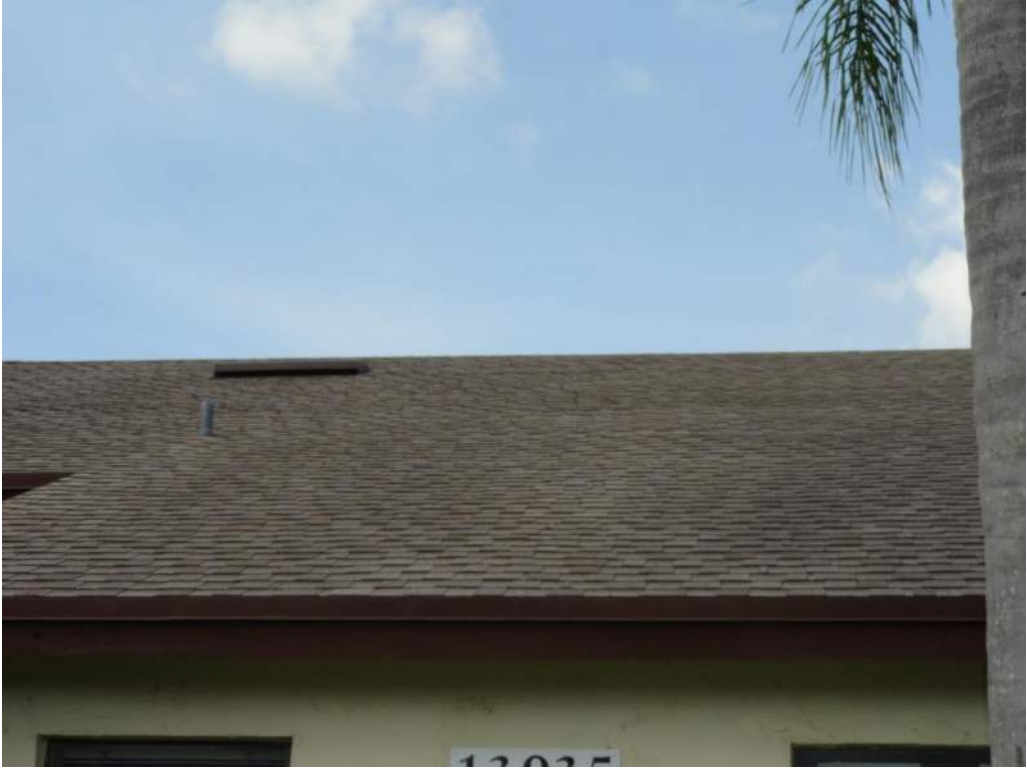
2. Roof Covering – Asphalt Shingles
