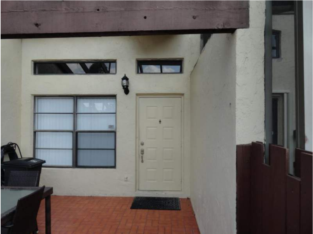
7. Opening Protection – Unprotected Unrated Unglazed Entry Door
