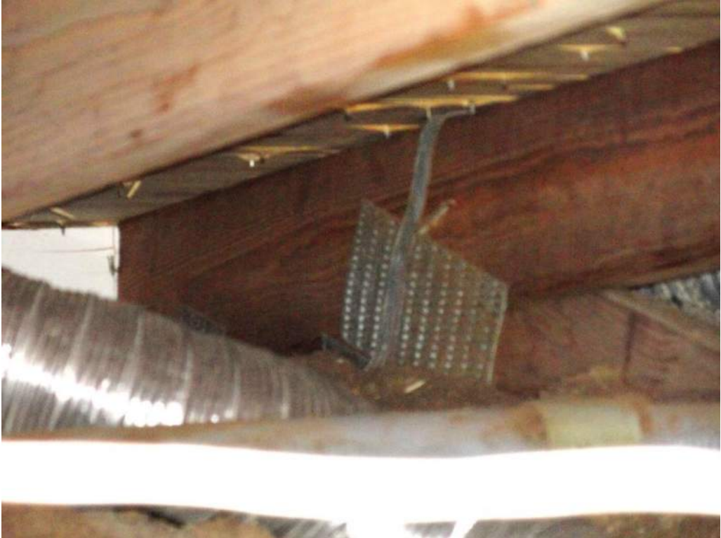
4. Roof to Wall Attachment – Single Wraps – Steel Straps w/ 2 Nails Min. at Face
