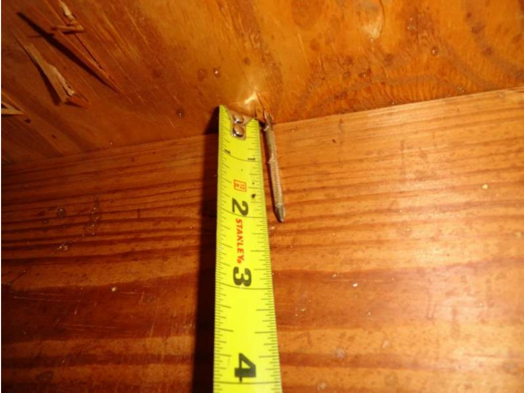
3. Roof Deck Attachment – 8d Nails
