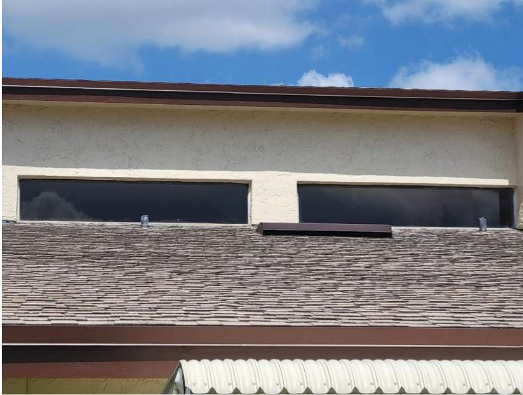
7. Opening Protection – Unrated Unprotected Windows
