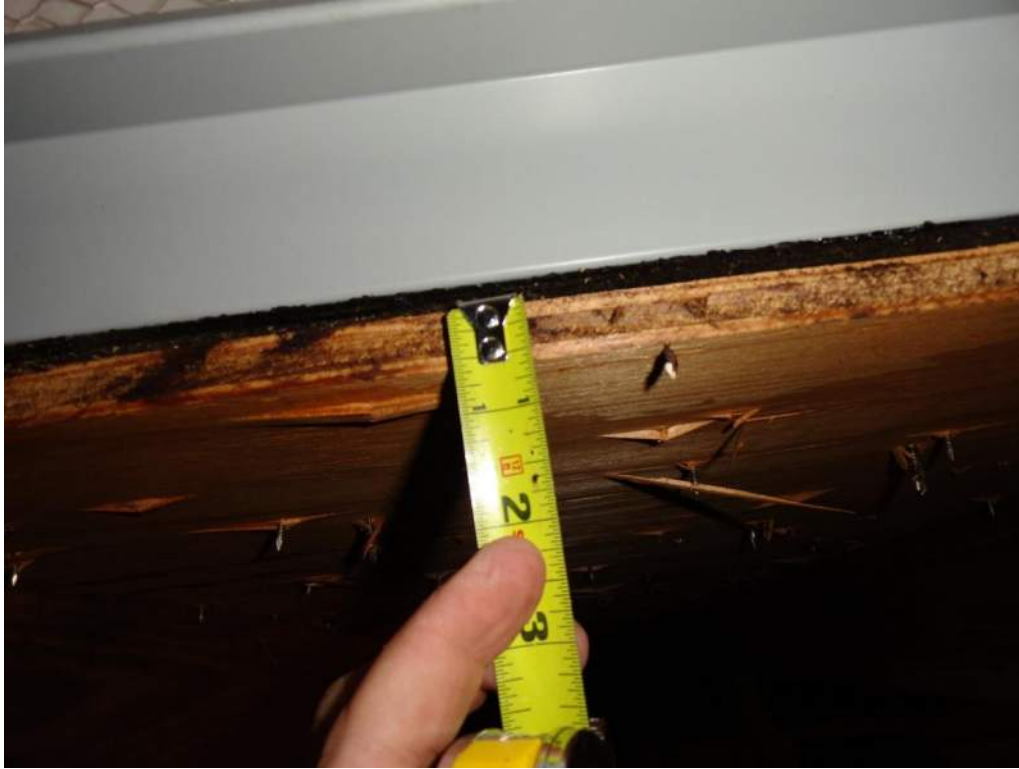
3. Roof Deck Attachment – 5/8" Plywood
