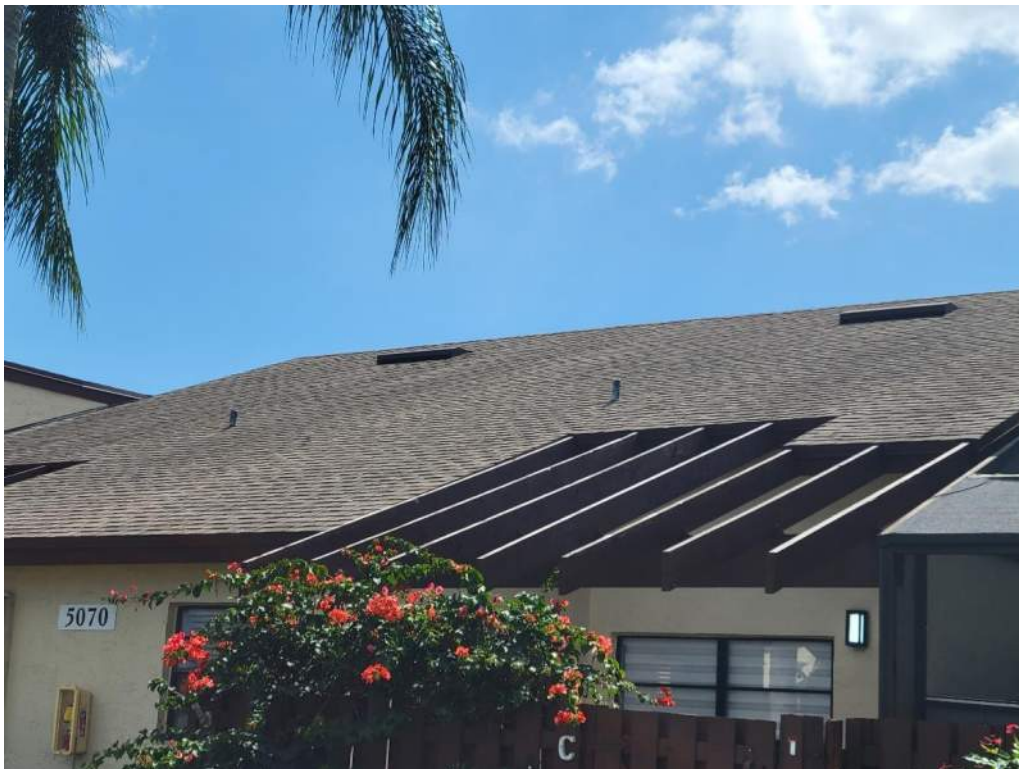
2. Roof Covering – Asphalt Shingles
