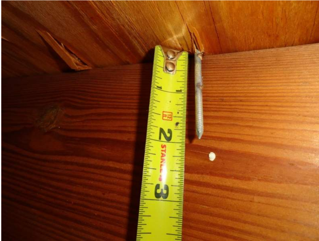
3. Roof Deck Attachment – 8d Nails
