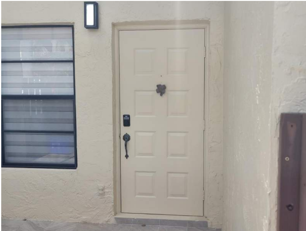
7. Opening Protection – Unprotected Unrated Unglazed Entry Door
