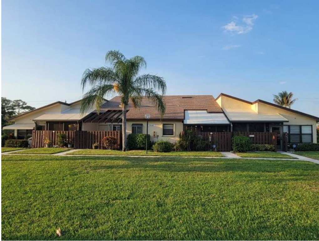
5. Roof Geometry – Front Elevation – Non-Hip
