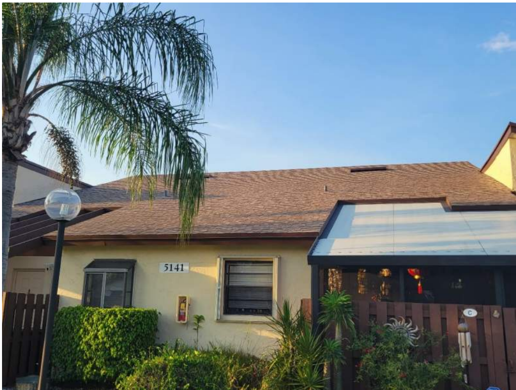
2. Roof Covering – Asphalt Shingles
