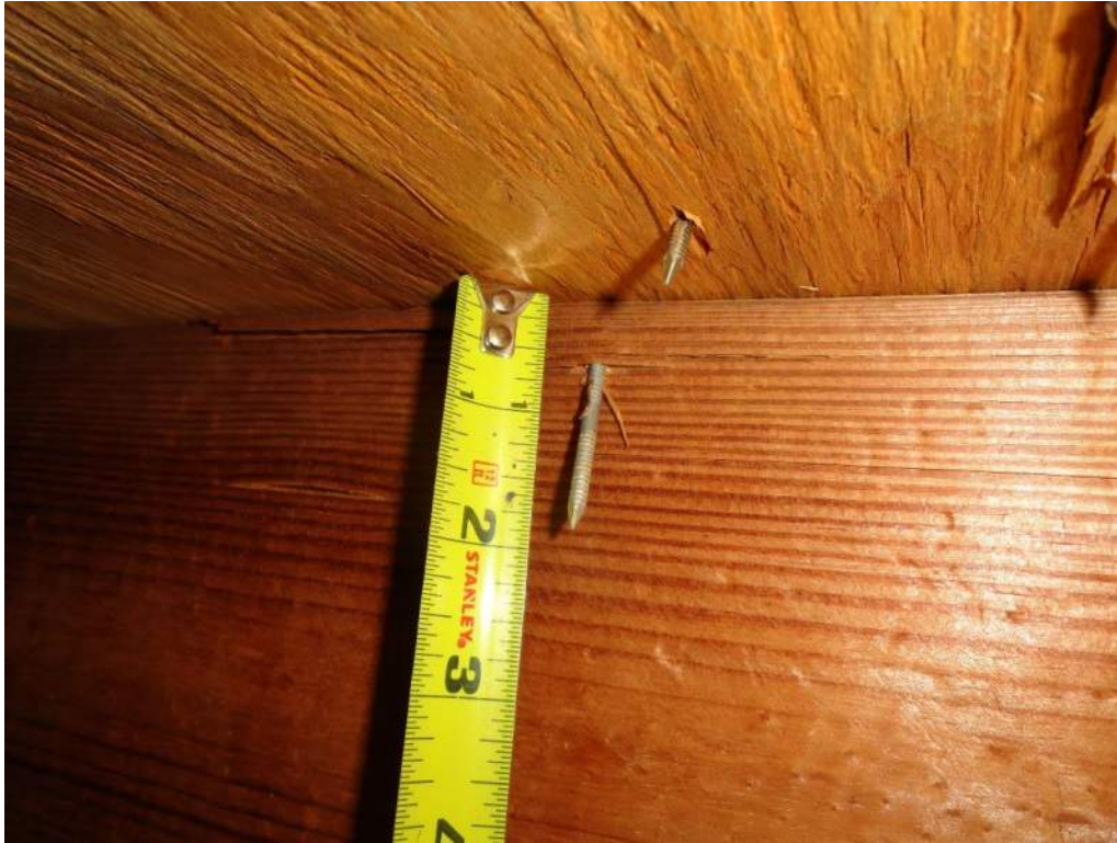
3. Roof Deck Attachment – 8d Nails
