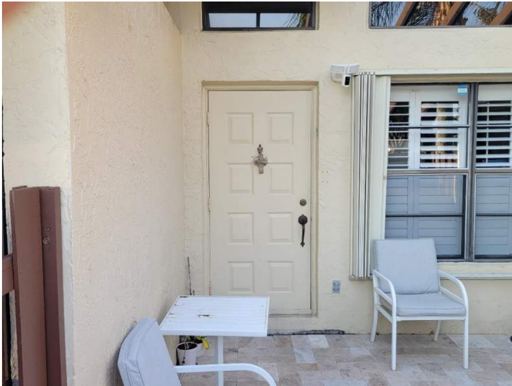
7. Opening Protection – Unprotected Unrated Unglazed Entry Door
