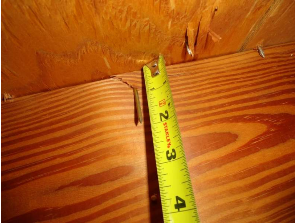
3. Roof Deck Attachment – 8d Nails
