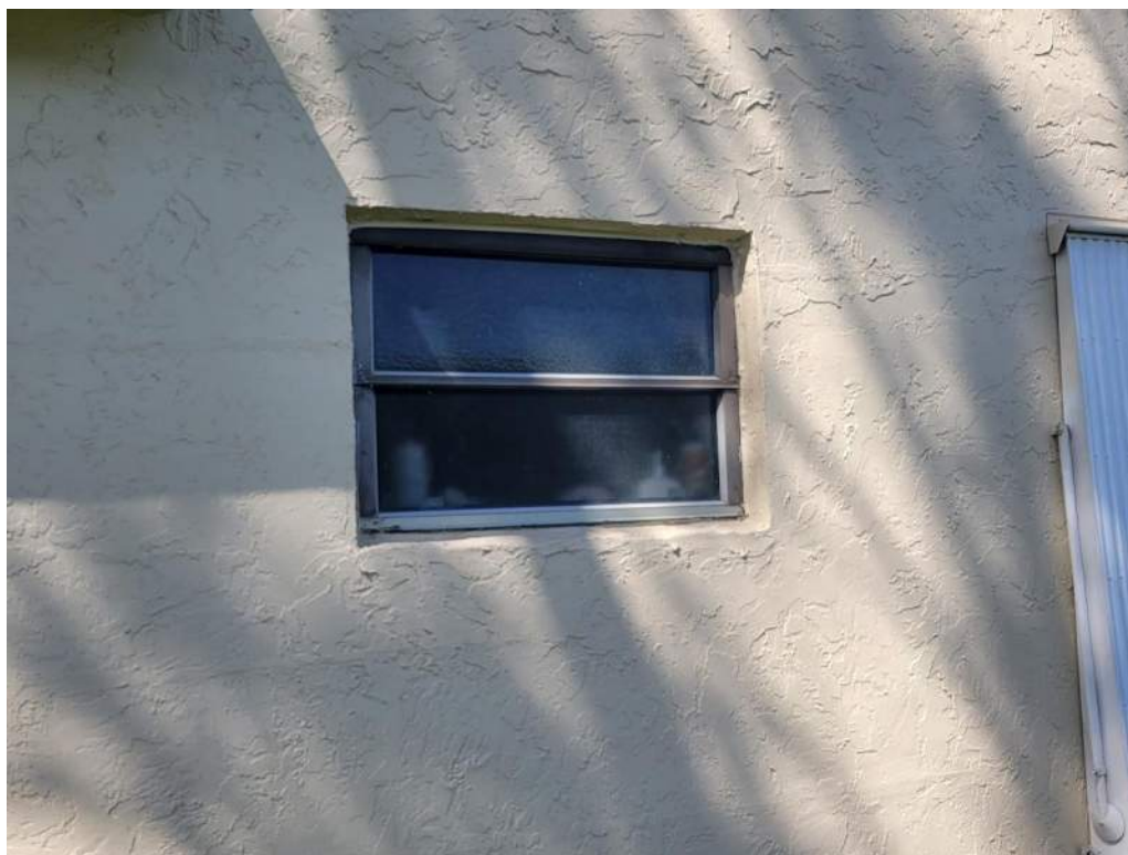
7. Opening Protection – Unprotected Unrated Windows
