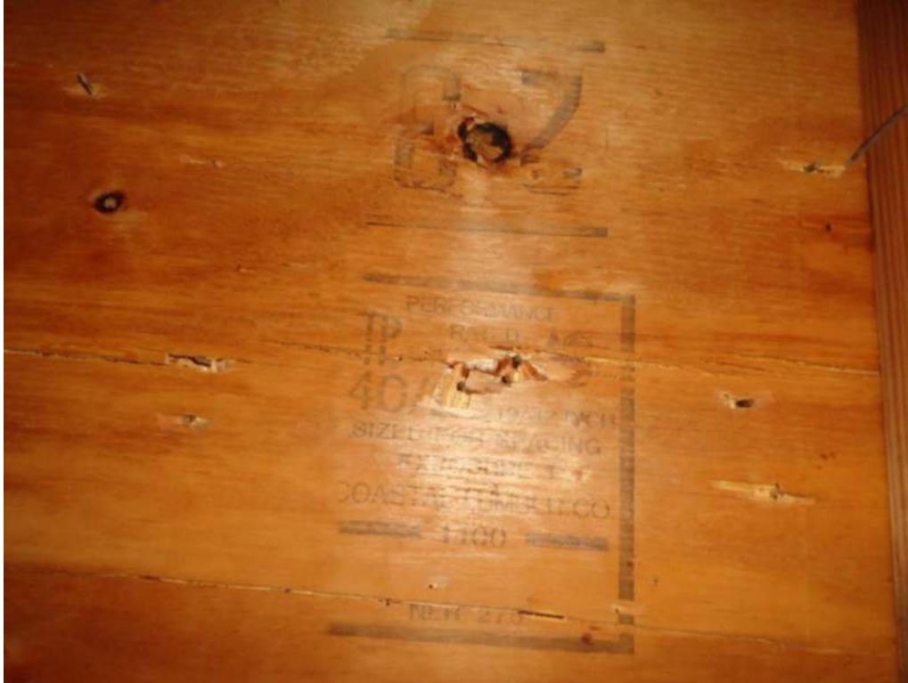
3. Roof Deck Attachment – 19/32" Plywood
