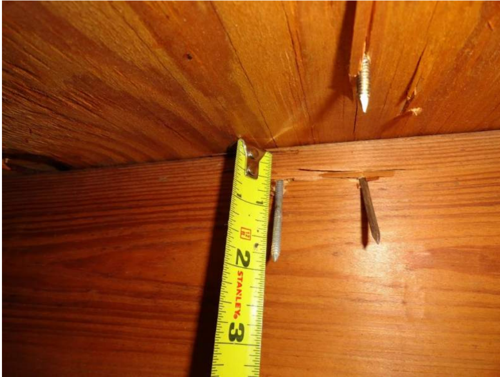
3. Roof Deck Attachment – 8d Nails
