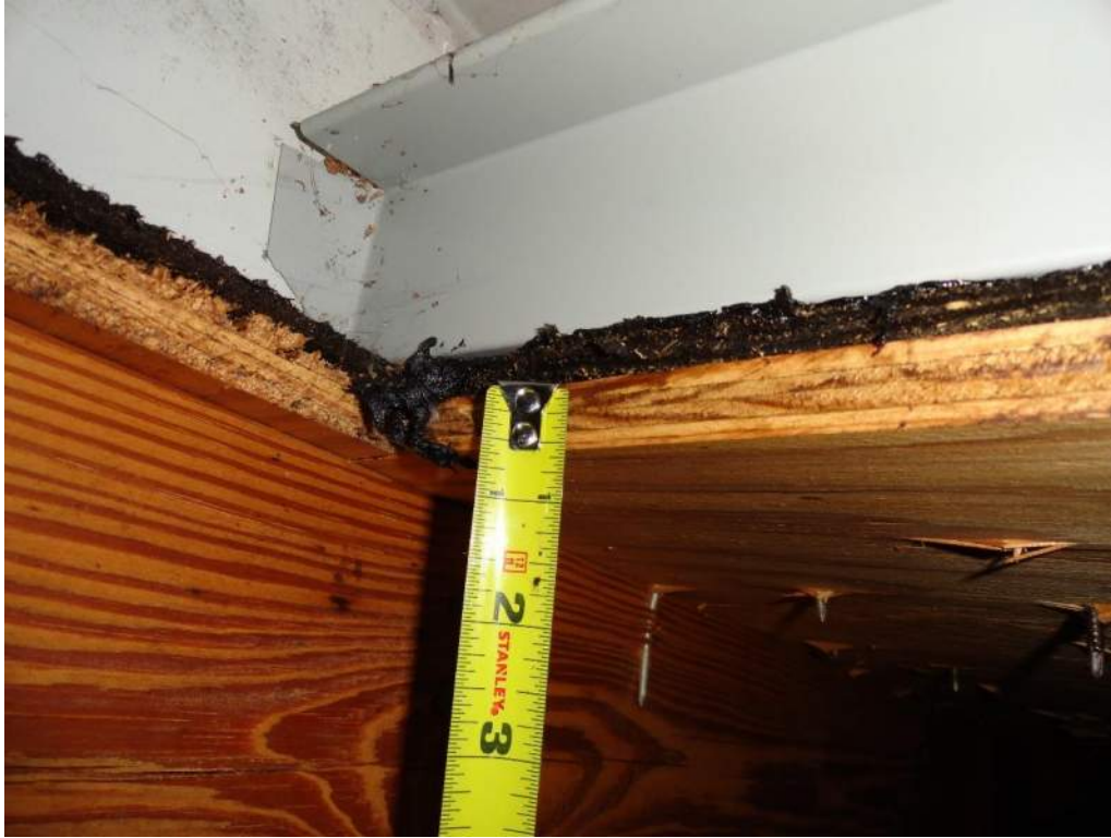
3. Roof Deck Attachment – 5/8" Plywood
