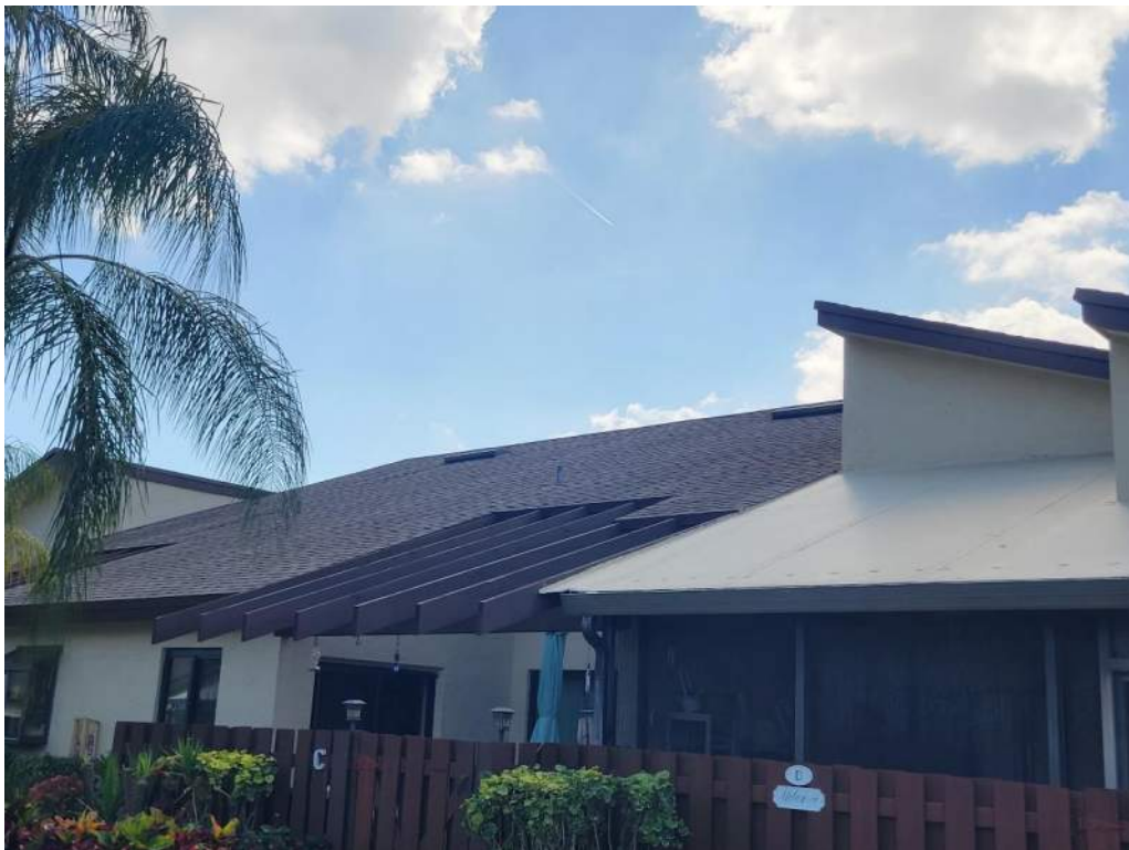
2. Roof Covering – Asphalt Shingles
