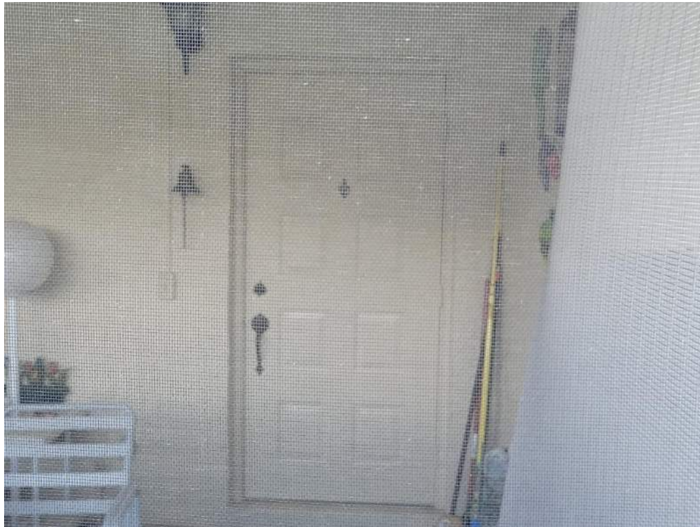
7. Opening Protection – Unprotected Unrated Unglazed Entry Door
