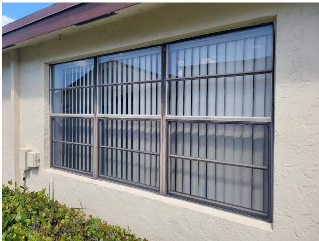
7. Opening Protection – Unrated Unprotected Windows
