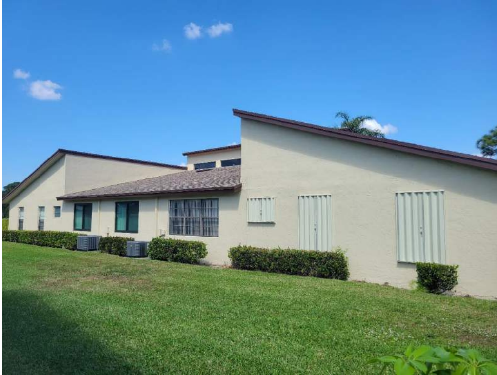
5. Roof Geometry – Rear Elevation – Non-Hip
