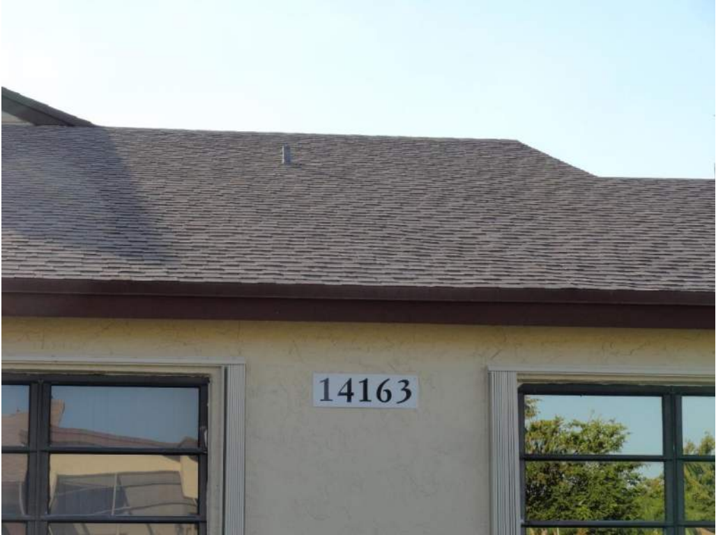
2. Roof Covering – Asphalt Shingles
