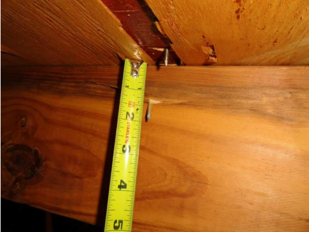
3. Roof Deck Attachment – 8d Nails
