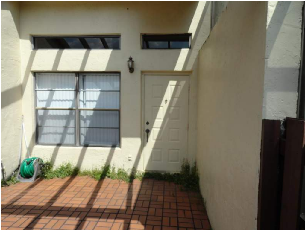
7. Opening Protection – Unprotected Unrated Unglazed Entry Door
