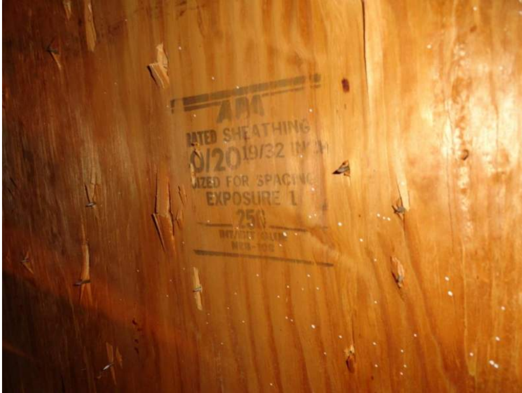
3. Roof Deck Attachment – 19/32" Plywood
