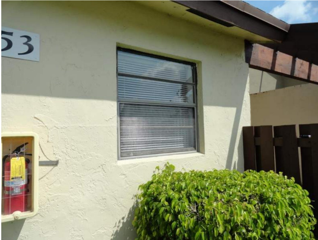
7. Opening Protection – Unrated Unprotected Windows
