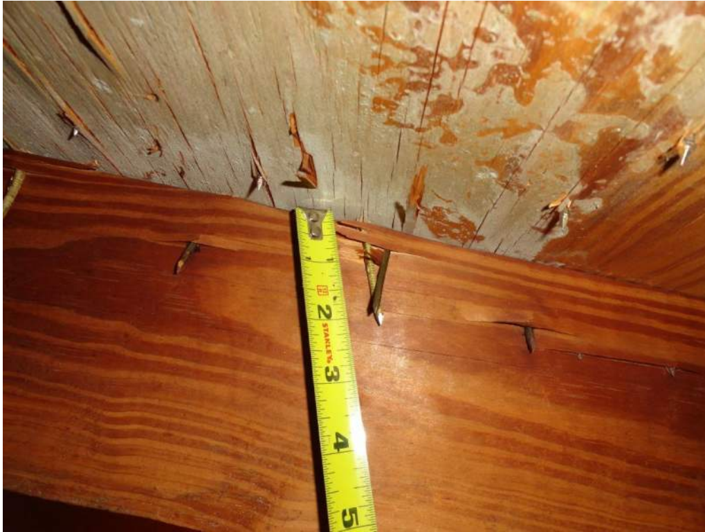
3. Roof Deck Attachment – 8d Nails
