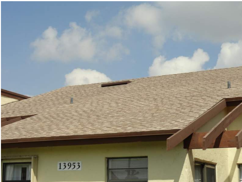
2. Roof Covering – Asphalt Shingles
