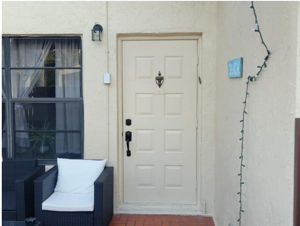
7. Opening Protection – Unprotected Unrated Unglazed Entry Door
