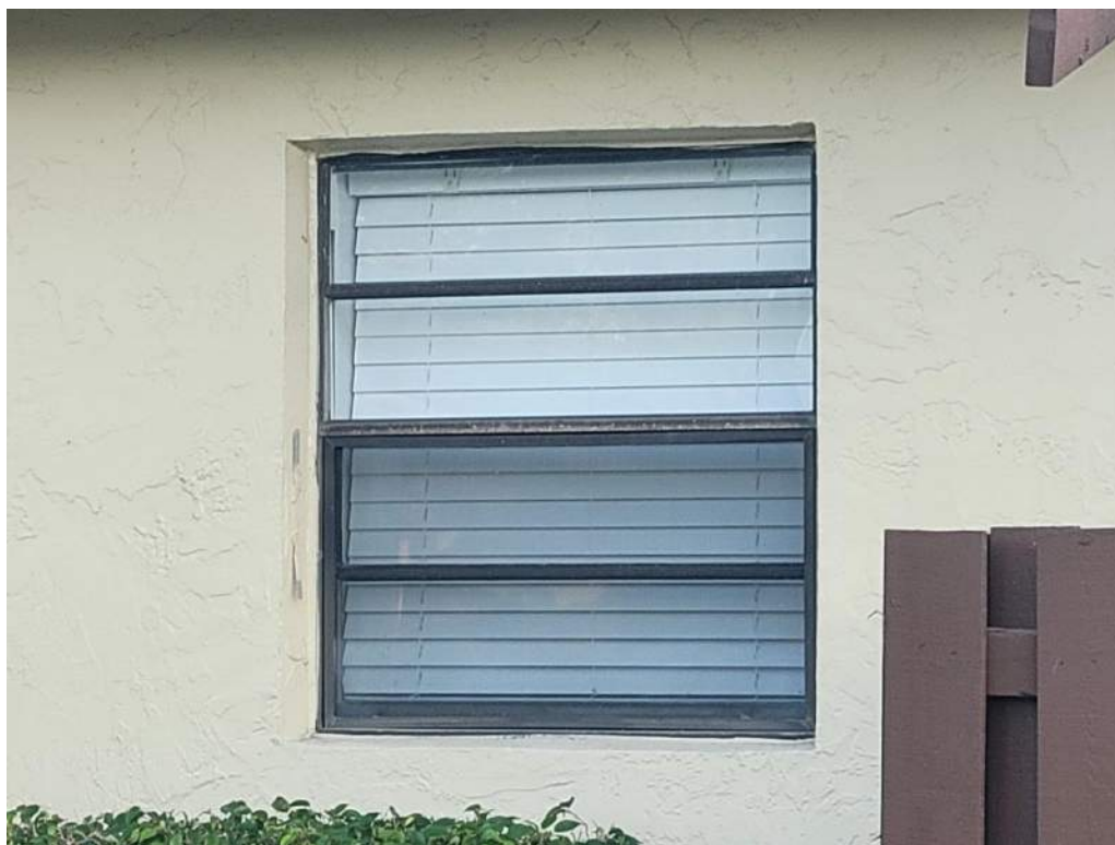
7. Opening Protection – Unrated Unprotected Windows
