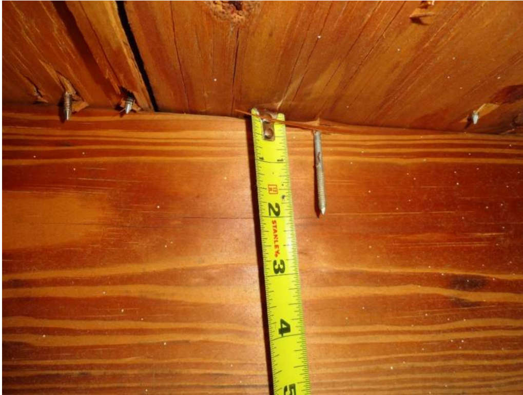
3. Roof Deck Attachment – 8d Nails
