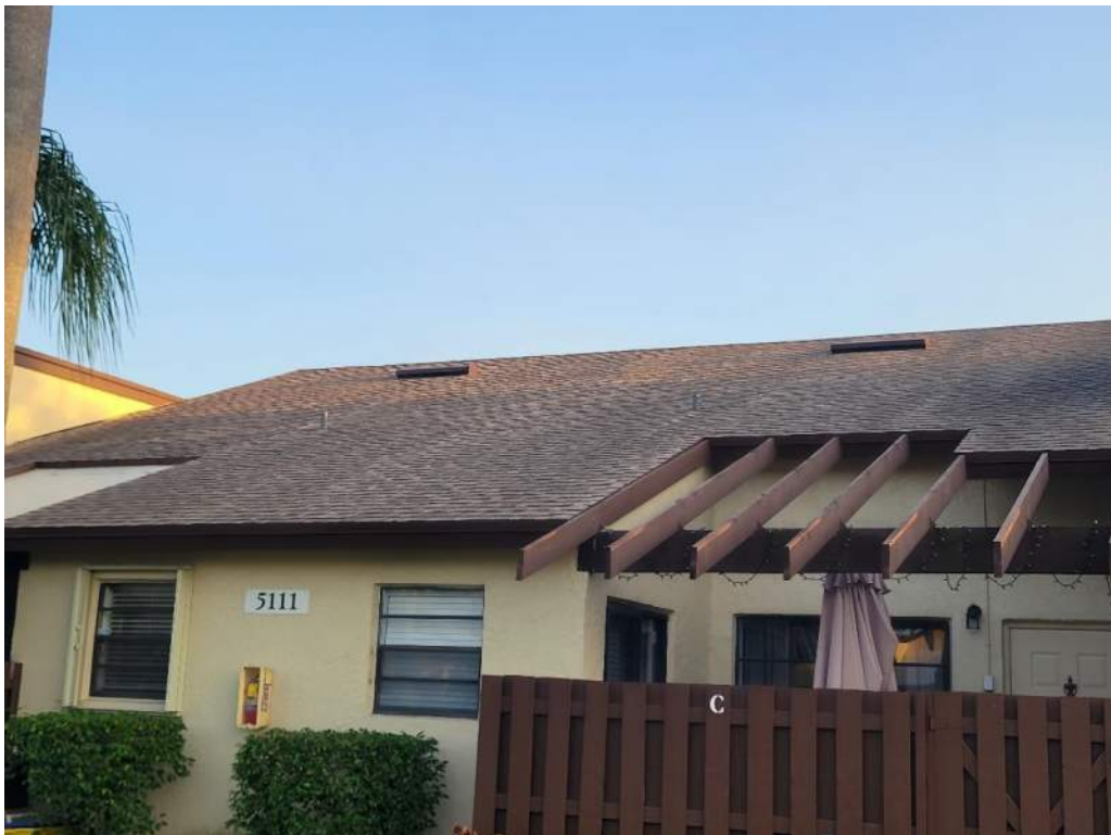
2. Roof Covering – Asphalt Shingles
