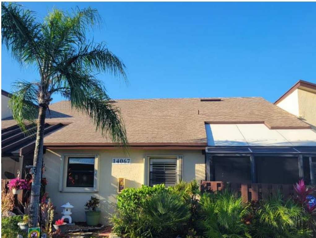
2. Roof Covering – Asphalt Shingles
