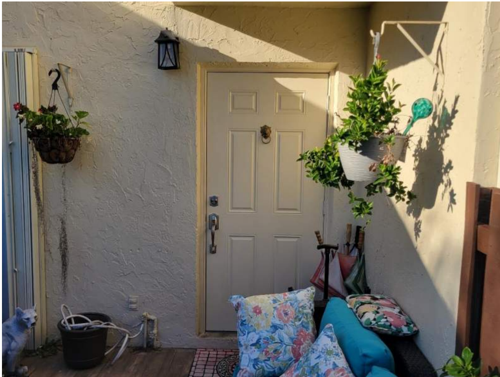
7. Opening Protection – Unprotected Unrated Unglazed Entry Door
