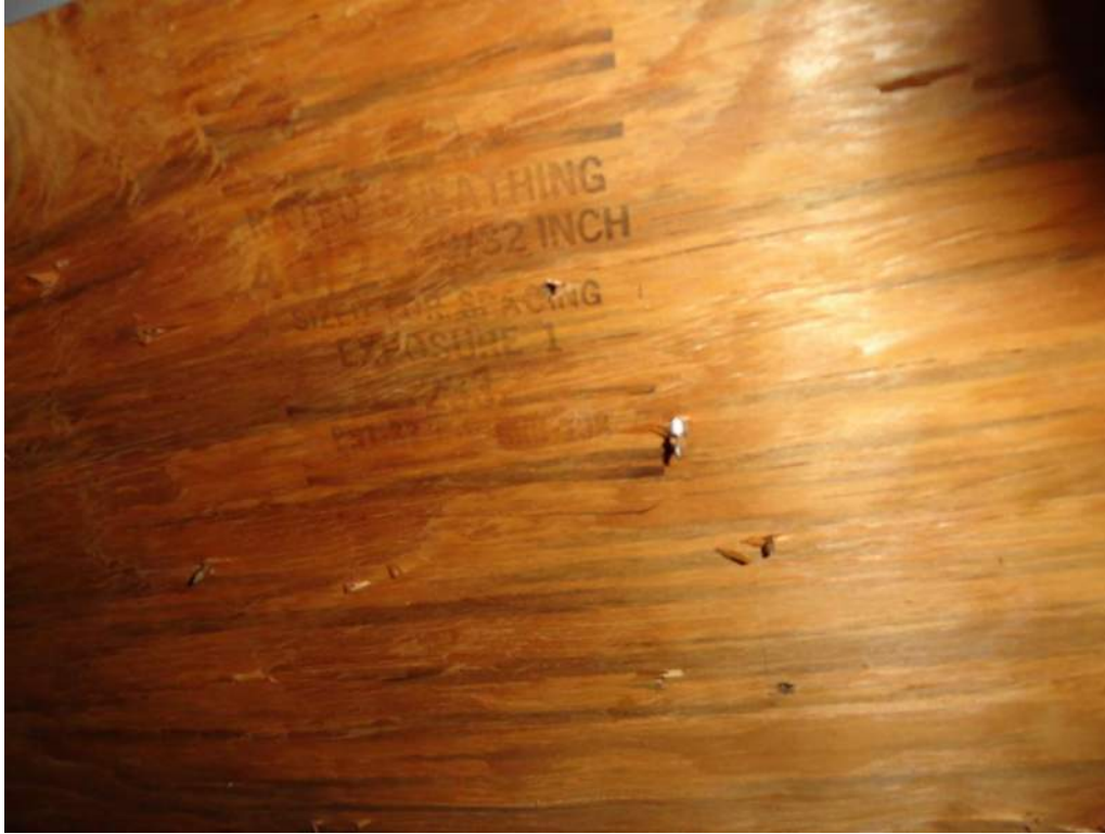
3. Roof Deck Attachment – 19/32" Plywood
