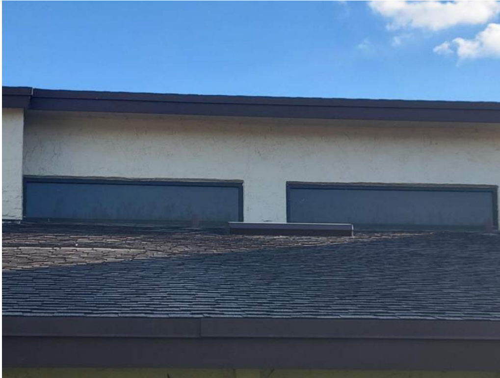
7. Opening Protection – Unprotected Unrated Windows
