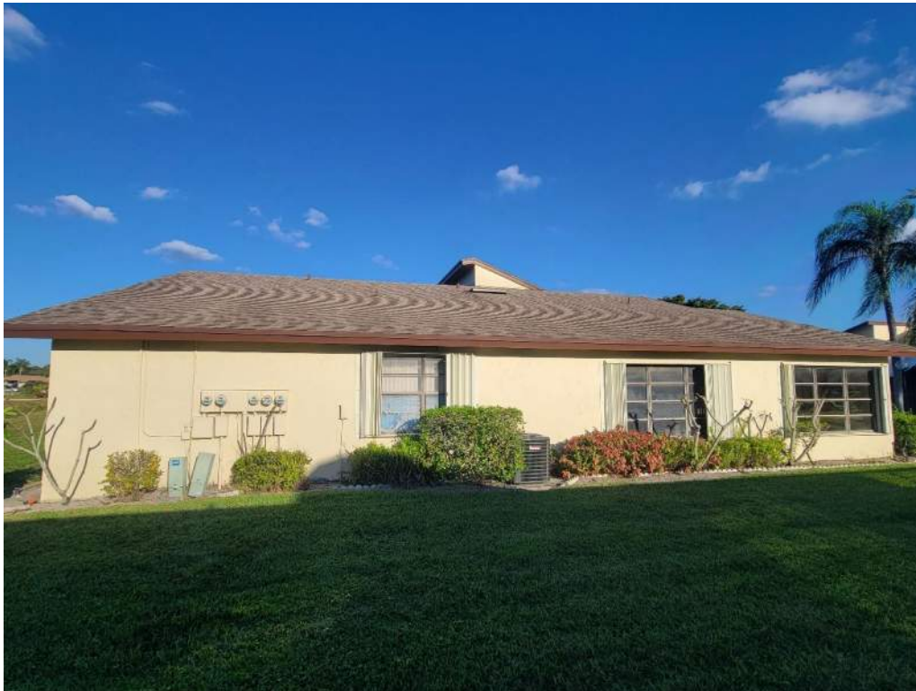
5. Roof Geometry – Right Elevation – Non-Hip
