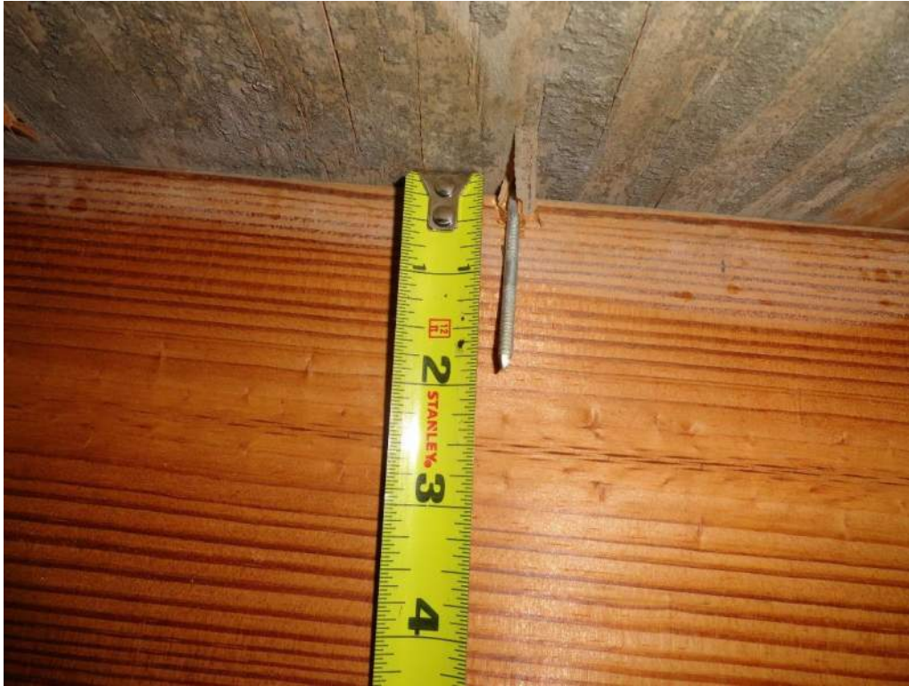
3. Roof Deck Attachment – 8d Nails
