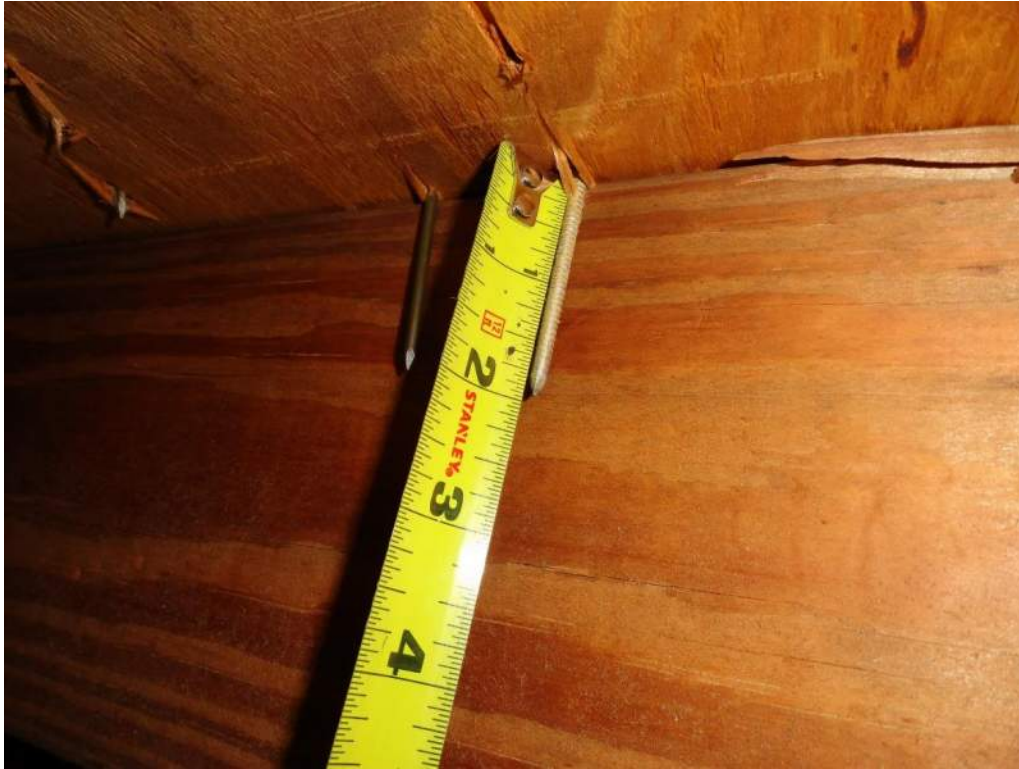
3. Roof Deck Attachment – 8d Nails
