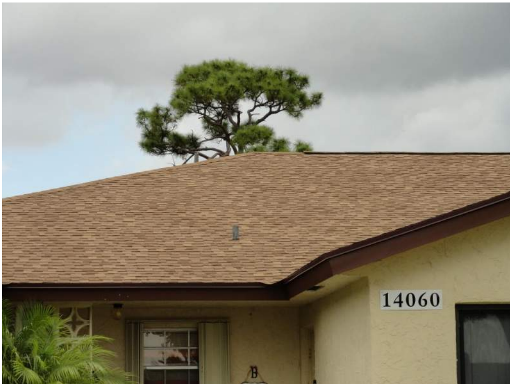
2. Roof Covering – Asphalt Shingles
