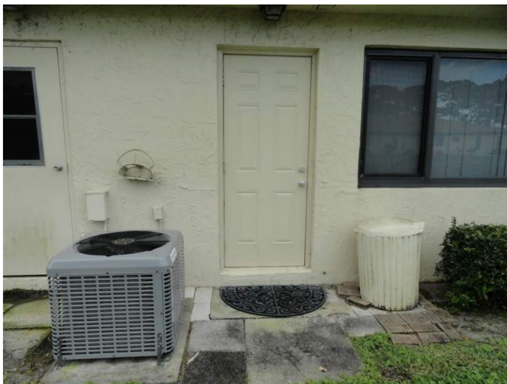
7. Opening Protection – Unprotected Unrated Unglazed Entry Door
