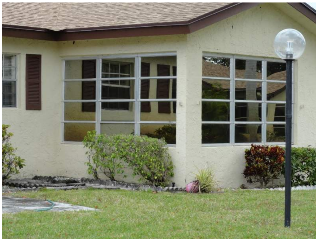
7. Opening Protection – Unrated Unprotected Windows
