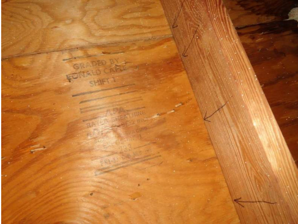
3. Roof Deck Attachment – 19/32" Plywood
