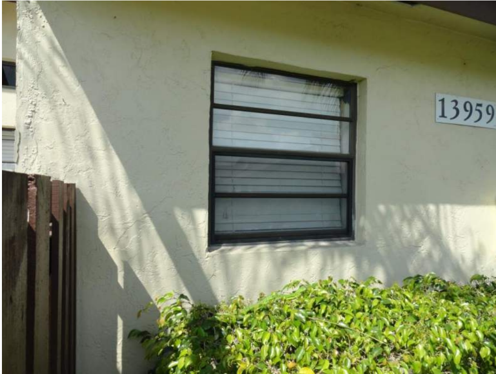
7. Opening Protection – Unrated Unprotected Windows
