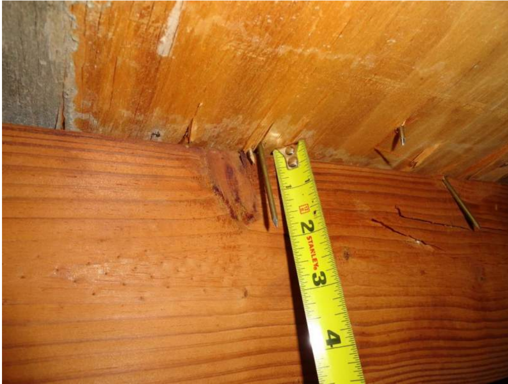
3. Roof Deck Attachment – 8d Nails
