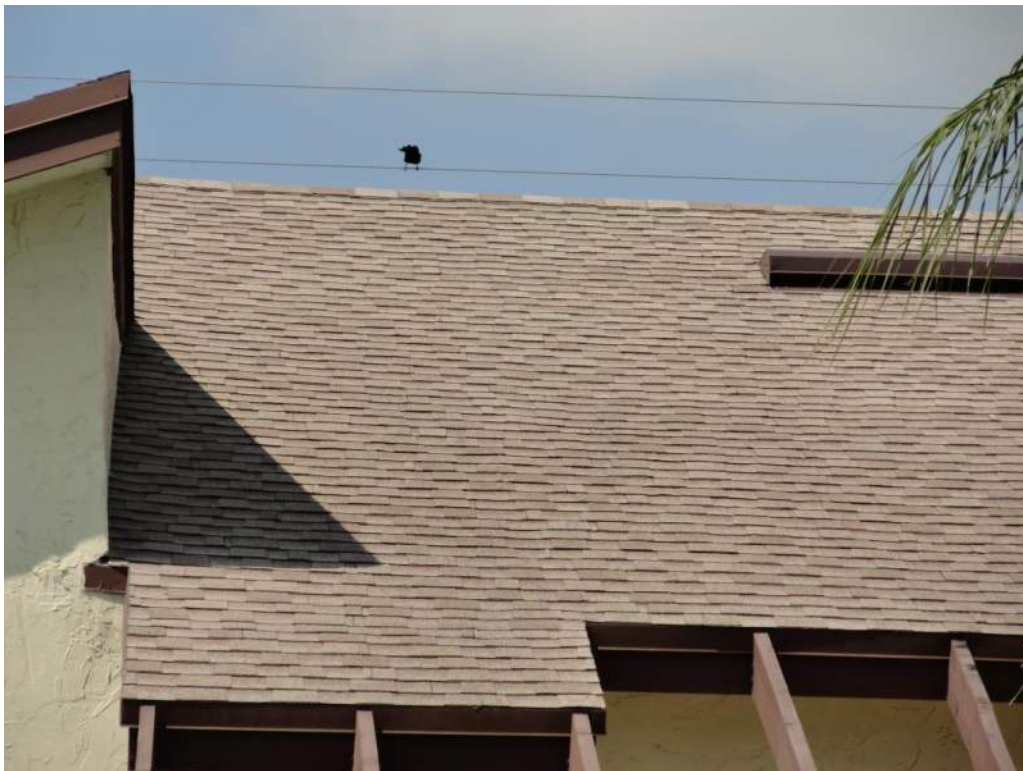
2. Roof Covering – Asphalt Shingles
