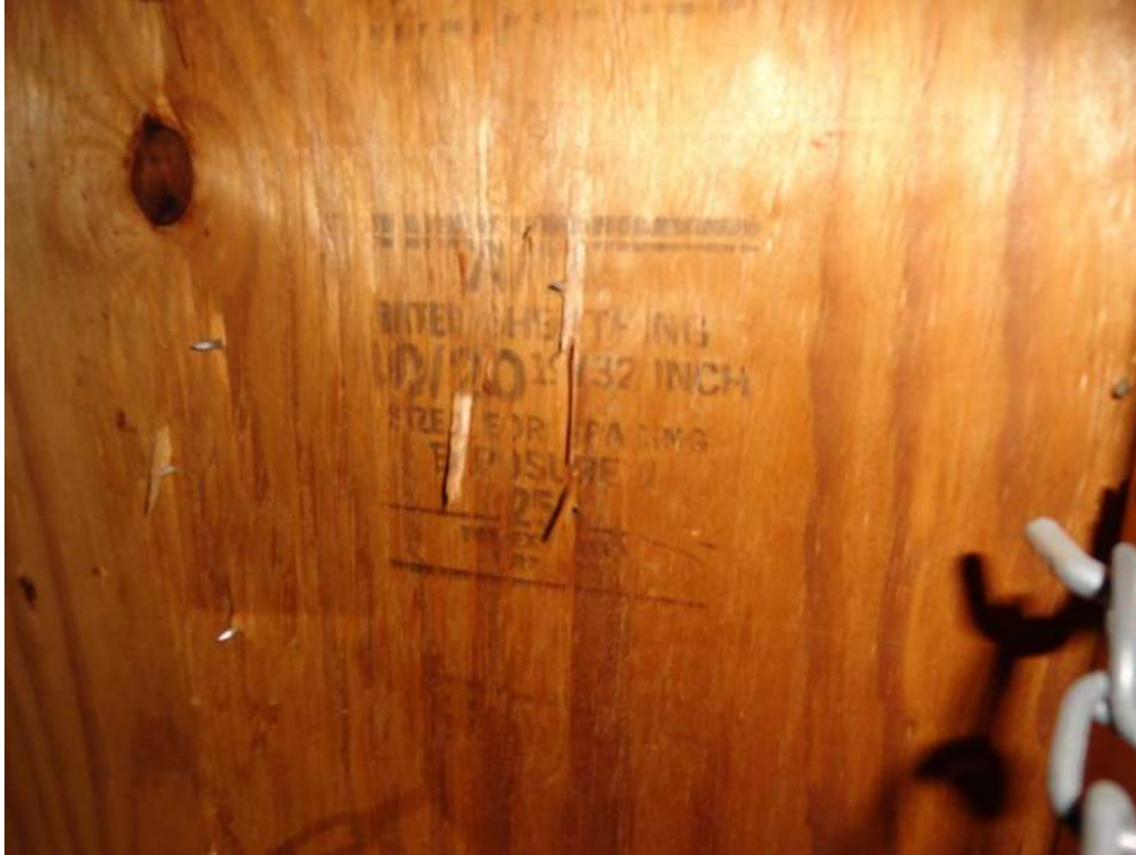
3. Roof Deck Attachment – 19/32" Plywood
