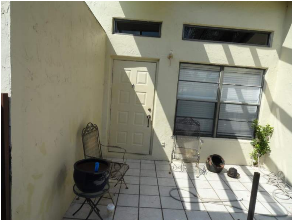
7. Opening Protection – Unprotected Unrated Unglazed Entry Door
