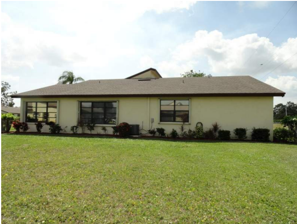
5. Roof Geometry – Right Elevation – Non-Hip
