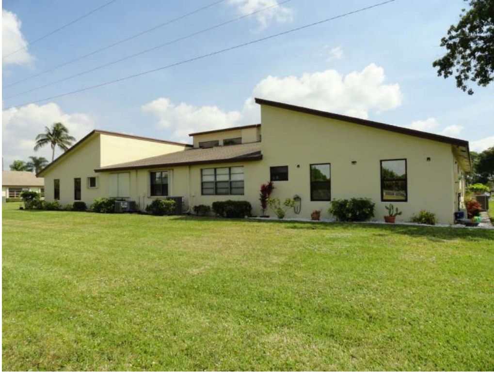
5. Roof Geometry – Rear Elevation – Non-Hip
