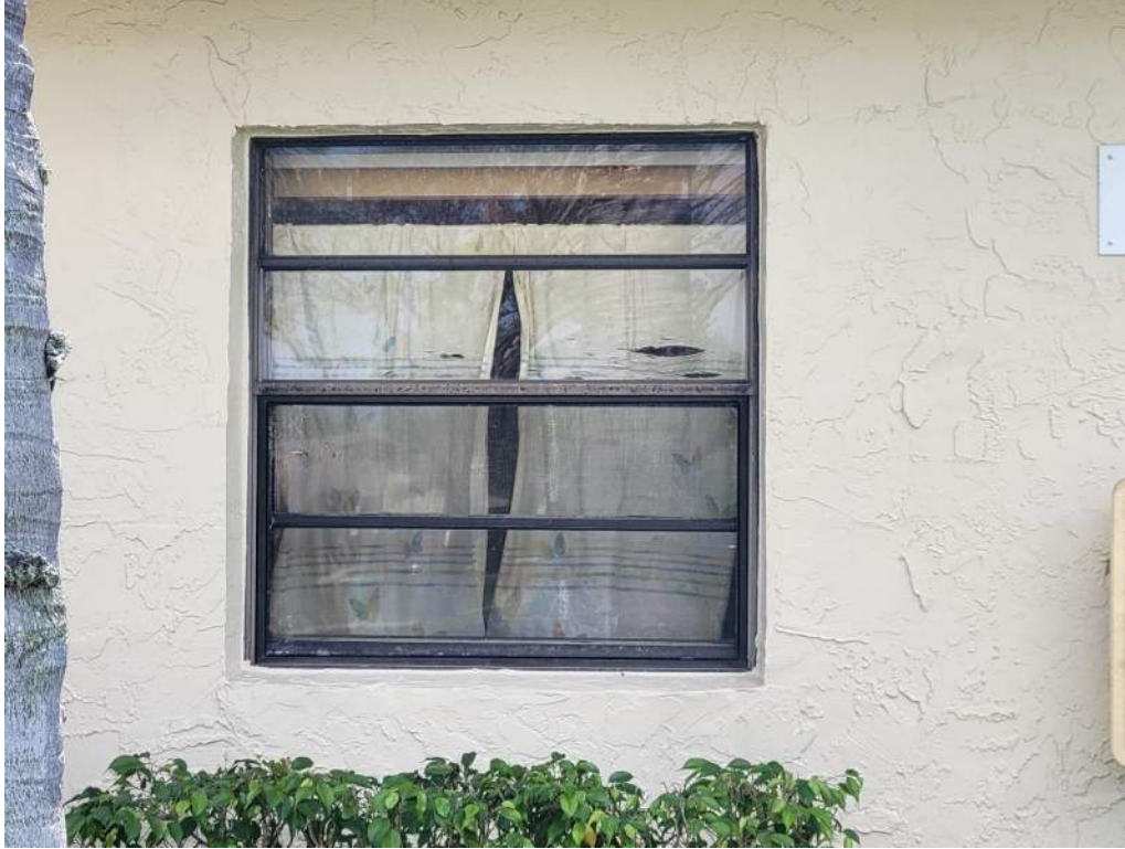
7. Opening Protection – Unrated Unprotected Windows
