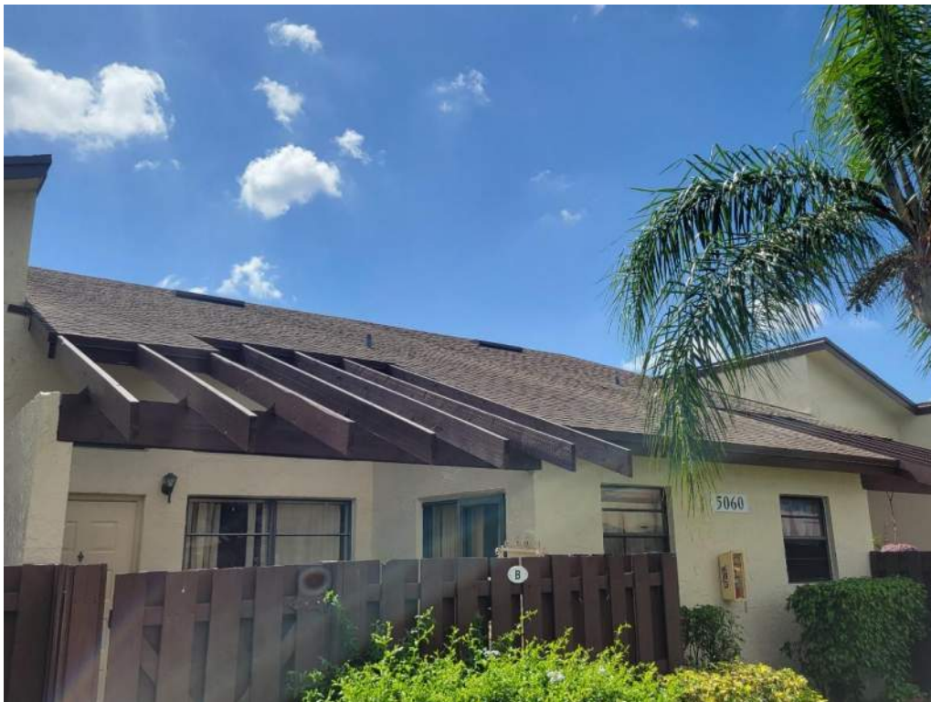
2. Roof Covering – Asphalt Shingles
