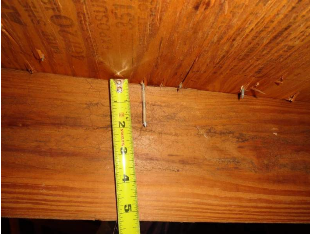
3. Roof Deck Attachment – 8d Nails
