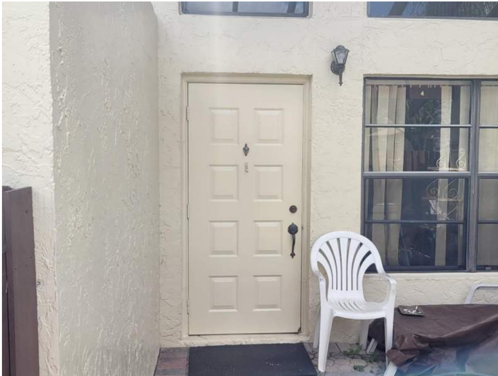
7. Opening Protection – Unprotected Unrated Unglazed Entry Door
