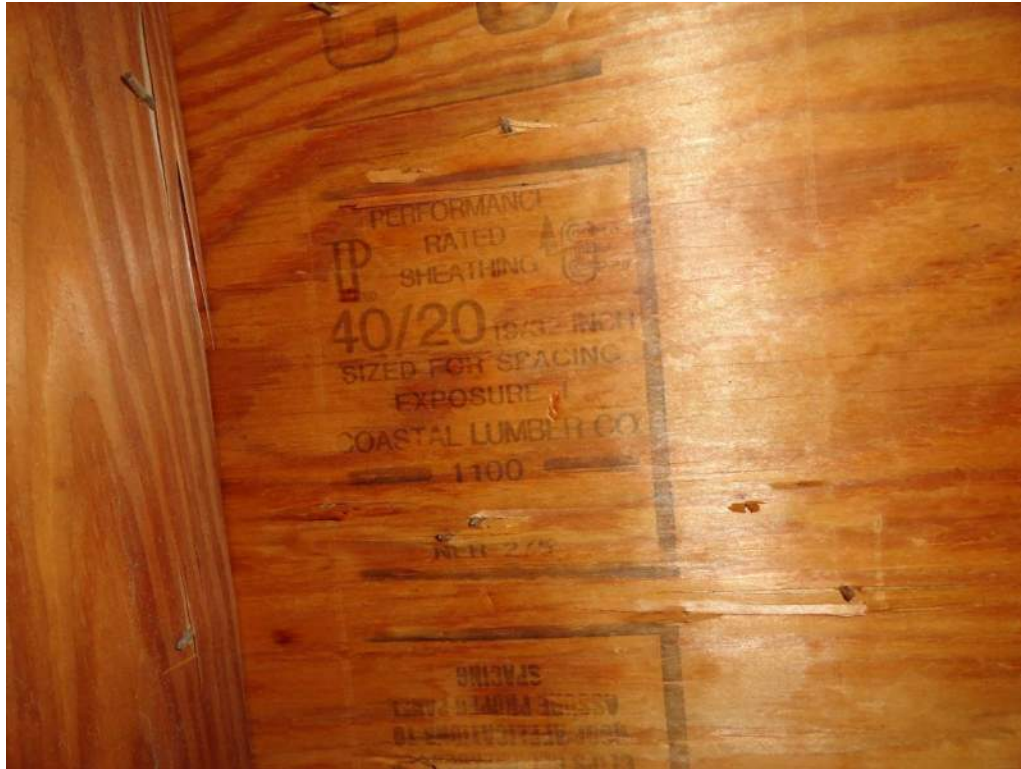
3. Roof Deck Attachment – 19/32" Plywood
