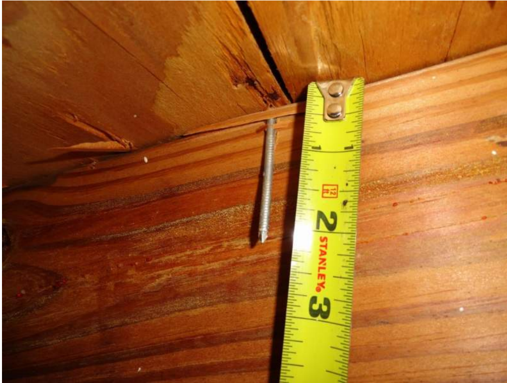
3. Roof Deck Attachment – 8d Nails
