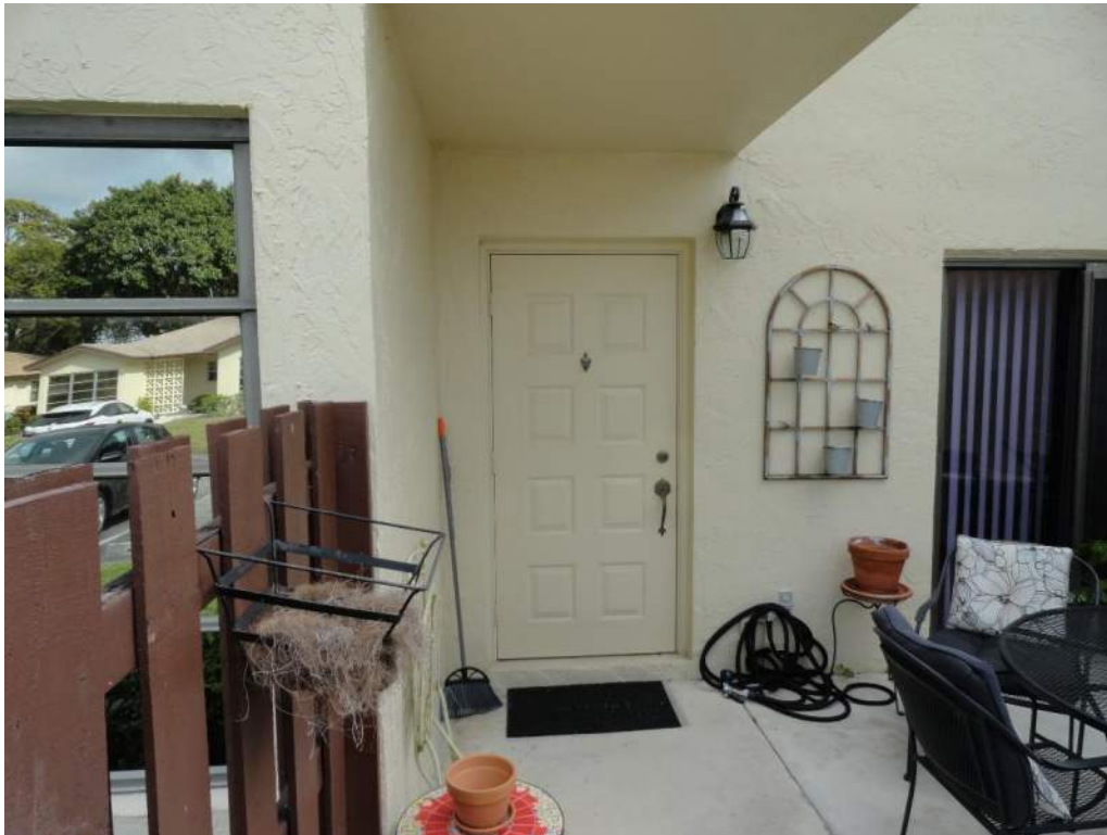
7. Opening Protection – Unprotected Unrated Unglazed Entry Door
