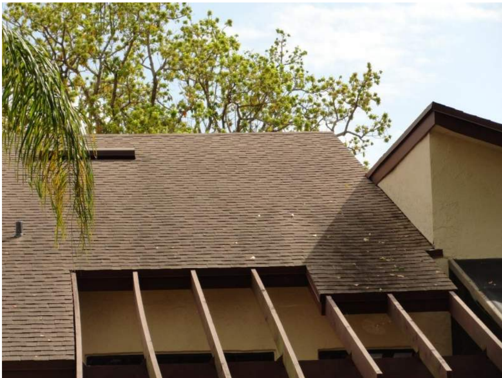
2. Roof Covering – Asphalt Shingles
