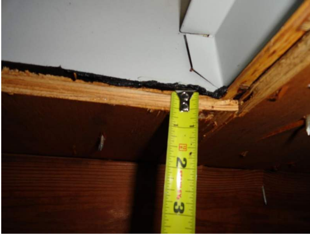
3. Roof Deck Attachment – 5/8" Plywood
